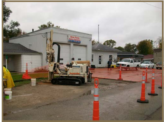
Soil boring installation
