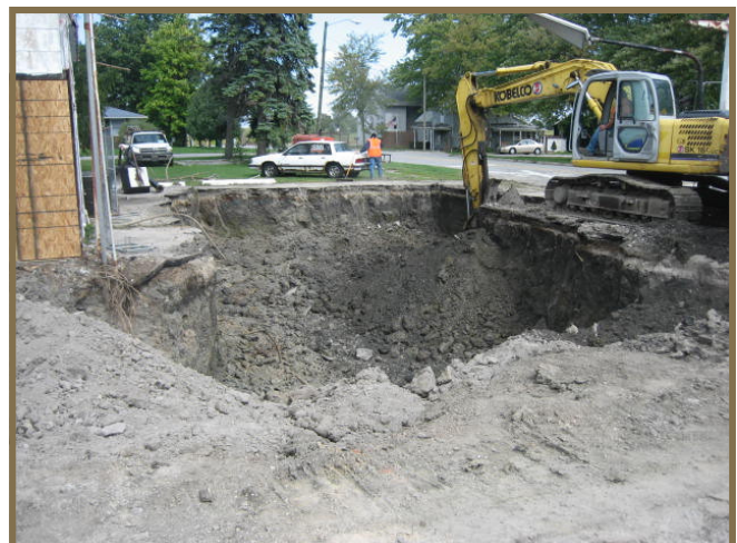
Over-excavation of contaminated soil
