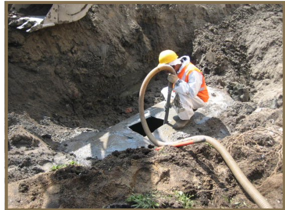
Removal of contents of 3,000-gallon gasoline tank
