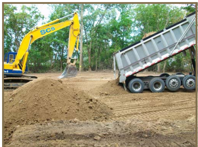
Bringing in backfill after UST removal.
