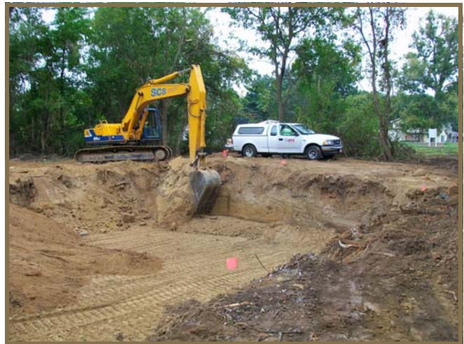
Excavation area after UST removal.
