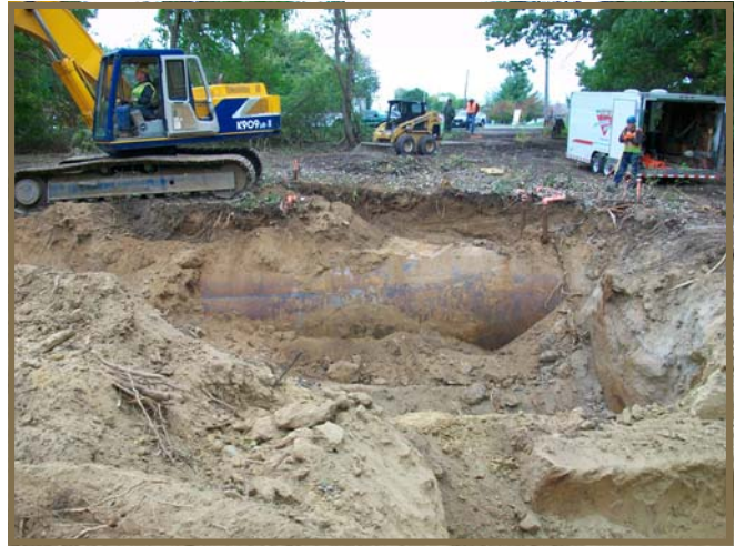
Initial uncovering of USTs.
