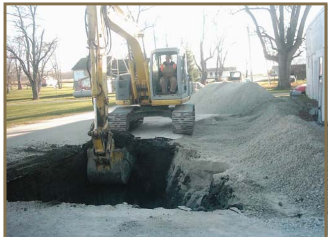
Over-excavation of contaminated soil
