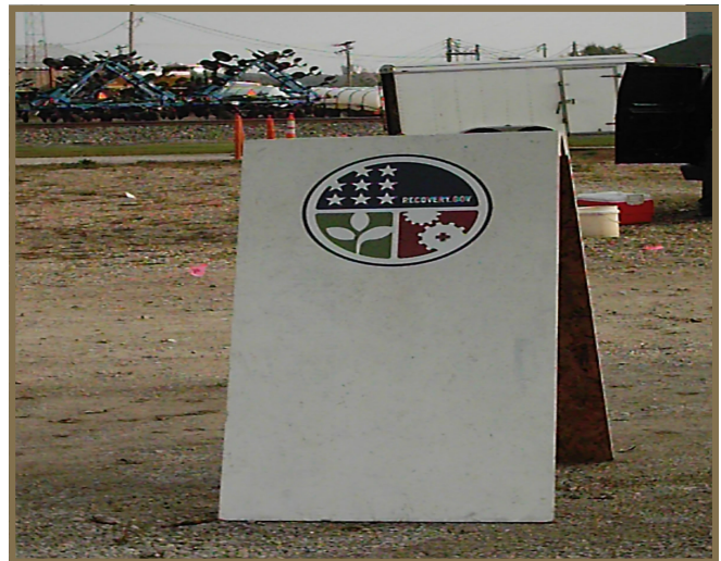
ARRA sign on site
