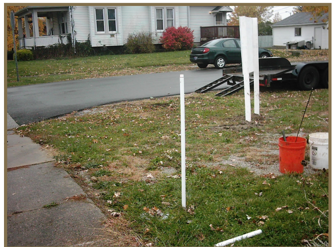
Temporary monitoring well
