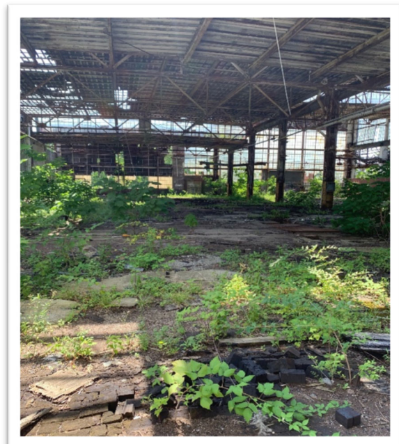
Roof and Ceiling of Machine Shop
