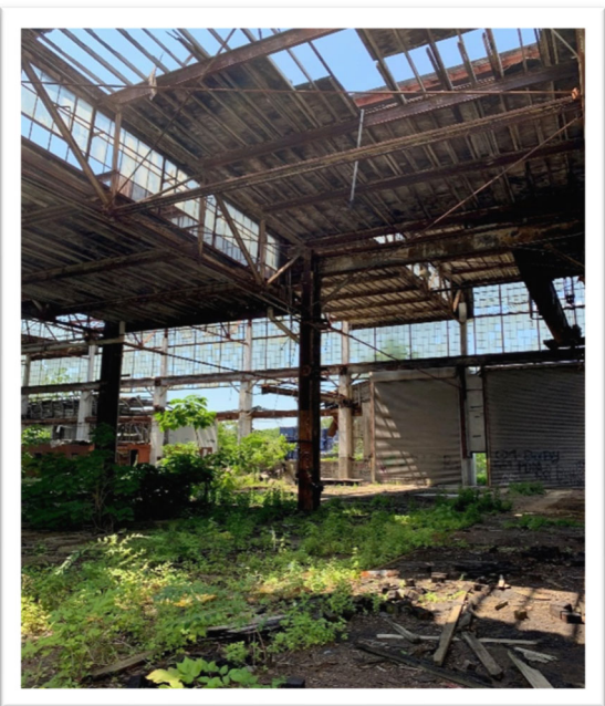
Roof and Ceiling of Coach Building
