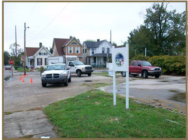
ARRA sign posted at the site; soil boring installation underway.
