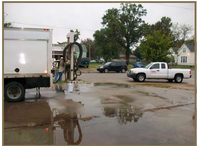
Soil boring installation.
