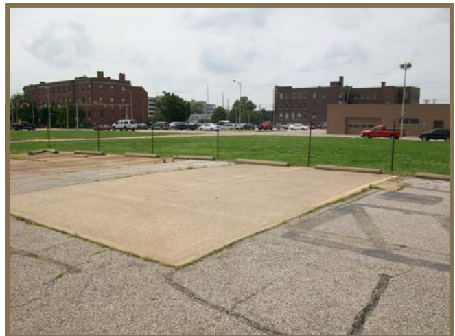
Former UST pit and excavation area.
