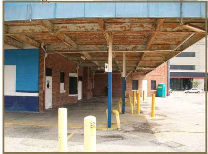
Former dispenser and refueling area.
