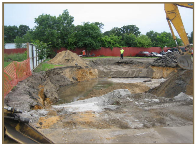
Over-excavation of contaminated soil
