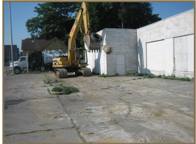
Breaking concrete above underground storage tank basin
