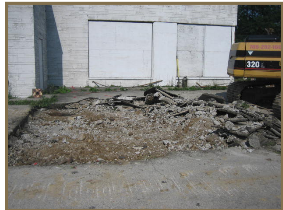
Excavation of contaminated soils
