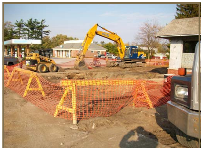
Over-excavation of contaminated soil once USTs were removed.
