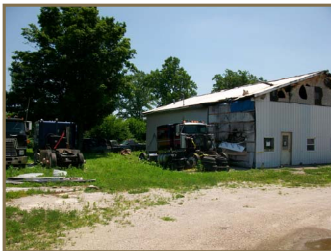
Site before remediation.
