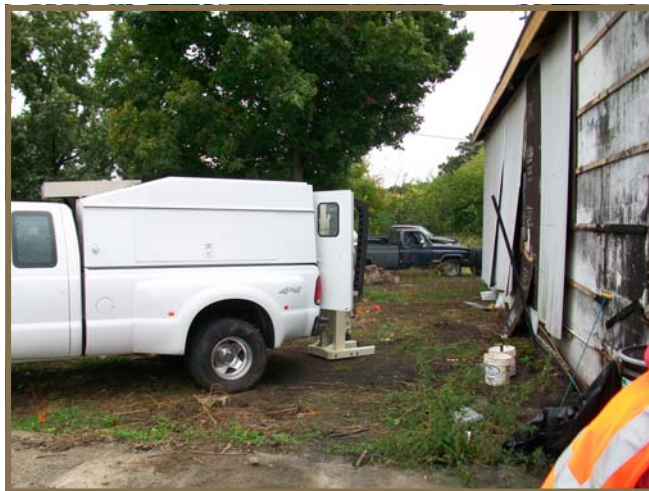
Soil boring installation
