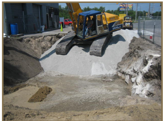
Backfilling of over-excitation
