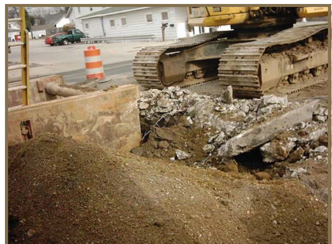
Soils at northern boundary of the site
