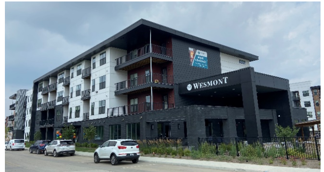
Former IPS Building & Grounds Project becomes The Wesmont in Indianapolis
