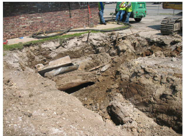
UST in the ground prior to removal
