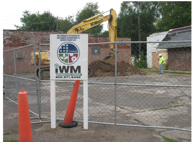
Site overview during UST removal
