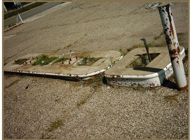
Former pump island
