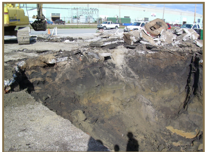
Over-excavation of contaminated soil
