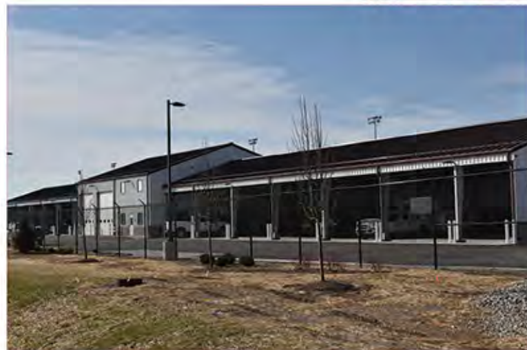
Left: Indiana Grand's brand new Track Maintenance building was erected as a part of Centaur Gaming's 2017 capital investment program. Right: The Winner's Circle in Downtown Indianapolis installed a brand new building facade giving the location a refreshed street presence.
