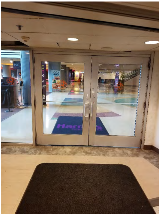
1 st floor entrance from parking garage
