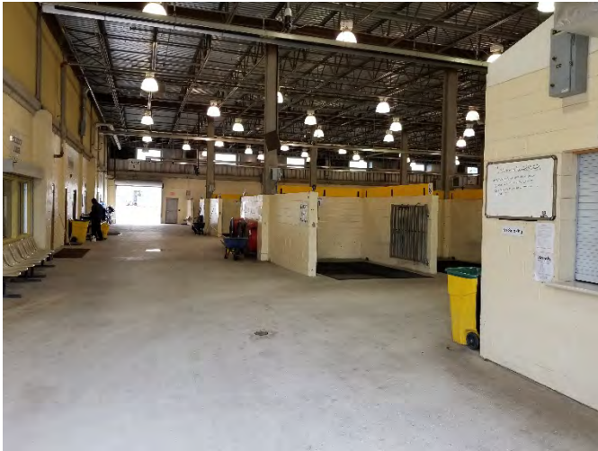
Ship-in/detention barn entrance
