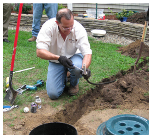
Figure 2: Bringing air line to riser.
