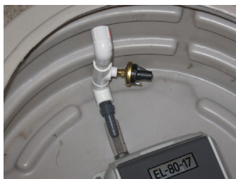
Figure A2: Air pump installed in protective basin.
