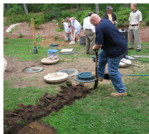
Figure 1: Trenching to riser.
