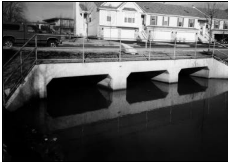
Exhibit 901a: Permanent Road Culvert (Source: CBBEL Files)
