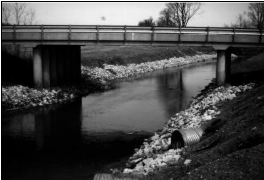
Exhibit 902a: A typical bridge (Source: NRCS Files)
