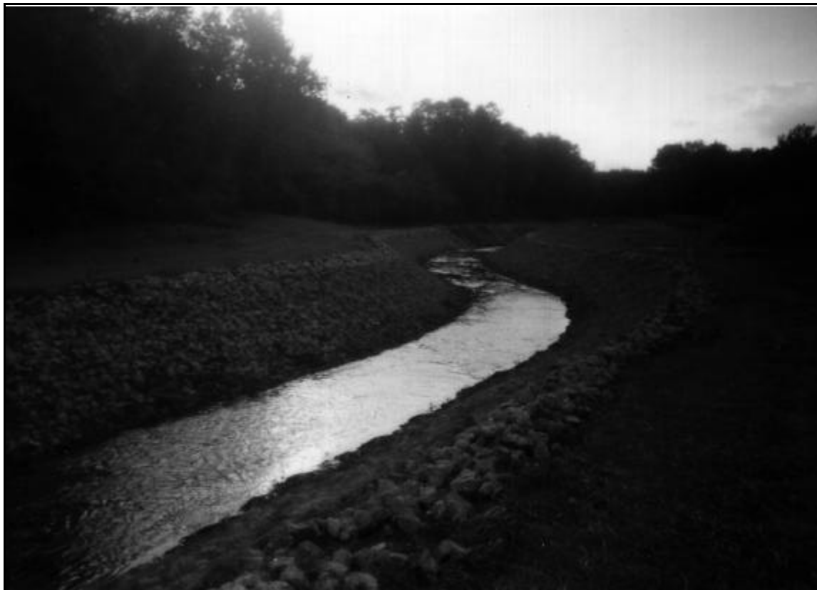
Exhibit 704a: Channel Transition (Source: Noble County Surveyor's Office Files)
