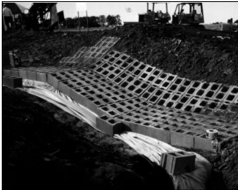
Exhibit 705c: Concrete Block Chute (Source: CBBEL Files)
