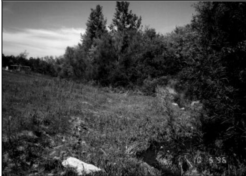
Exhibit 603a: Overbank excavation on one side of channel increases the flood carrying capacity of the stream (Source: CBBEL Files)
