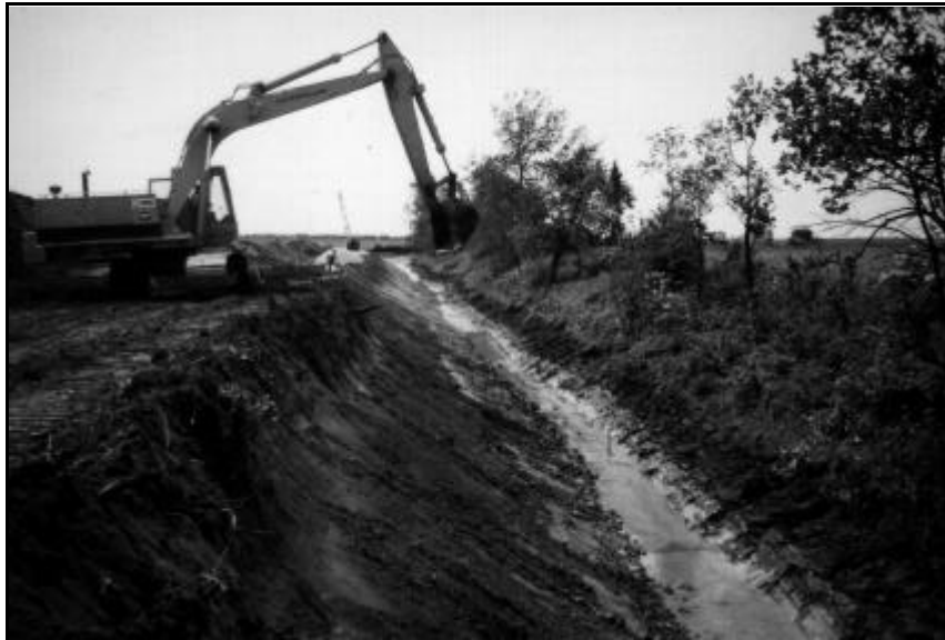
Exhibit 602a: Channel Excavation/Dredging (Source: NRCS Files)
