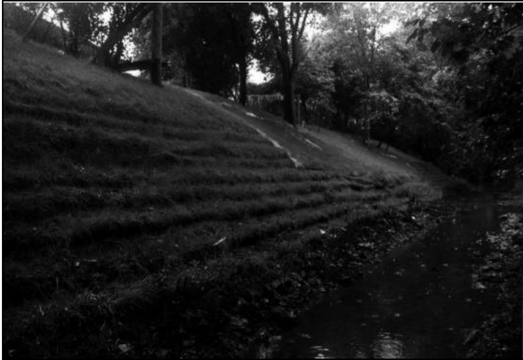
Exhibit 506a: Vegetative Geogrid (Source: Biotechnical Erosion Control Limited)
