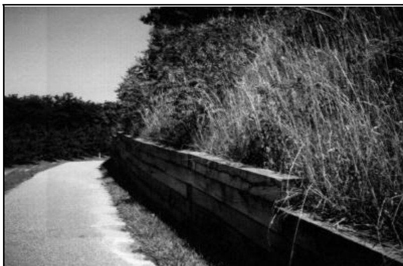
Exhibit 513a: Timber Retaining Wall (Source: NRCS Engineering Field Handbook)
