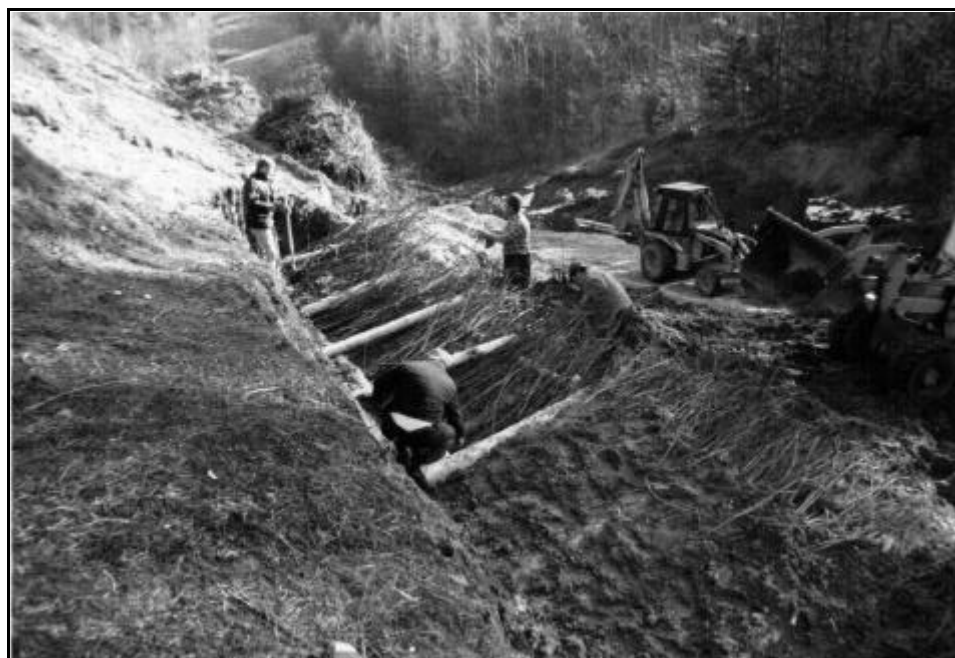
Exhibit 507a: Live Cribwalls (Source: NRCS Engineering Field Handbook)
