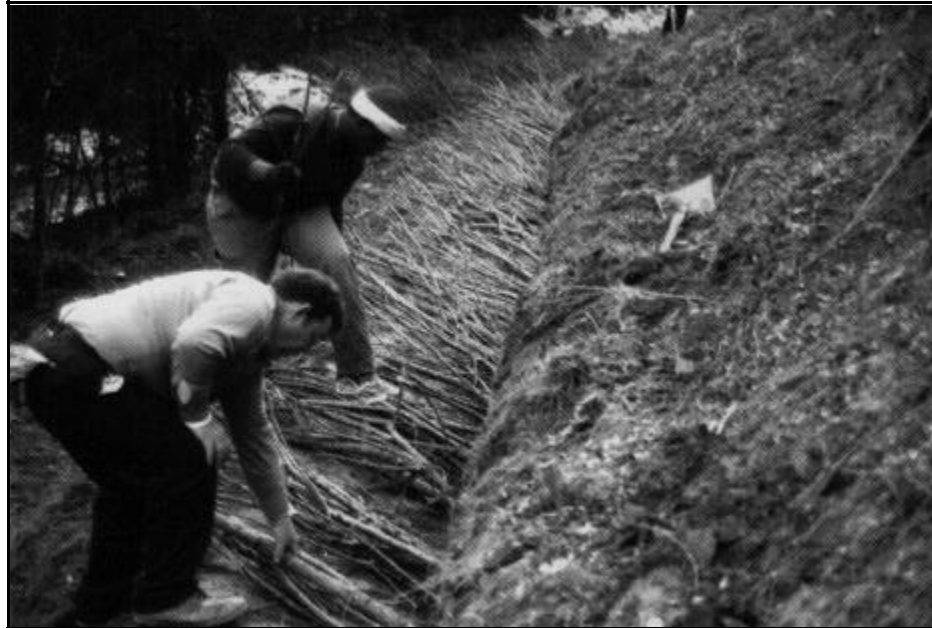
Exhibit 503a: Branch Packings (Source: NRCS Engineering Field Handbook)
