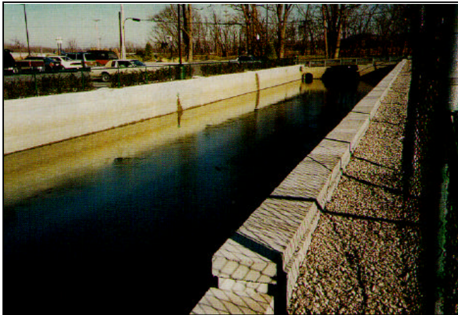
Exhibit 511a: Concrete Retaining Wall (Source: Land and Water Magazine)
