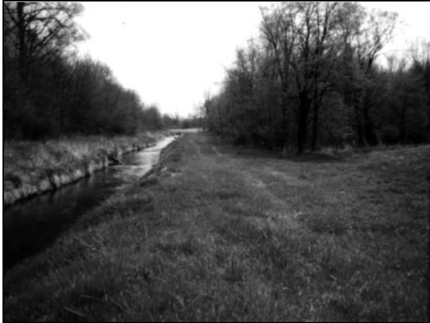
Exhibit 1303a: Permanent Maintenance Access (Source: Allen County Surveyor's Office Files)
