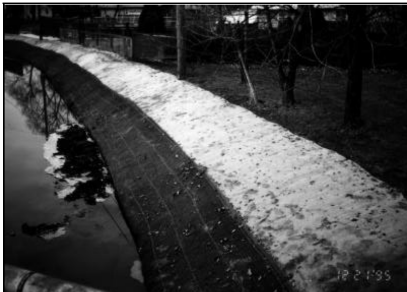
Exhibit 1104a: Erosion Control Blanket (Source: CBBEL Files)
