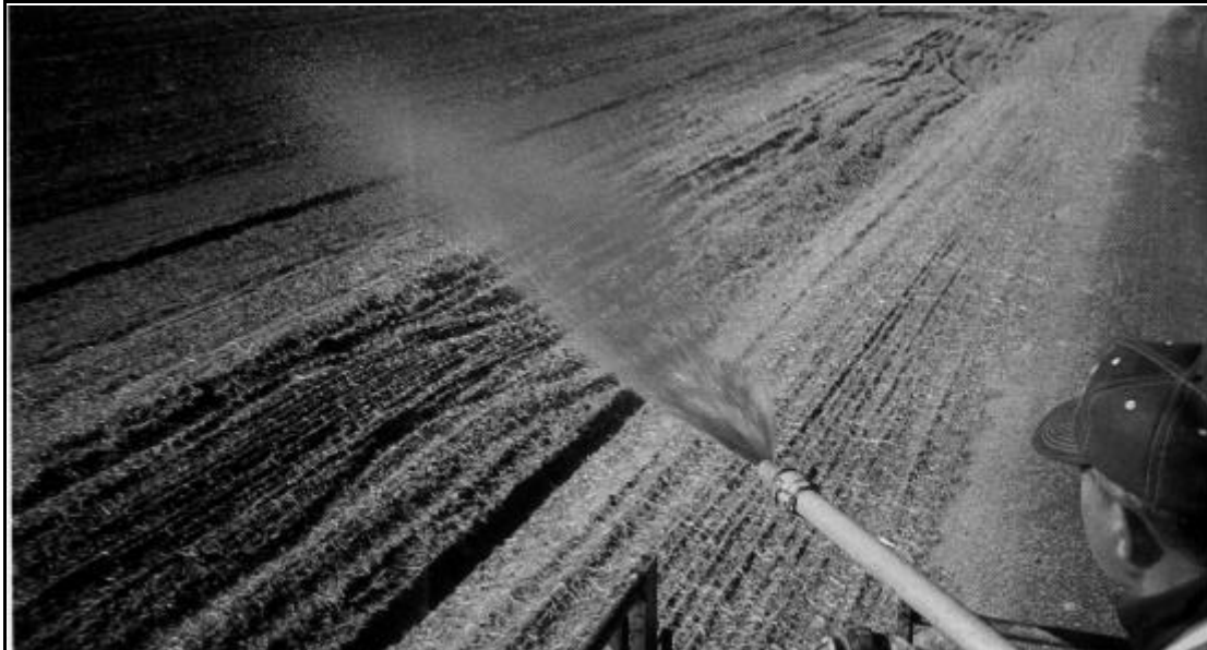
Exhibit 1101a: Mulching (Source: North Carolina Erosion Control Manual)
