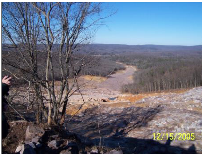
Figure 1-3 Photo showing downstream environmental damage after the Taum Sauk Dam failure in December, 2005, near Lesterville, Missouri. No people were injured. The dam failed when pump/reservoir level control equipment failed to shut off the reservoir filling pumps.
