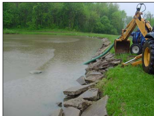
Figure 3-3 Backhoe being used to place an emergency pump in the reservoir.
