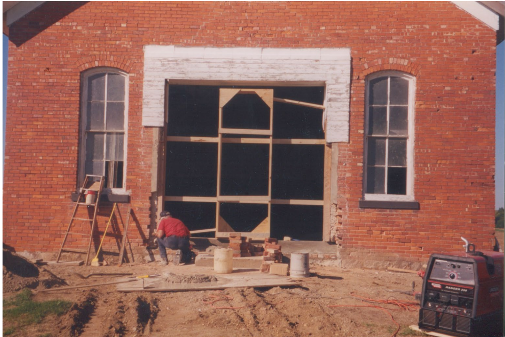
Clay Township District 8 Schoolhouse during rehabilitation, c. 2003 Photo from collection of Ransbottom family
