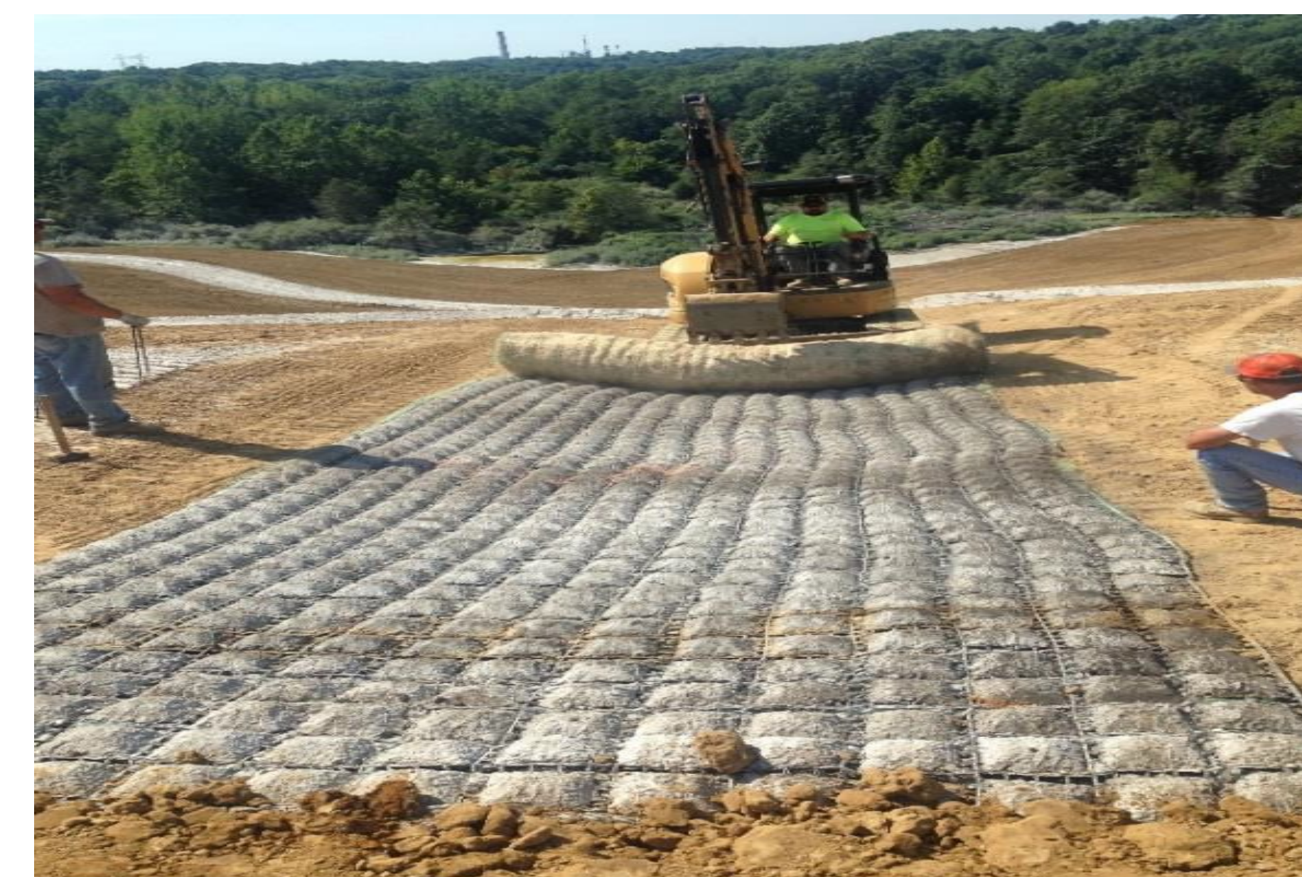
Below: Installation of Flexamat® ditch armoring, north refuse
