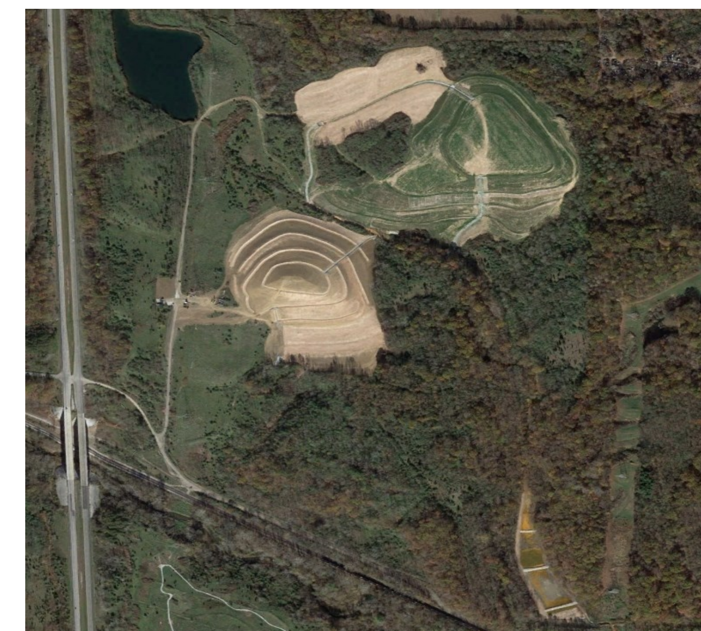
Post Construction of the project showing both of the buried gob piles and the wetland and settling pond.
