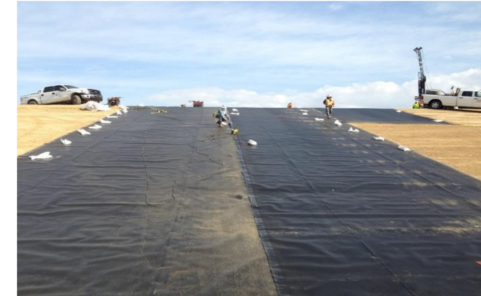
Welding of installed geomembrane sections, south refuse pile.
