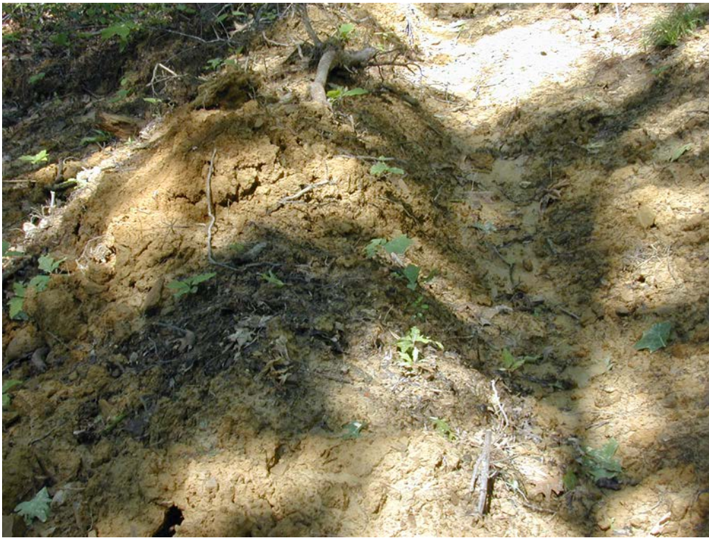
An effective water bar conveying runoff from a skid trail and diverting the flow onto the forest duff layer, where it will infiltrate, remove sediment and return to groundwater.
