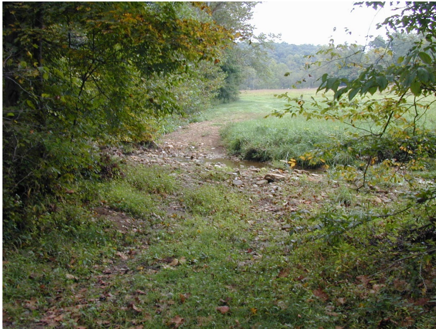
An access-road ford across a small stream with low and stable banks.
