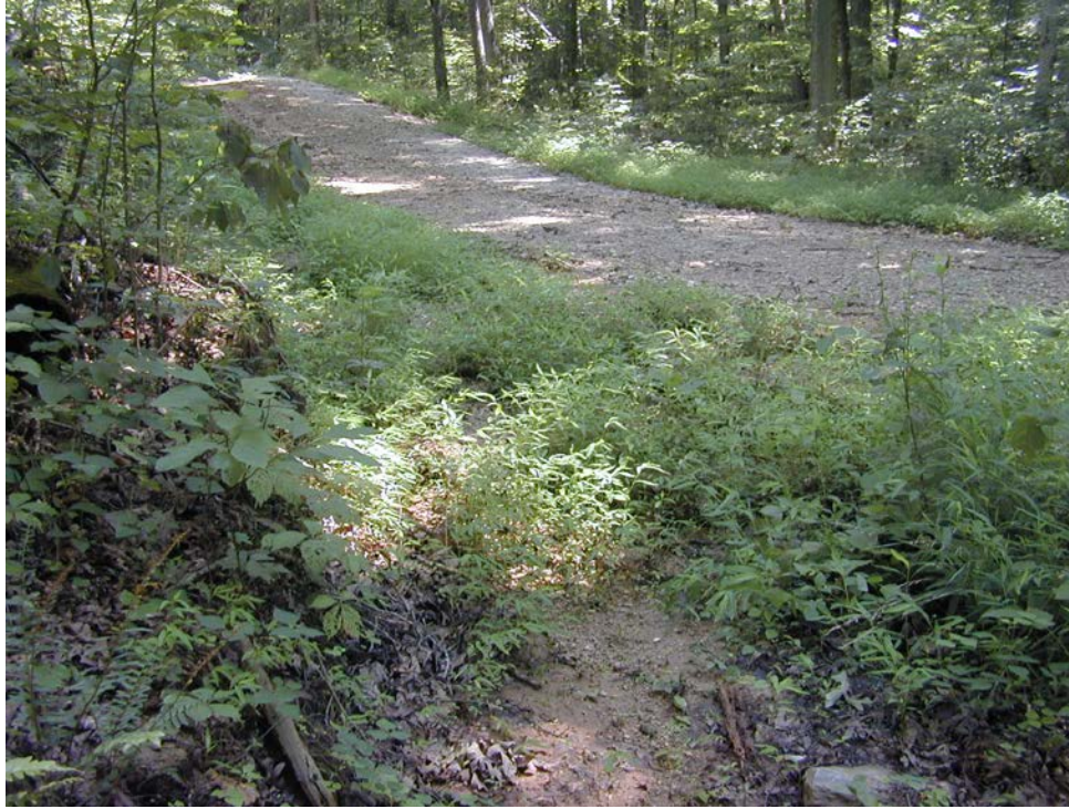
Effective cutout on a permanent access road.
