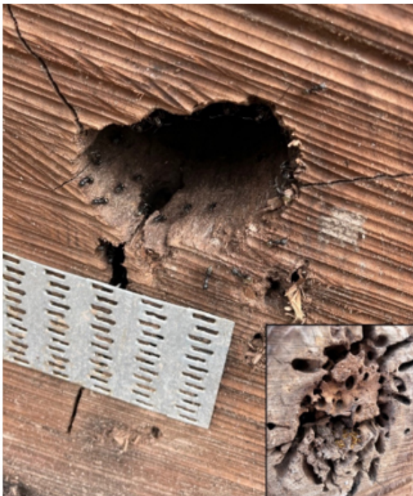
Photo 10 – Recent carpenter ant ( Camponotus spp.) activity in a Black Walnut ( Juglans nigra ) log. Carpenter ants can make some elaborate and structured tunnel systems in decayed areas of logs as seen in the inset photo. These are more common pests of logs than termites, which they can be confused for (see next image)
