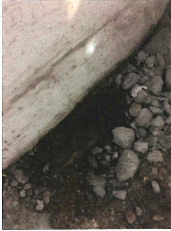
Photo 1. Footing Along East Nonbearing Wall
