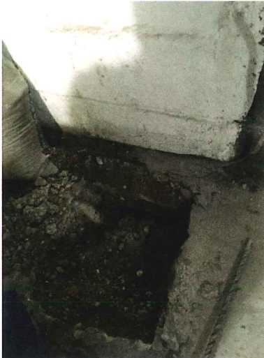
Photo 7. North Bearing Wall
