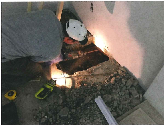
Photo 3. Drilling Into Footing
