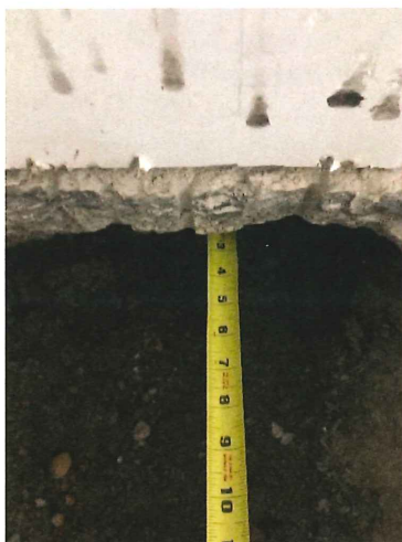
Photo 5. South Bearing Wall (Footing setback from Non-loadbearing framing)
