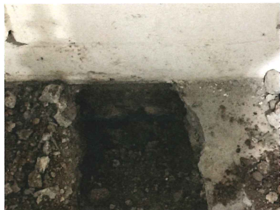
Photo 6. Middle Bearing Wall Footing
