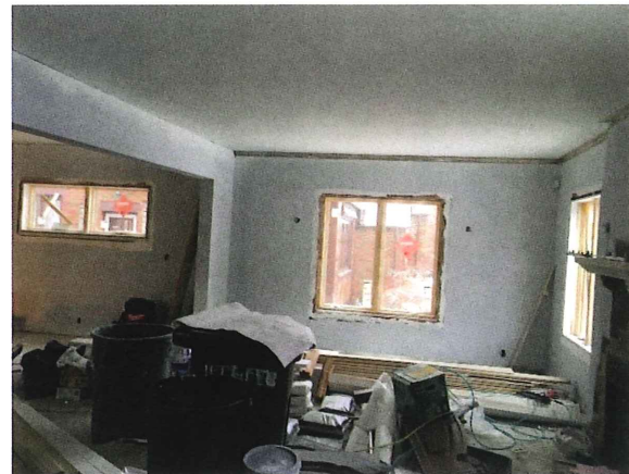
Photo 10. First Floor Living Room
