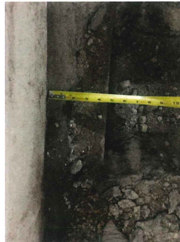
Photo 8. North Bearing Wall Toe Measurement
