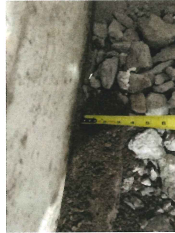
Photo 2. Toe Measurement Along East Nonbearing Wall
