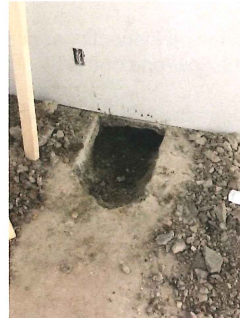
Photo 4. South Bearing Wall Footing
