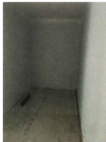
Photo 12. Second Floor Attic Entry Hallway
