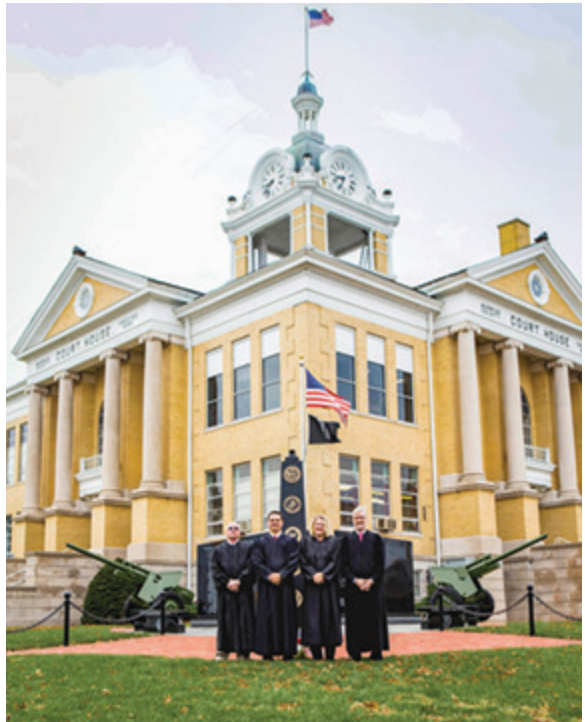
Judicial officers from Warrick County stand outside the county courthouse in Boonville, which was completed in 1904.
