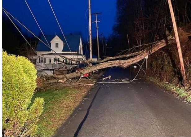
Figure 26: Damage from High Winds during a Thunderstorm
