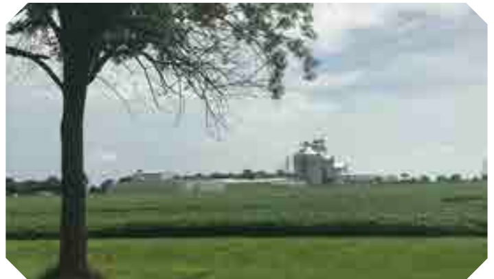
Image Source: HWC Engineering
