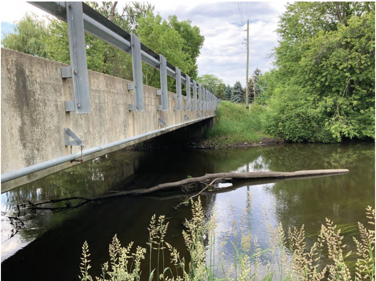
16. Looking south from Elkhart River right bank
