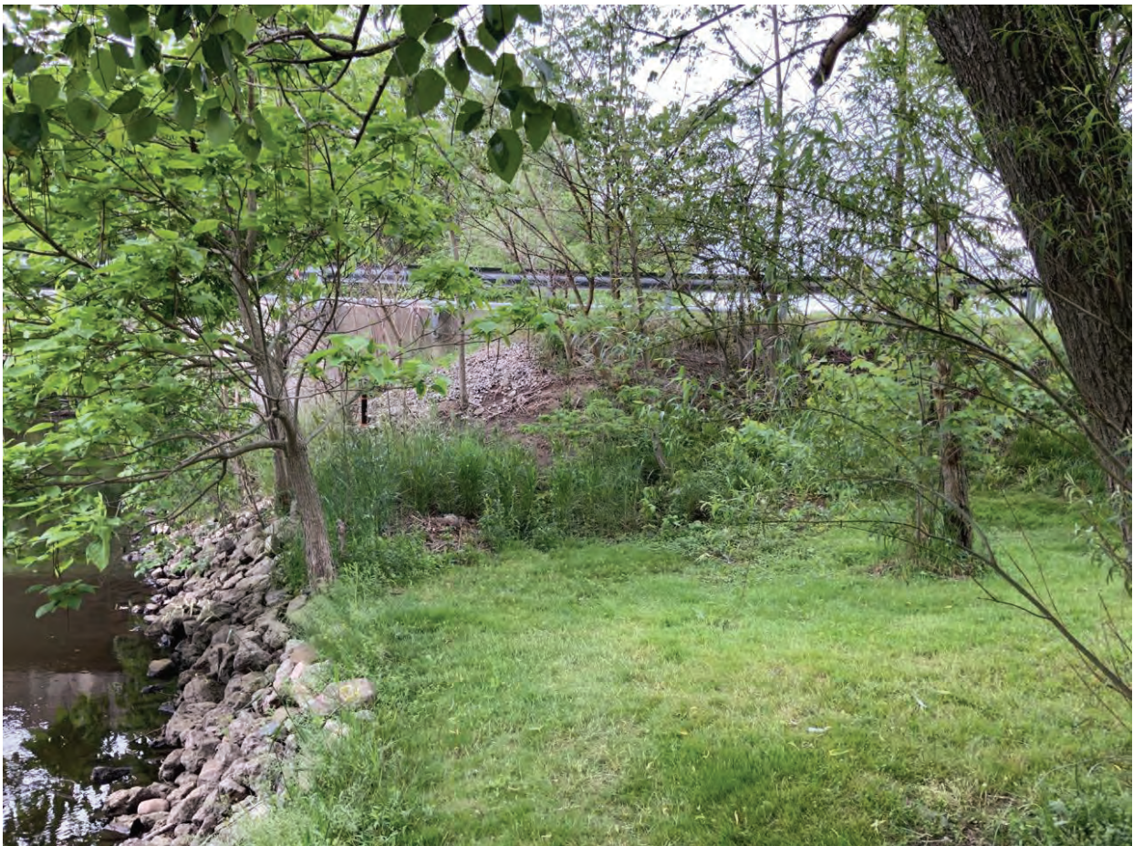
20. Looking west toward structure along Elkhart River right bank
