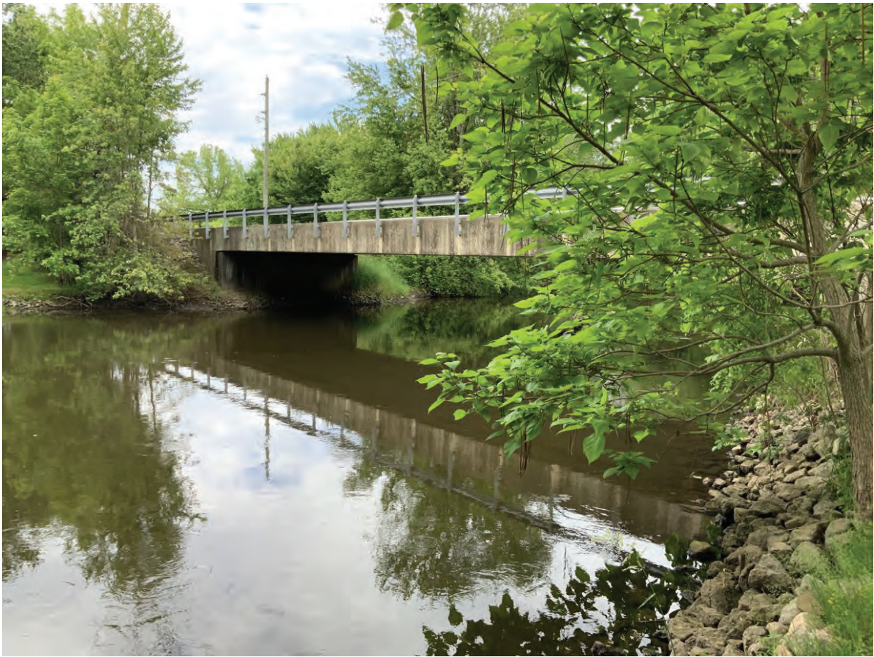
19. Looking southwest at structure from Elkhart River right bank
