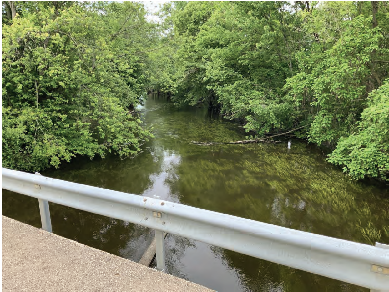
13. Looking southwest from structure along Elkhart River downstream
