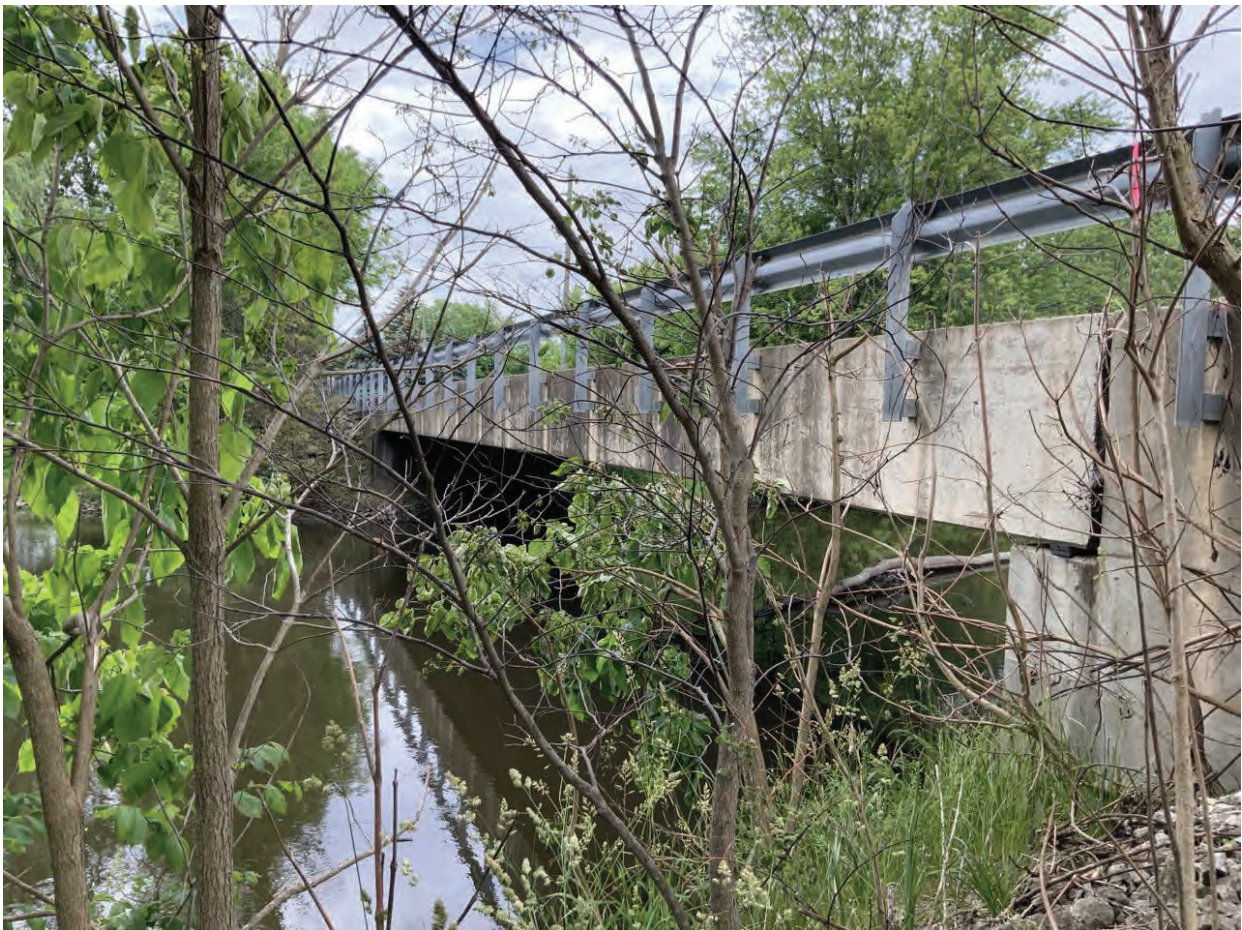
18. Looking south at structure from embankment
