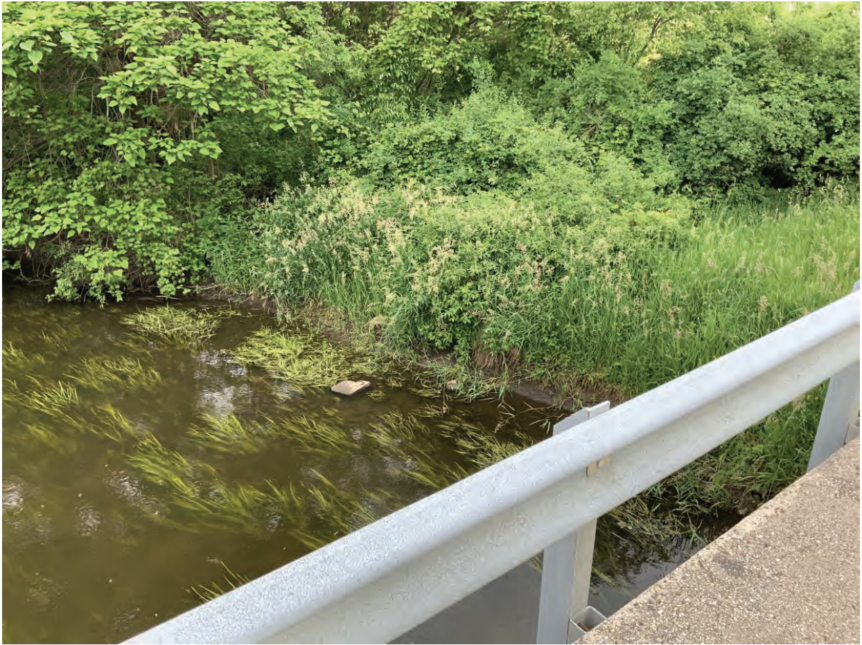
15. Looking northwest from structure at Elkhart River right bank
