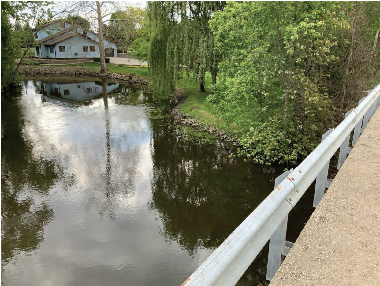
11. Looking southeast from structure at Elkhart River left bank
