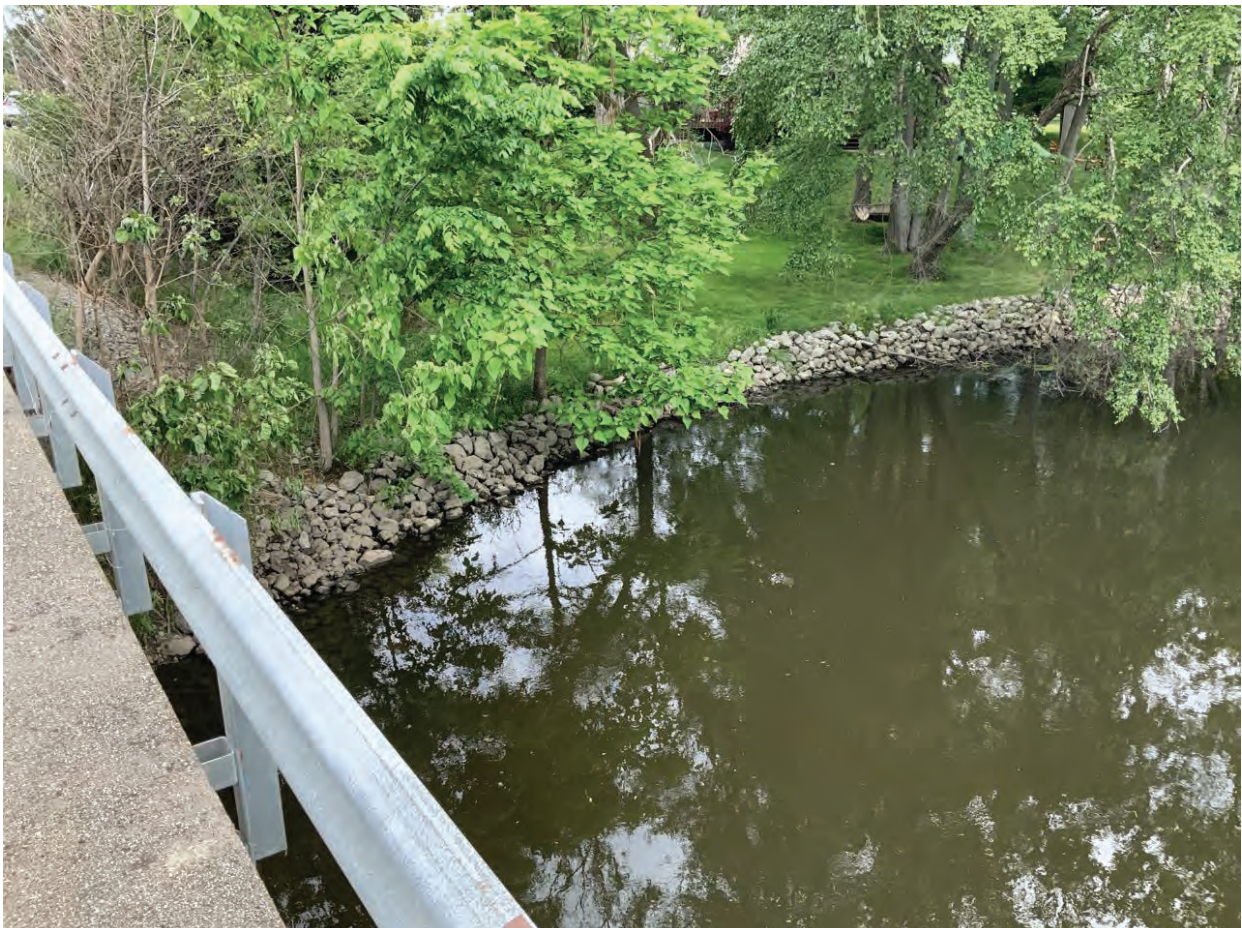
10. Looking northeast from structure at Elkhart River right bank
