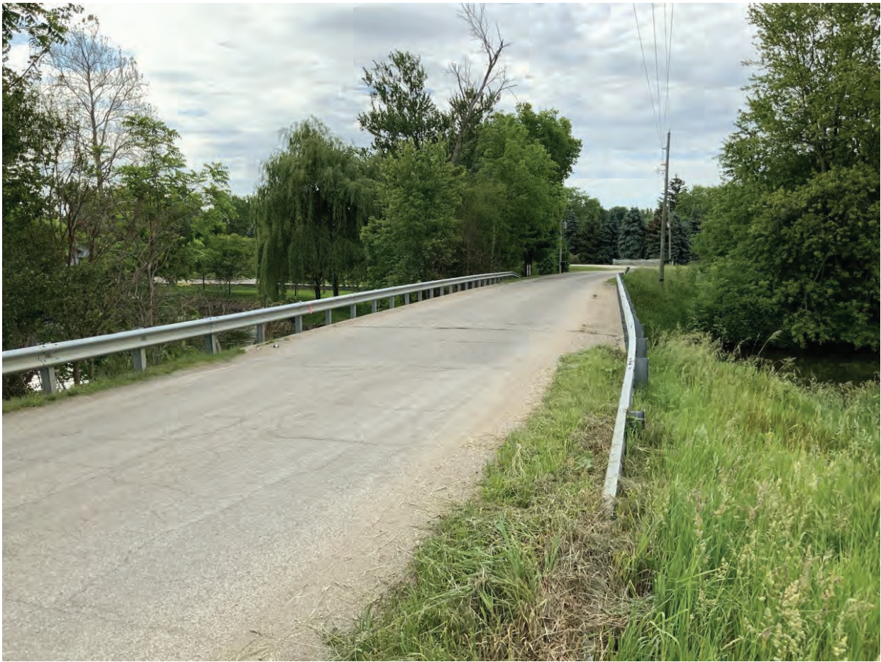
21. Looking south along Rochester Road at structure
