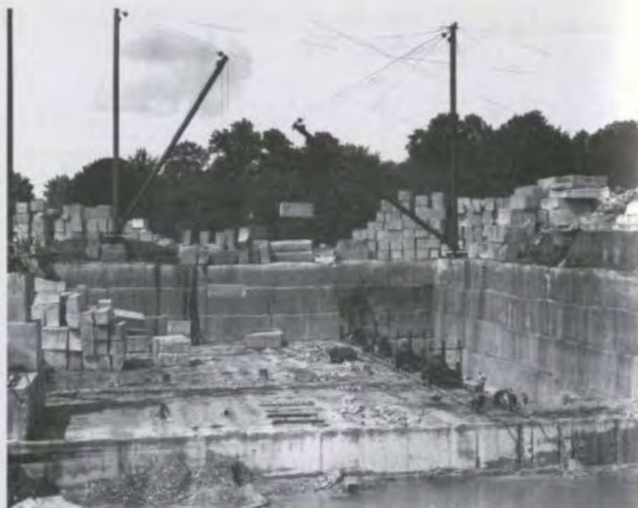
Quarry with steam-powered channeling machines. Photo by Charles Gilbert Shaw. Courtesy, Monroe County Historical Museum.
