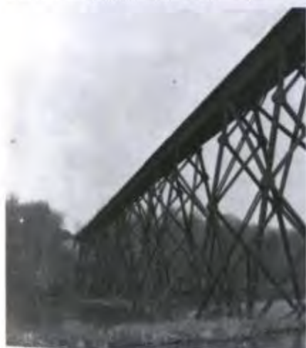
Railroad Trestle (01017) When the Illinois Central Railroad brought its tracks through Monroe County after the turn of the century, it had to build sizable trestles in Benton Township, to attain a relatively level grade. Like the trestle in Victor, the wooden trestle near Lake Lemon has been rebuilt since its original construction, but the tall steel trestle that spans Shuffle Creek is the original version.
