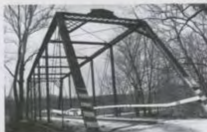
Bridge No. 625 (30002) This Pratt Through Truss bridge was fabricated by the Wrought Iron Bridge Company of Ohio and erected over Salt Creek around 1895. It is the finest and most picturesque of the few remaining metal bridges in Monroe County.
