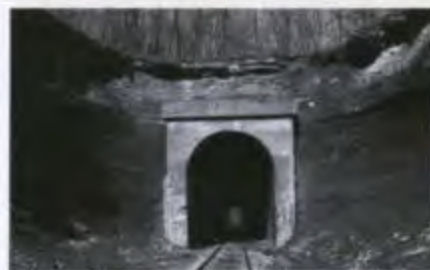
Railroad Tunnel (01021) This tunnel, built in 1918 to accommodate the second major railroad line through Monroe County, the Illinois Central, runs under Tunnel Road. It is 584 feet long.
