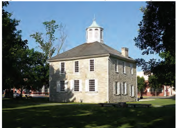
Figure 3.9: Historic State Capitol Building
