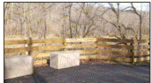
Railing at viewing area is too high.
