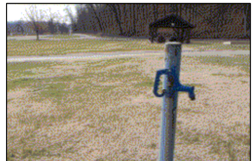
Noe's Rest Park water source is too high and not on an accessible route.
