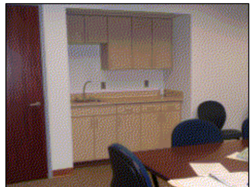
Countertop is too high and there is no knee space to use sink.
