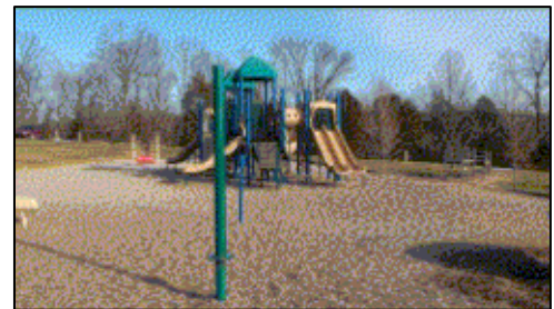
Playground has no accessible route provided and surfacing is not compliant.
