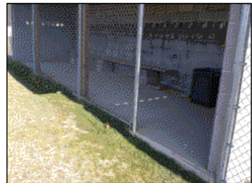
Dugout entrance is not accessible.
