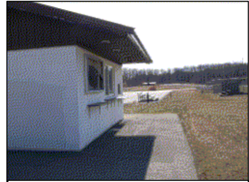
Protruding concessions counter at South Harrison Park.
