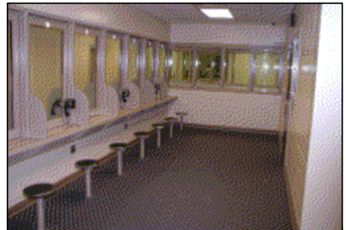
Prisoner visitation area lacks space for wheelchair to park.
