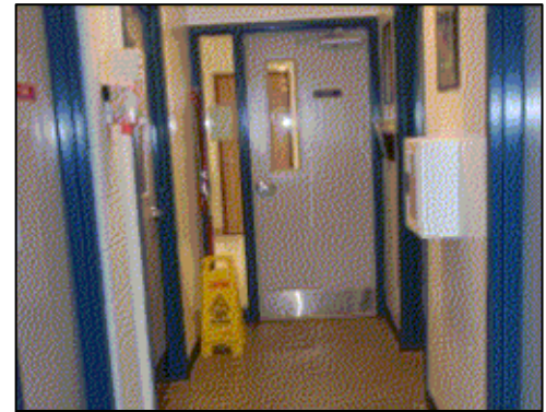
Defibrillator and ear plug container protrude at Animal Control hallway.
