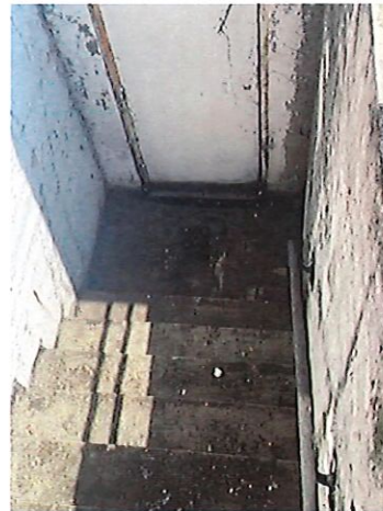
Eastern Stairwell & Cistern
