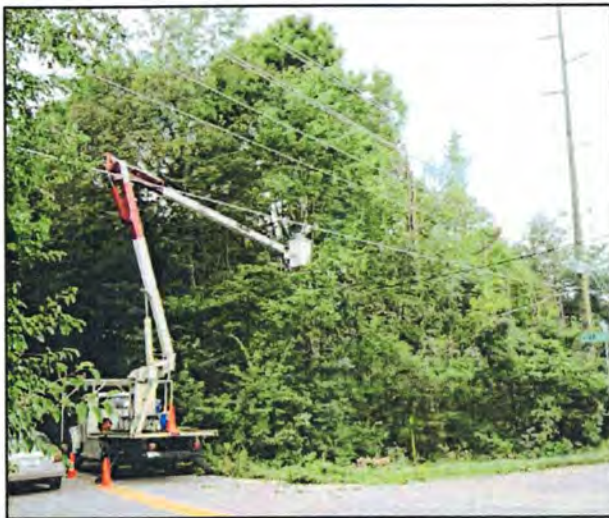
Utility arborists prune for safe clearance around distribution lines.
