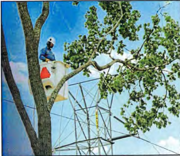
Utility arborists are trained specifically for working around utility lines.
