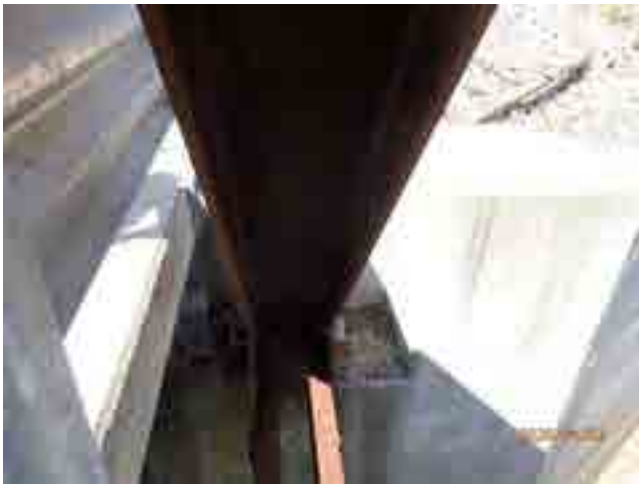
LOOKING AT NORTH TRUSS L0
