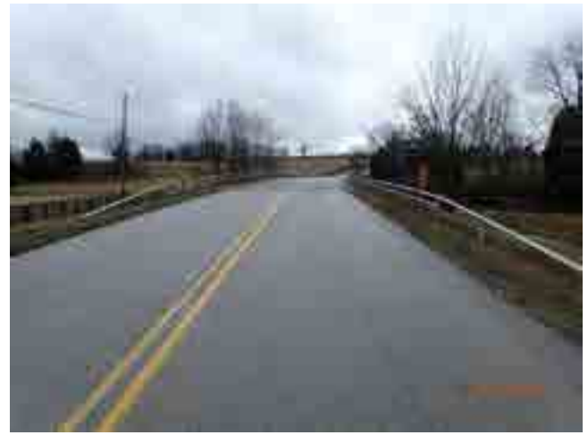
LOOKING SOUTH FROM ROAD
