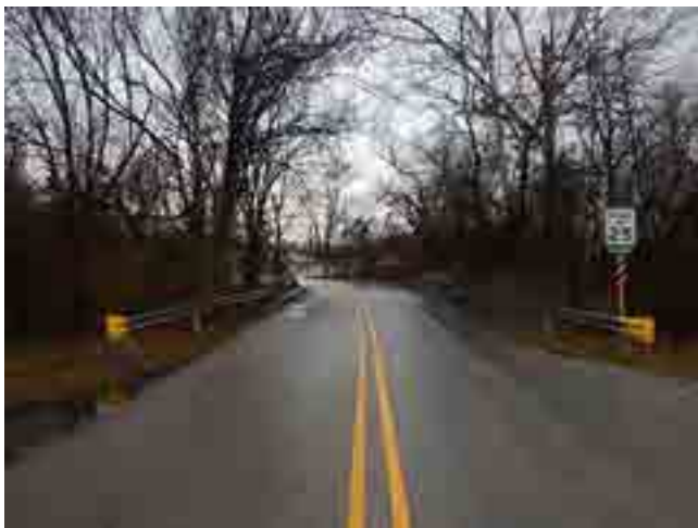
LOOKING NORTH FROM ROAD
