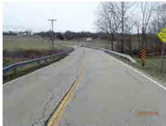
LOOKING WEST FROM ROAD
