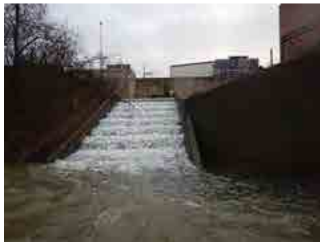
LOOKING EAST AT SEWAGE TREATMENT PLANT
