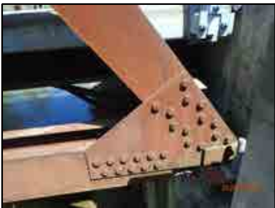
LOOKING AT SOUTH TRUSS L12
