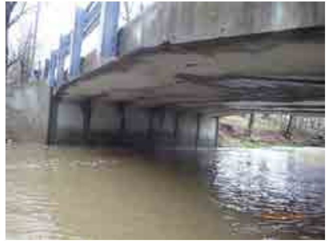
WEST ABUTMENT AND DOWNSTREAM COPING
