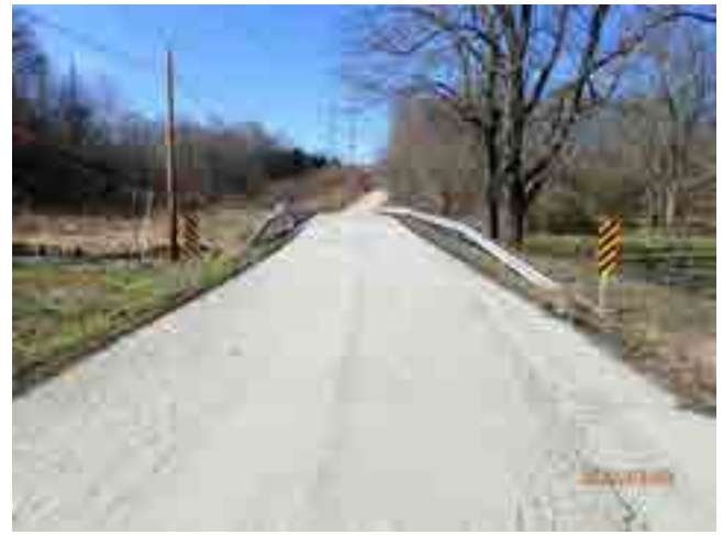
LOOKING WEST FROM ROAD
