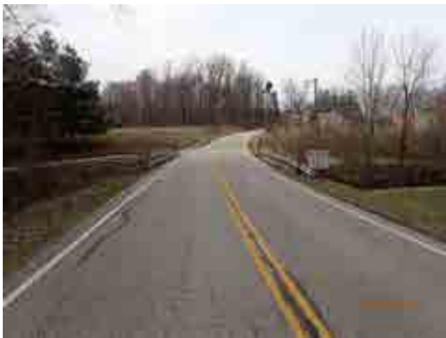
LOOKING NORTH FROM ROAD
