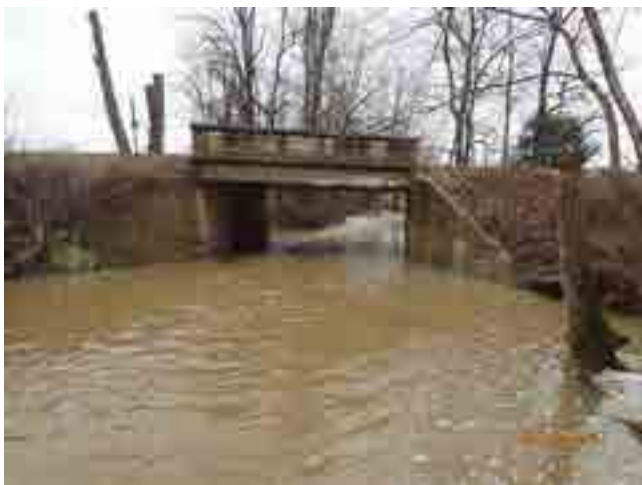
LOOKING EAST THROUGH CHANNEL
