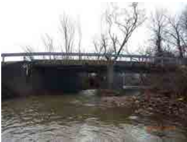
LOOKING SOUTH DOWNSTREAM
