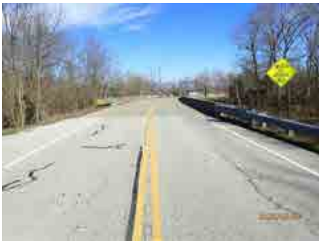
LOOKING NORTH FROM ROAD
