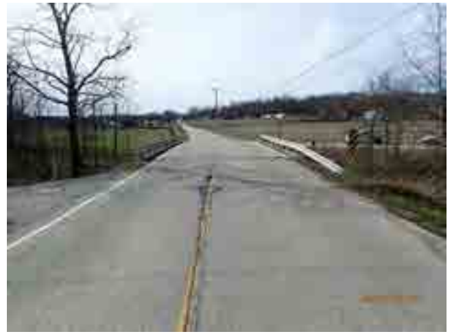
LOOKING WEST FROM ROAD
