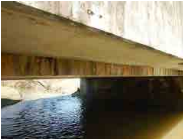
WEST EFFL. BTWN. THE OUTER E TWO BEAMS
