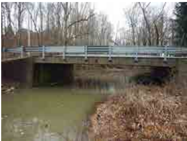
LOOKING SOUTH FROM CHANNEL
