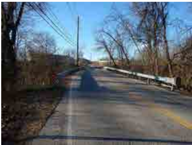
LOOKING NORTH FROM ROAD
