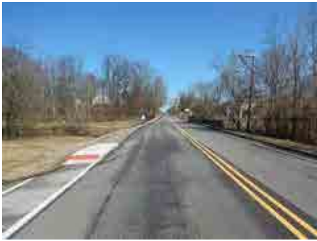
LOOKING NORTH FROM ROAD
