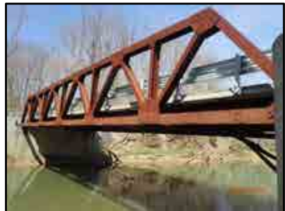
LOOKING NORTH FROM CHANNEL
