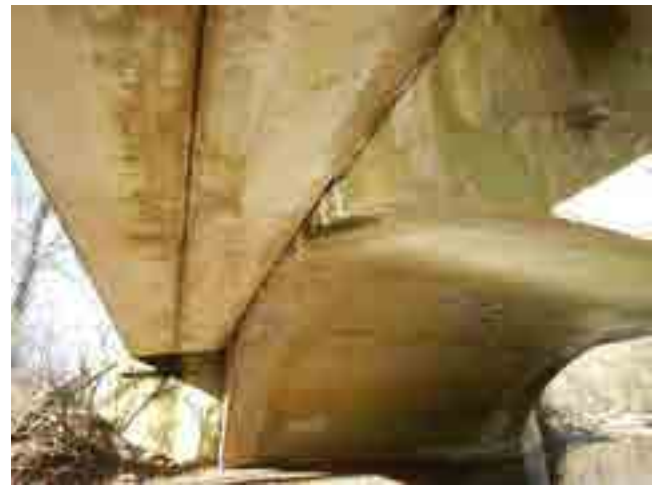
LOOKING SOUTH AT EAST ARCH COPING
