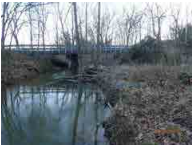
LOOKING SOUTH THROUGH CHANNEL
