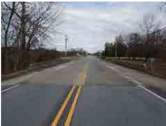
LOOKING NORTH FROM ROAD
