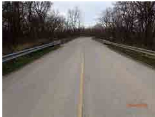
LOOKING WEST FROM ROAD
