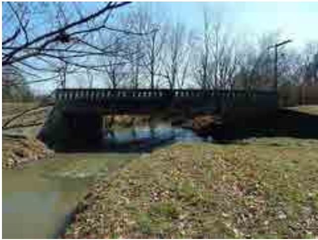
LOOKING EAST DOWNSTREAM
