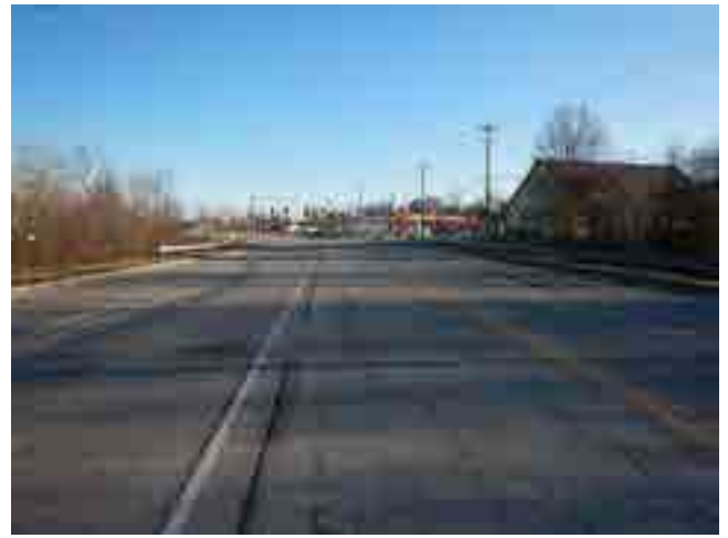
LOOKING NORTH FROM ROAD
