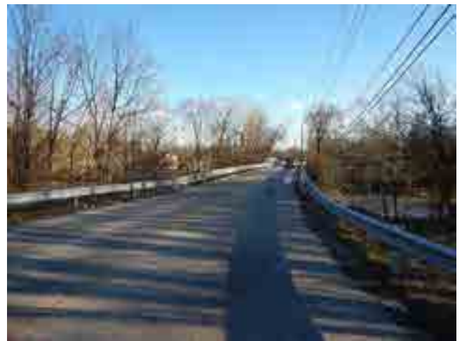
LOOKING SOUTH FROM ROAD
