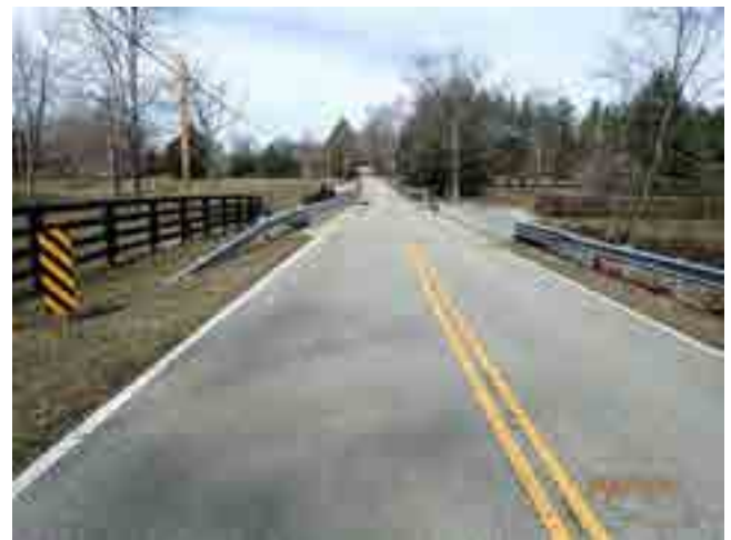
LOOKING NORTH FROM ROAD
