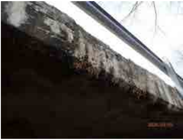
DOWNSTREAM COPING RAVELING
