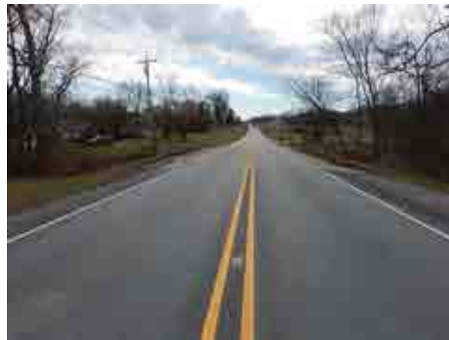
LOOKING SOUTH FROM ROAD
