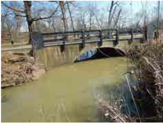
LOOKING NORTH DOWNSTREAM
