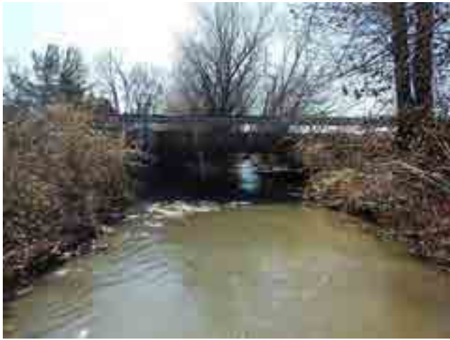
LOOKING SOUTH DOWNSTREAM
