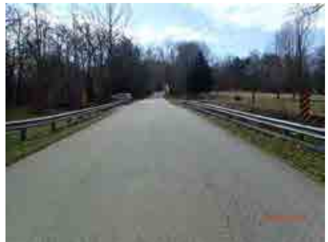
LOOKING SOUTH FROM ROAD
