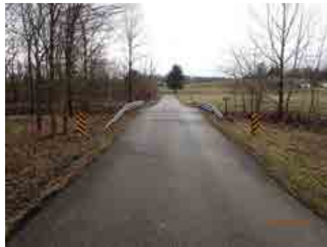
LOOKING WEST FROM ROAD
