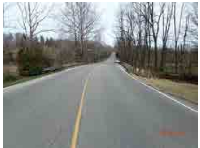
LOOKING NORTH FROM ROAD
