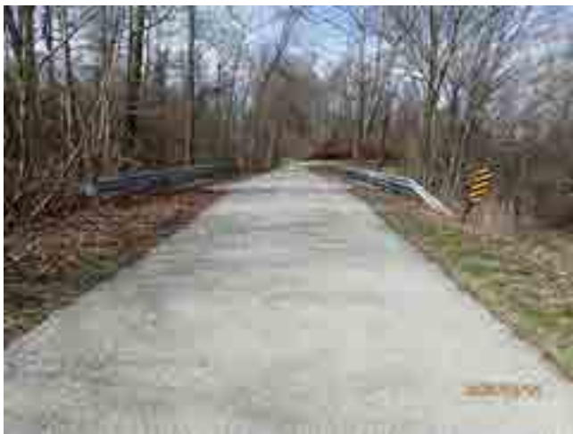
LOOKING NW FROM ROAD
