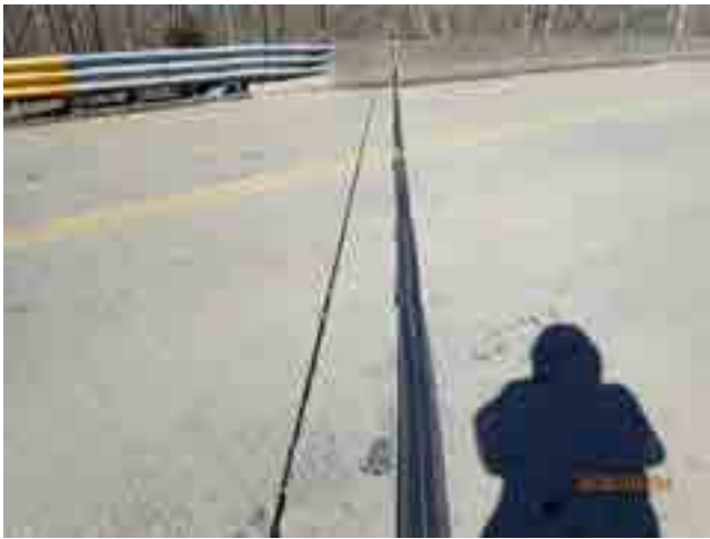
SOUTH EXPANSION JOINT
