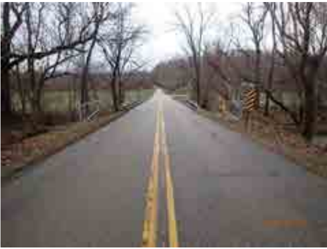
LOOKING WEST FROM ROAD
