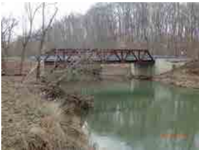
LOOKING SOUTH THROUGH CHANNEL
