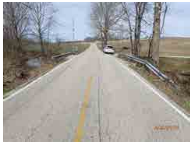
LOOKING NORTH FROM ROAD
