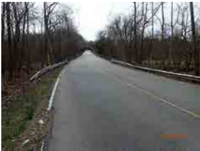
LOOKING SOUTH FROM ROAD
