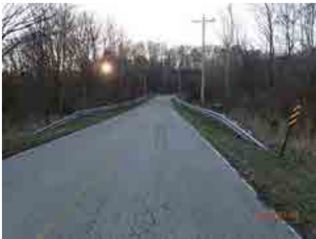
LOOKING WEST FROM ROAD
