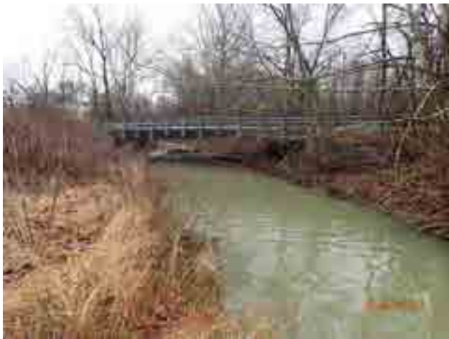
LOOKING SOUTH FROM CHANNEL
