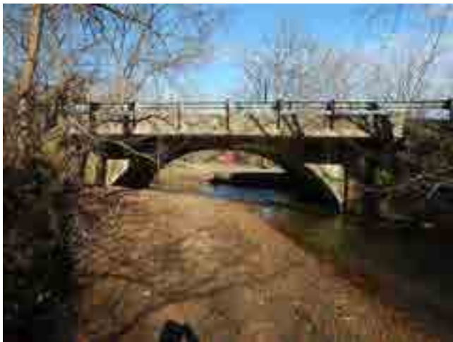
LOOKING WEST UPSTREAM
