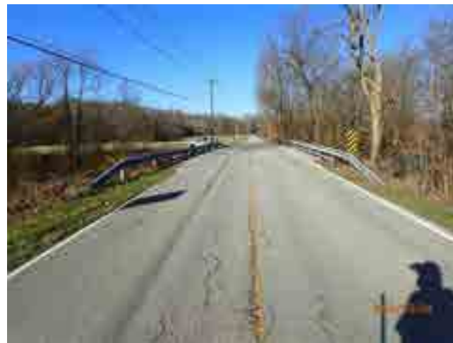
LOOKING WEST FROM ROAD
