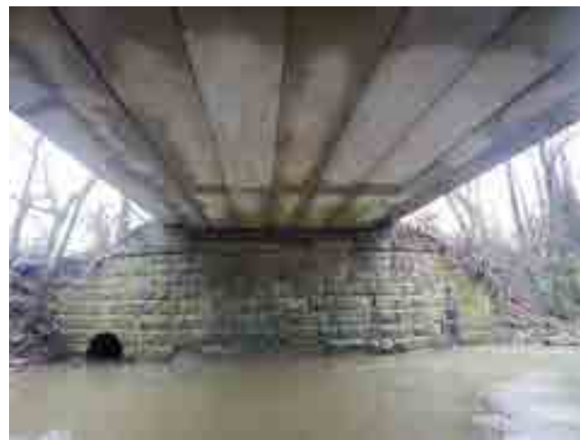
LOOKING SOUTH AT SOUTH ABUTMENT
