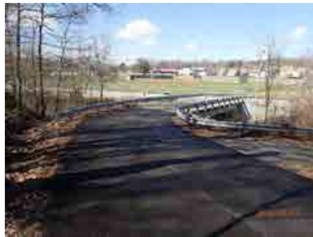
LOOKING NORTH FROM ROAD
