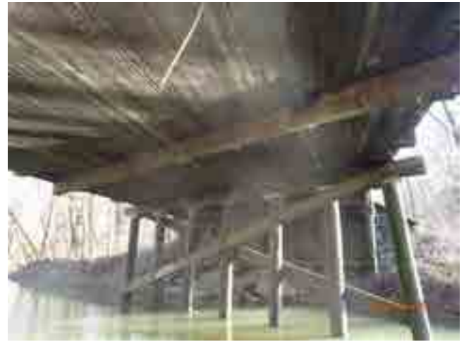
LOOKING SOUTH AT SOUTH PIER
