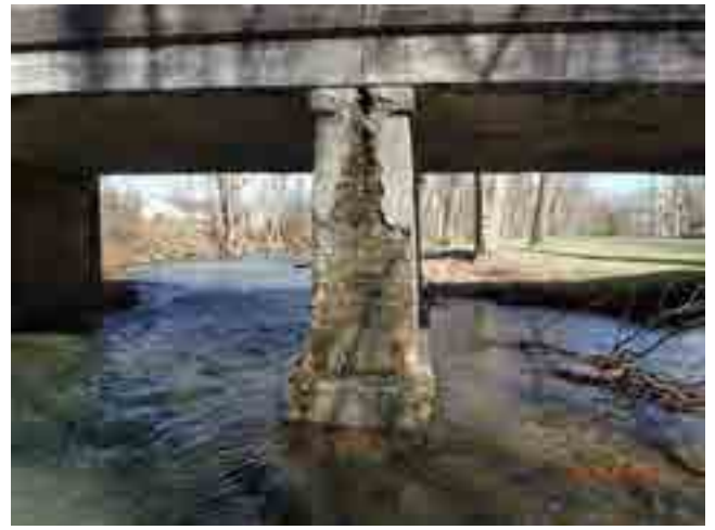
DOWNSTREAM PIER NOSE
