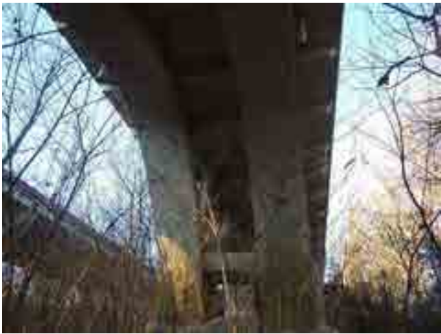
LOOKING WEST AT APPROACH SPANS
