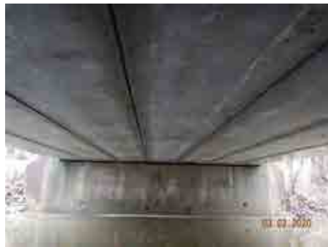
LOOKING EAST AT SUPERSTRUCTURE AND EAST
