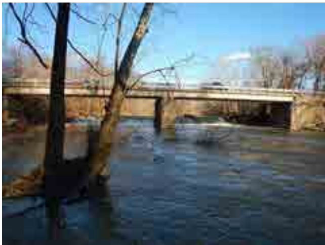
LOOKING EAST UPSTREAM
