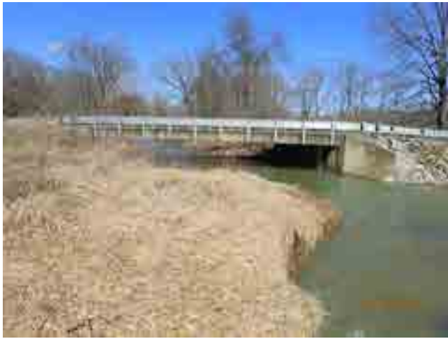
LOOKING NORTH FROM CHANNEL
