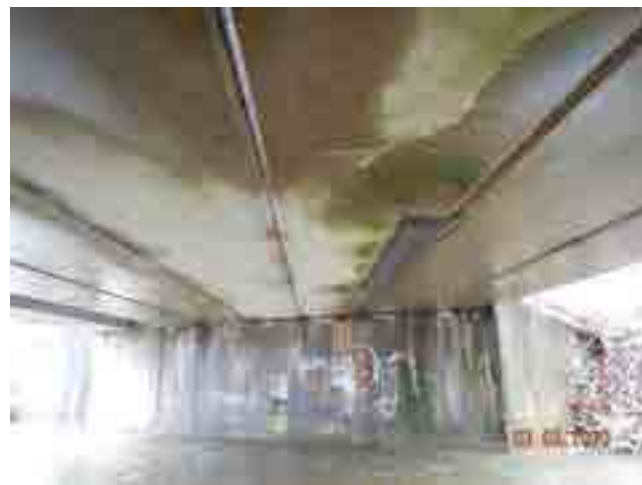
LOOKING WEST AT REPAIRED BEAM 3
