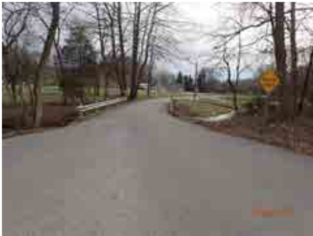
LOOKING SOUTH FROM ROAD
