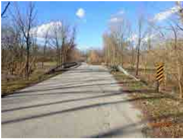
LOOKING NORTH FROM ROAD
