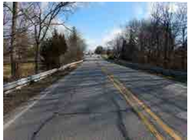
LOOKING NORTH FROM ROAD
