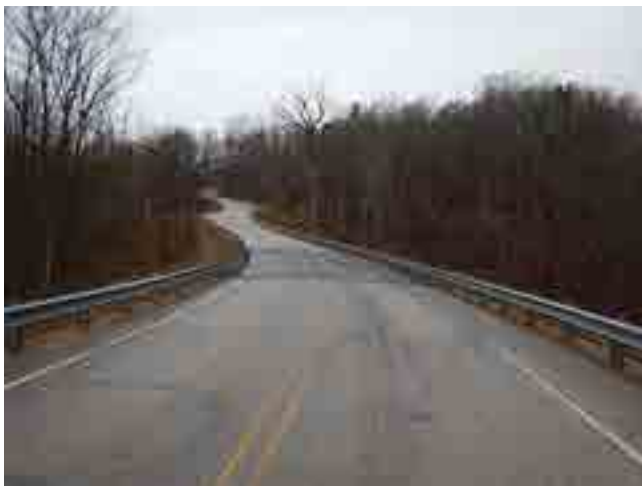
LOOKING WEST FROM ROAD
