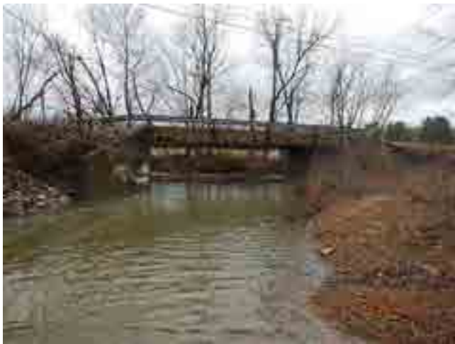
LOOKING WEST THROUGH CHANNEL
