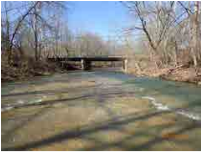
LOOKING WEST THROUGH CHANNEL
