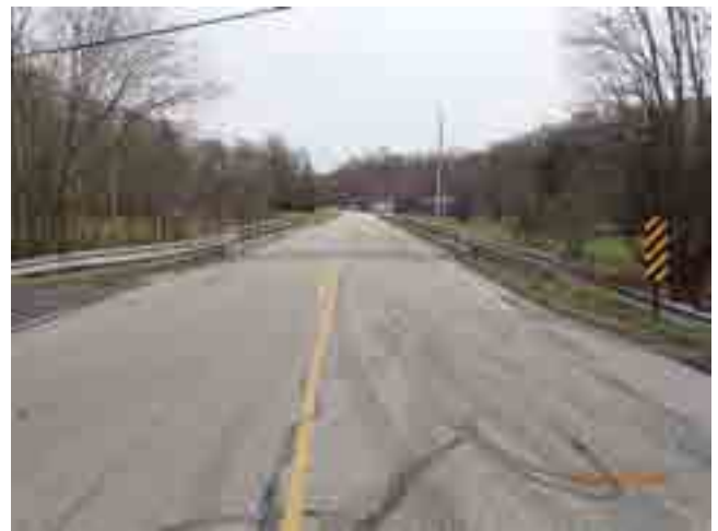
LOOKING SOUTH FROM ROAD
