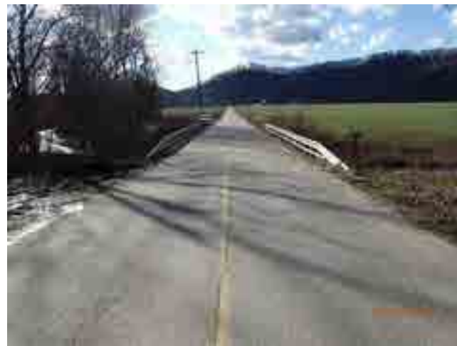
LOOKING WEST FROM ROAD
