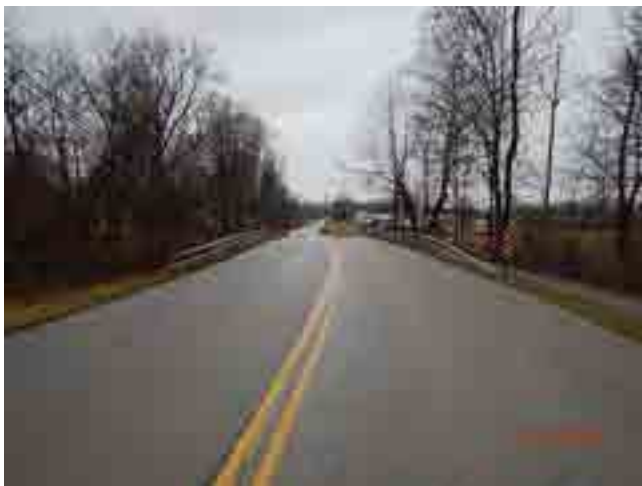
LOOKING NORTH FROM ROAD
