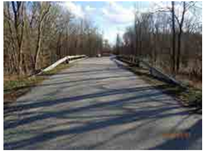
LOOKING SOUTH FROM ROAD
