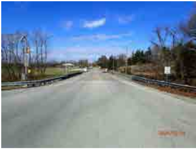
LOOKING WEST FROM ROAD
