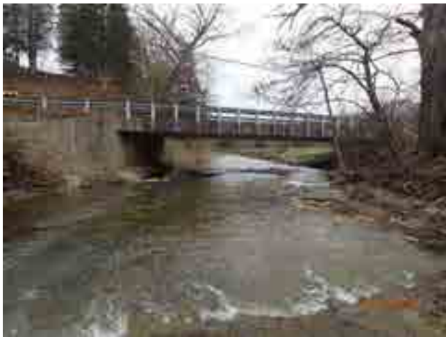
LOOKING SOUTH THROUGH CHANNEL
