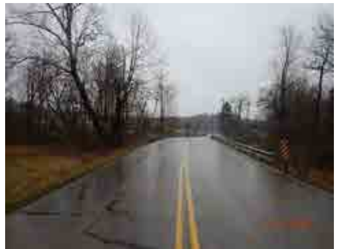
LOOKING SOUTH FROM ROAD
