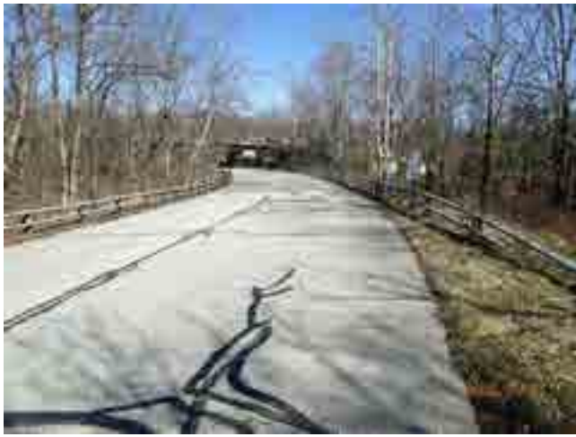
LOOKING NORTH FROM ROAD
