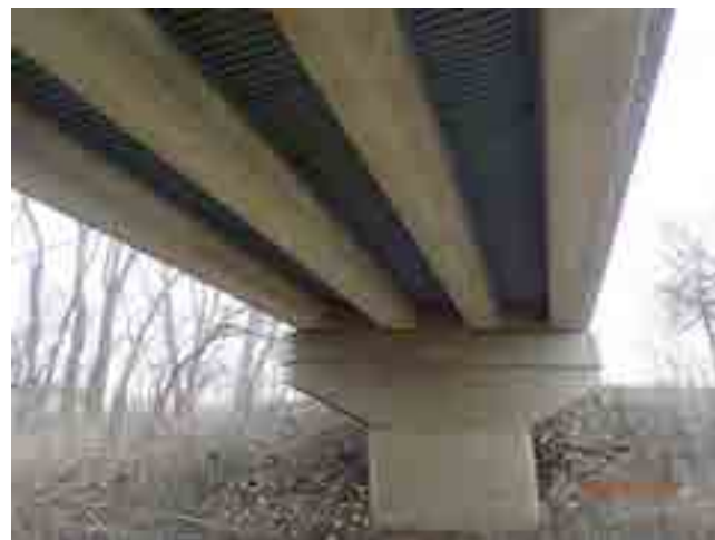
LOOKING EAST AT EAST PIER
