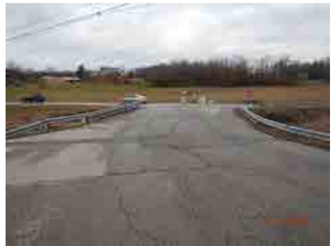
LOOKING NORTH FROM ROAD
