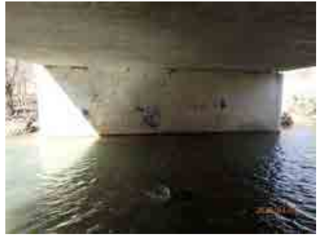
NORTH PIER, CENTER SPAN
