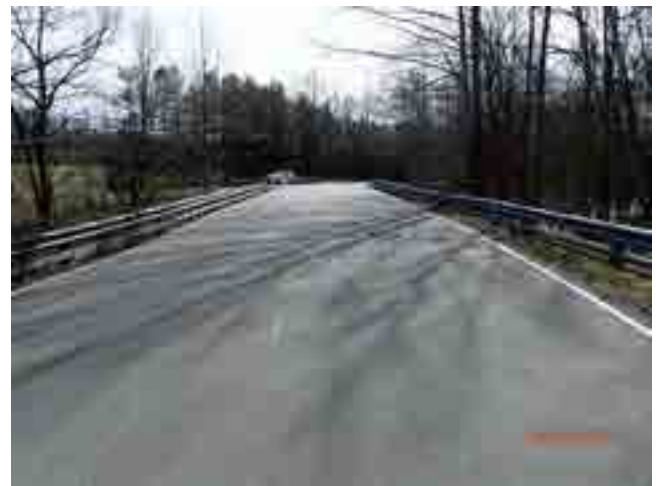
LOOKING SOUTH FROM ROAD
