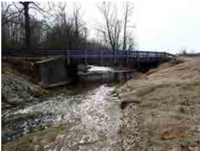
LOOKING SOUTH THROUGH CHANNEL
