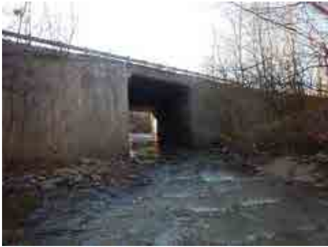
LOOKING EAST DOWNSTREAM
