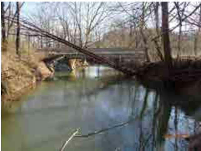
LOOKING NORTH THROUGH CHANNEL
