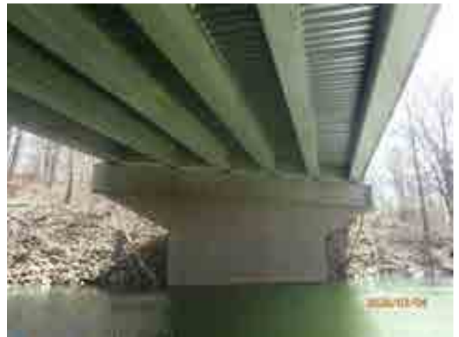
LOOKING SOUTH AT SOUTH PIER
