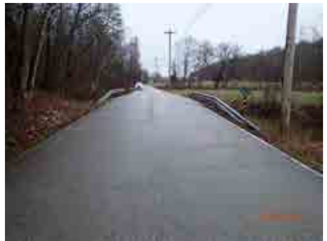
LOOKING SOUTH FROM ROAD
