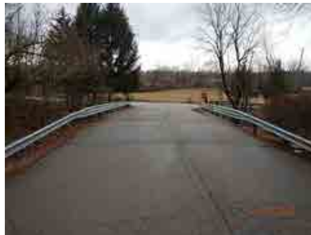
LOOKING WEST FROM ROAD
