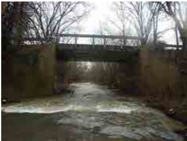
LOOKING WEST THROUGH CHANNEL
