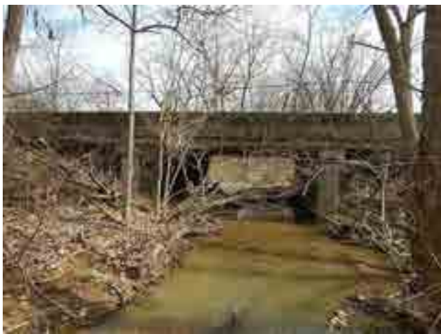
LOOKING EAST DOWNSTREAM
