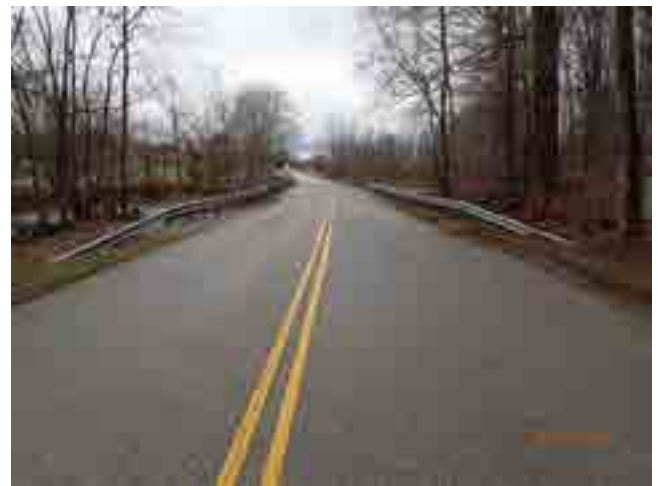
LOOKING NORTH FROM ROAD
