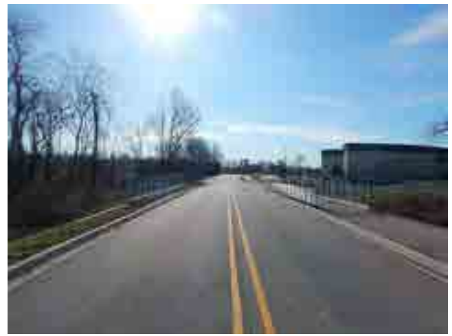
LOOKING SOUTH AT ROAD
