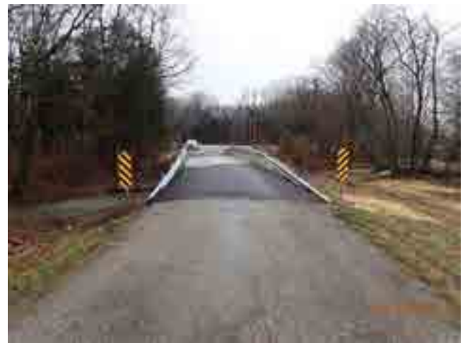
LOOKING WEST FROM ROAD
