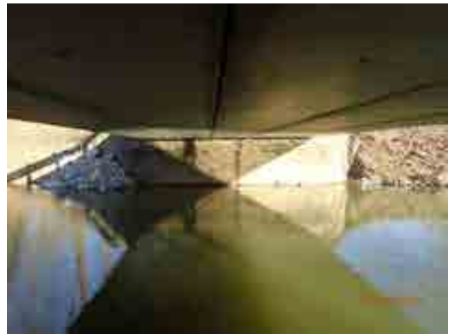
LOOKING EAST AT ABUTMENT
