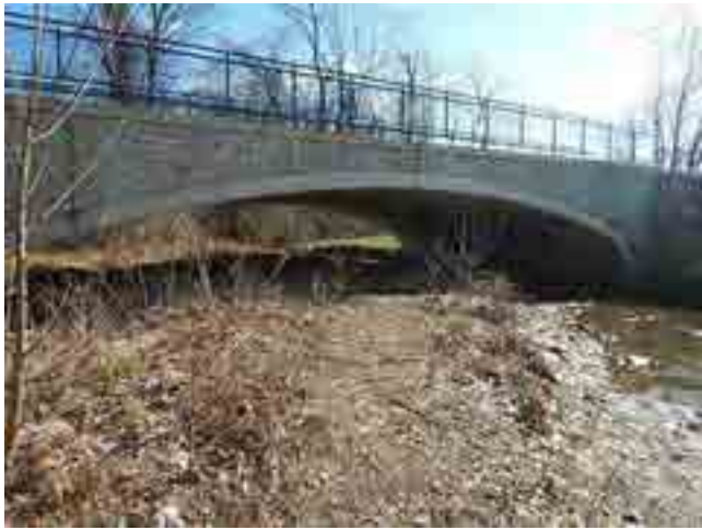
LOOKING EAST DOWNSTREAM
