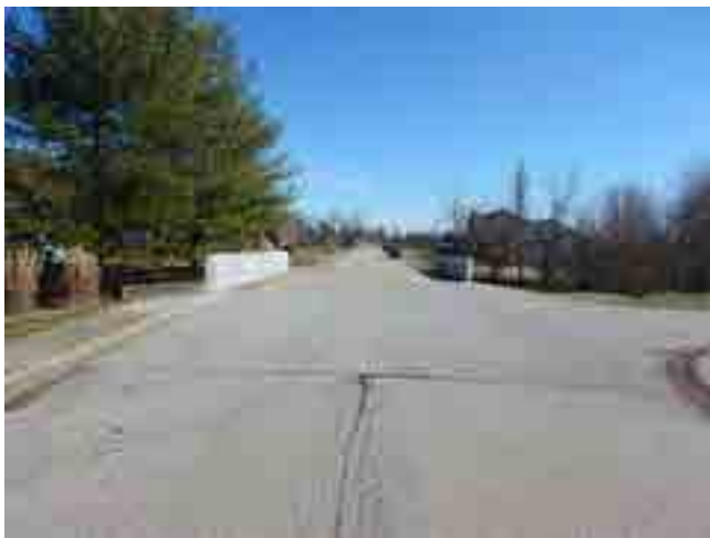
LOOKING NORTH FROM ROAD
