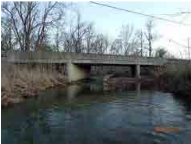
LOOKING EAST FROM CHANNEL
