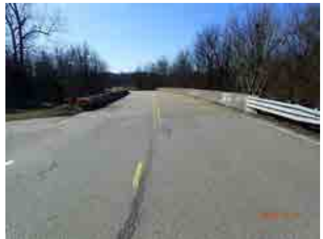
LOOKING SOUTH FROM ROAD
