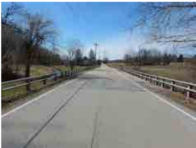
LOOKING WEST FROM ROAD
