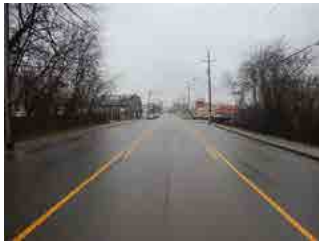
LOOKING SOUTH FROM ROAD
