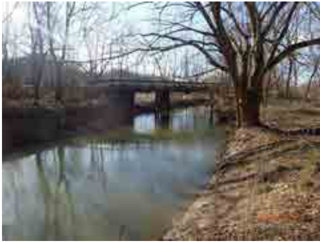
LOOKING WEST FROM CHANNEL
