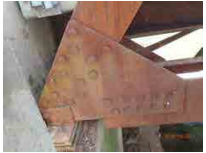
LOOKING AT NORTH TRUSS L12
