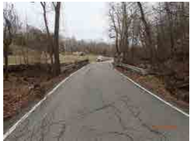
LOOKING SOUTH FROM ROAD
