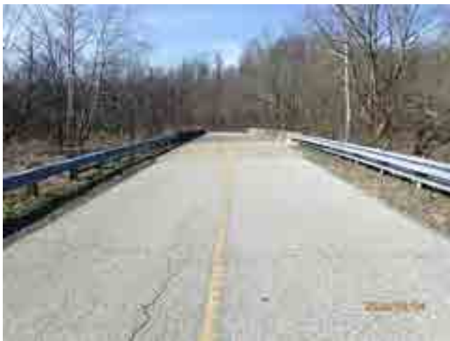
LOOKING WEST FROM ROAD
