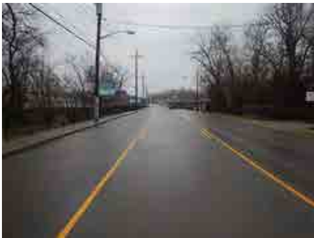
LOOKING NORTH FROM ROAD
