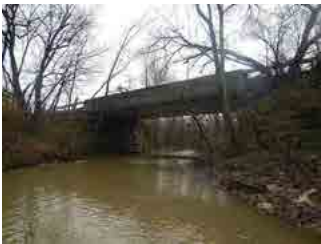
LOOKING WEST DOWNSTREAM
