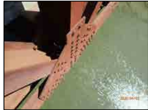
LOOKING AT SOUTH TRUSS L6 OUTSIDE GUSSET PLATE
