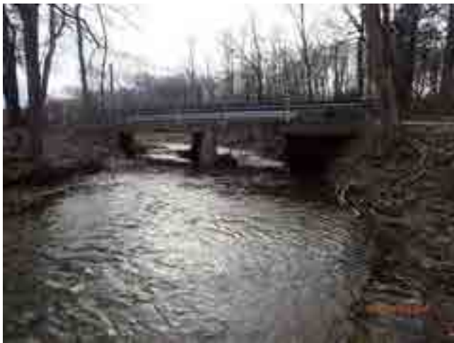
LOOKING WEST FROM CHANNEL
