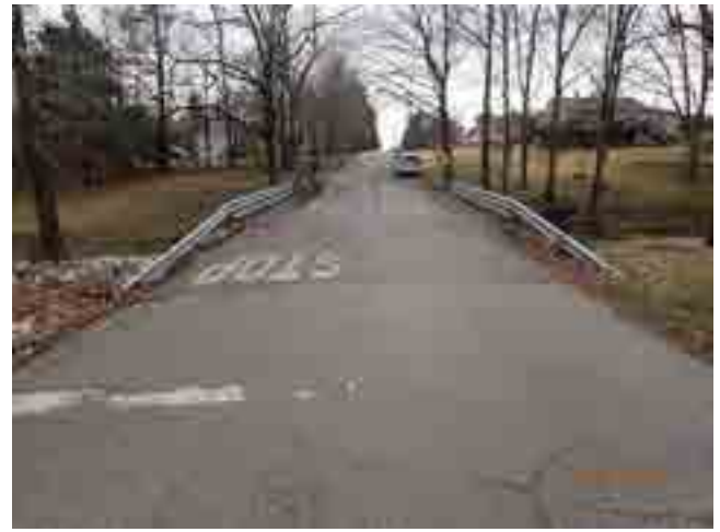
LOOKING WEST FROM ROAD
