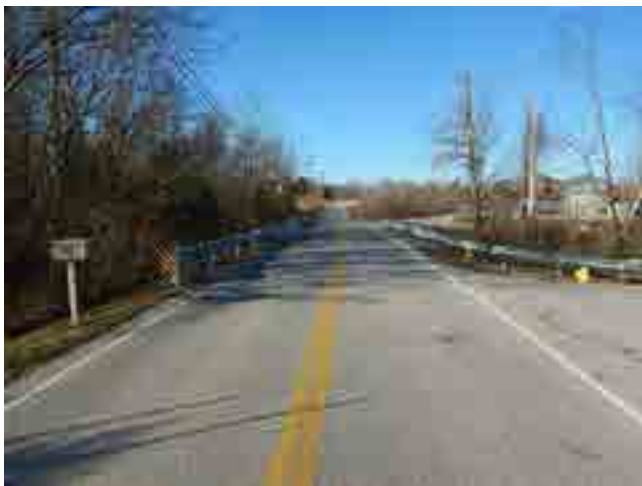
LOOKING WEST FROM ROAD
