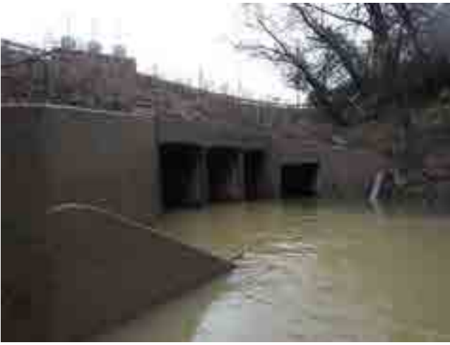
LOOKING AT SOUTH OPENING OF STRUCTURE
