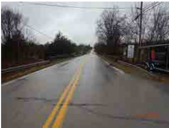
LOOKING WEST FROM ROAD
