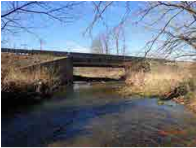
LOOKING SOUTH THROUGH CHANNEL
