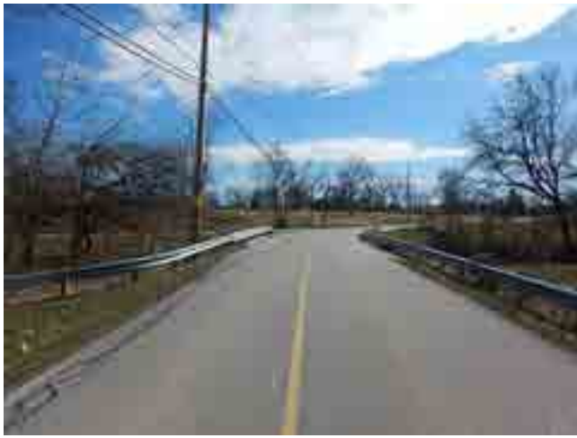
LOOKING SOUTH FROM ROAD
