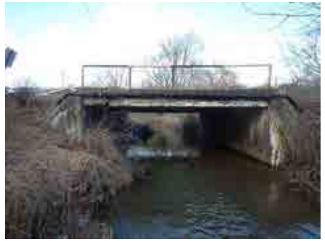
LOOKING EAST THROUGH CHANNEL
