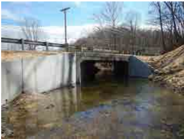
LOOKING EAST THROUGH CHANNEL
