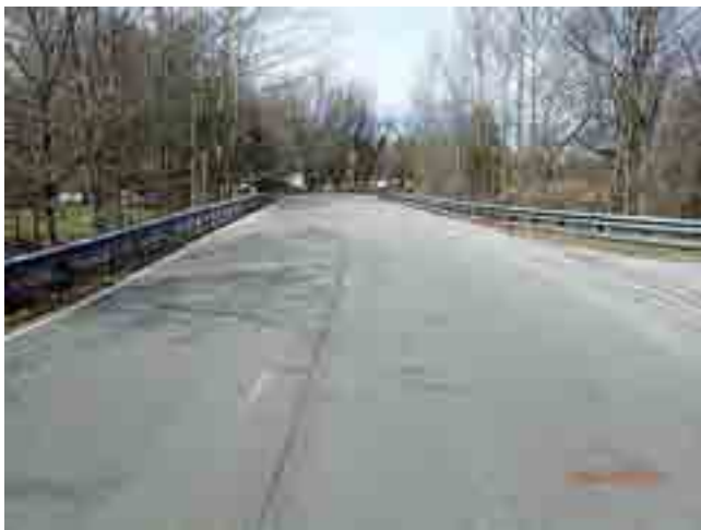
LOOKING NORTH FROM ROAD
