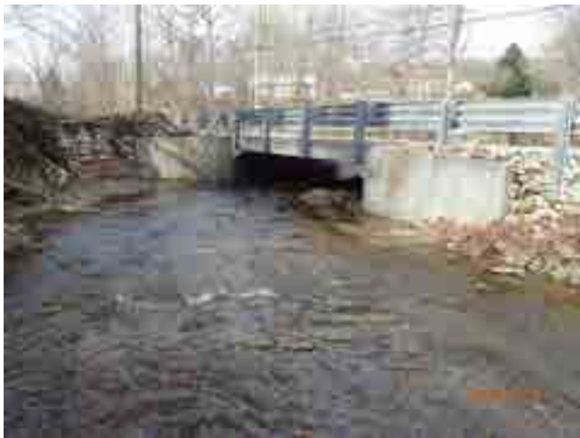
LOOKING WEST THROUGH CHANNEL
