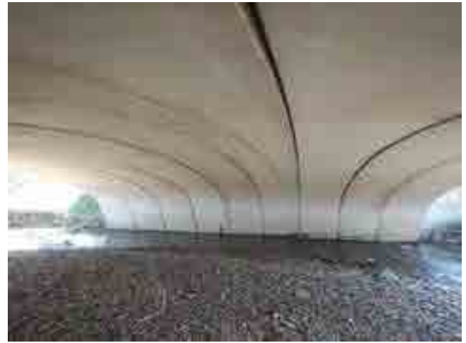
LOOKING SOUTH AT PRECAST UNITS
