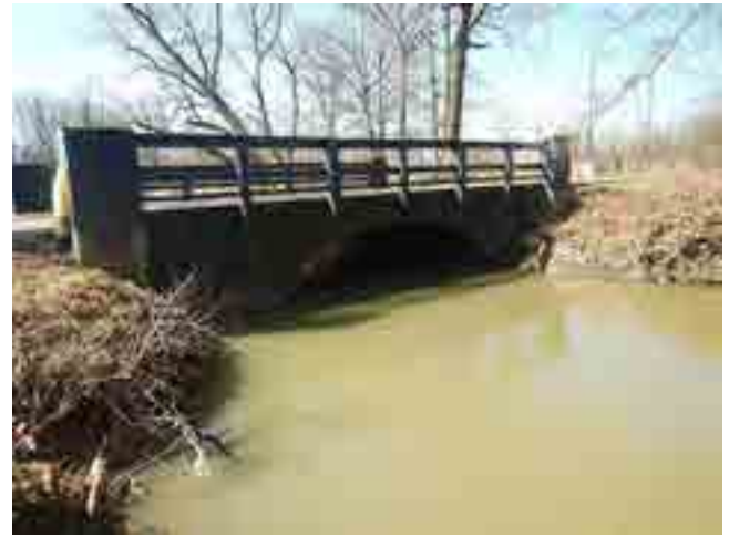
LOOKING SOUTH UPSTREAM
