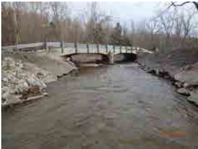
LOOKING SOUTH FROM CHANNEL
