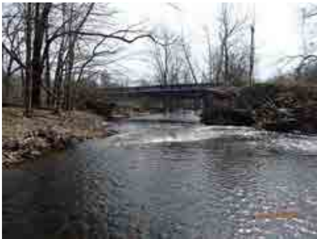
LOOKING SOUTH THROUGH CHANNEL
