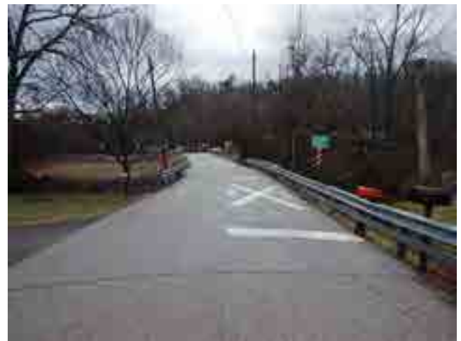
LOOKING SOUTH FROM ROAD
