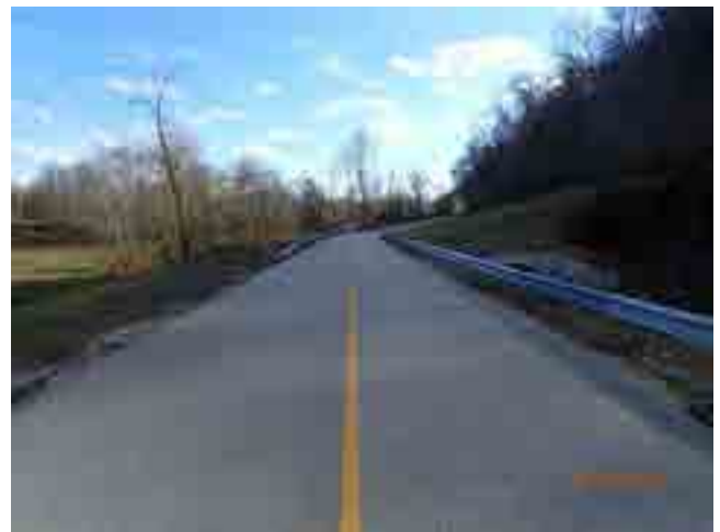
LOOKING SOUTH FROM ROAD
