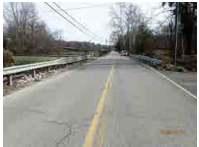
LOOKING NORTH FROM ROAD
