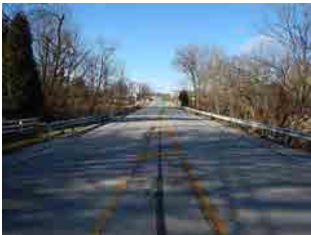
LOOKING SOUTH FROM ROAD
