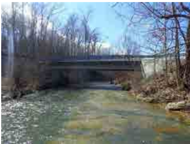
LOOKING WEST THROUGH CHANNEL
