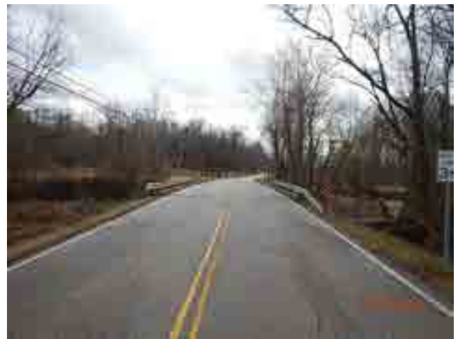
LOOKING SOUTH FROM ROAD
