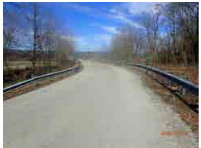
LOOKING NORTH FROM ROAD
