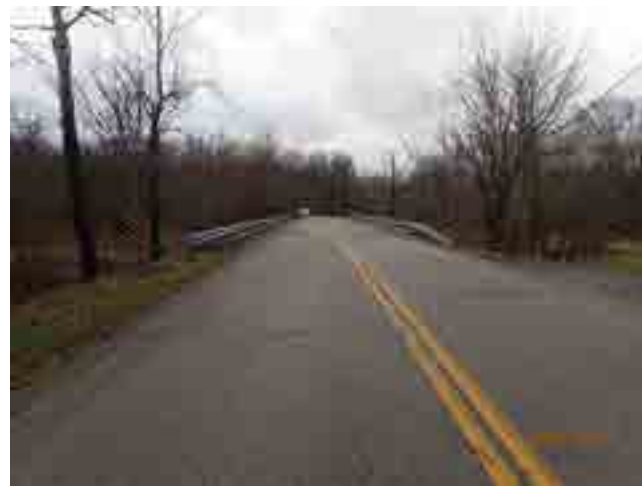
LOOKING WEST FROM ROAD
