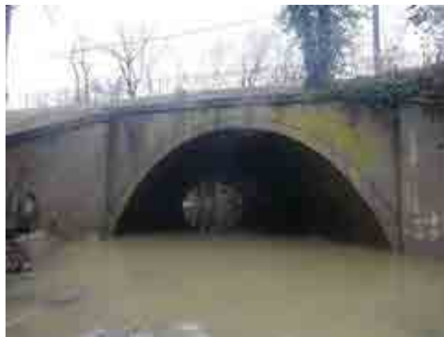
LOOKING EAST FROM CHANNEL
