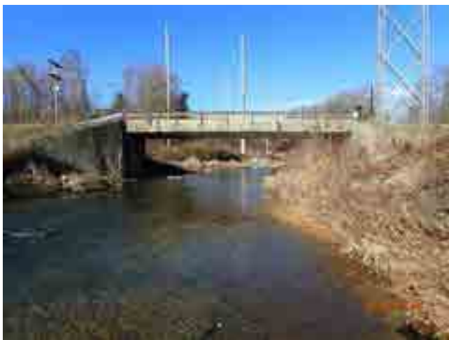
LOOKING WEST THROUGH CHANNEL
