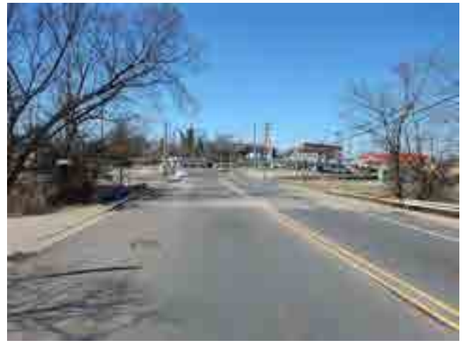
LOOKING WEST FROM ROAD
