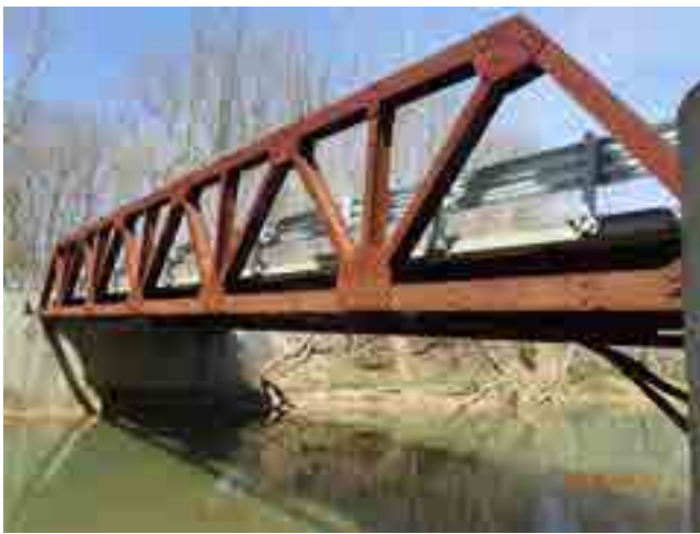
LOOKING NORTH FROM CHANNEL
