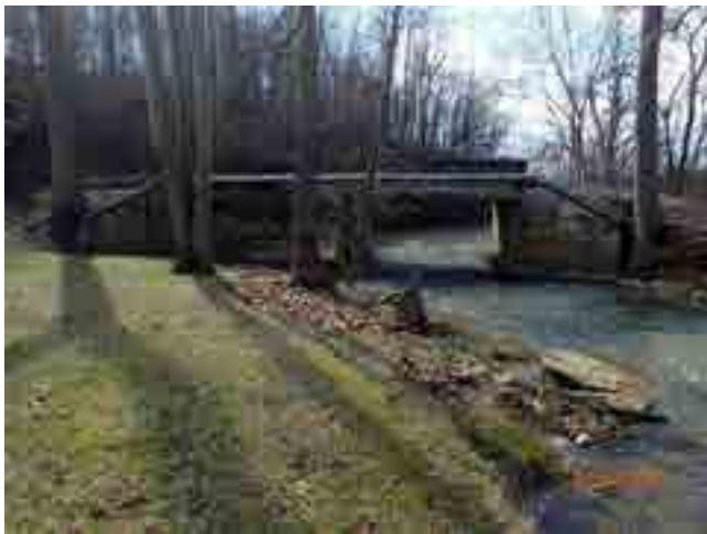
LOOKING WEST THROUGH CHANNEL
