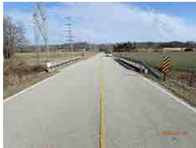
LOOKING NORTH FROM ROAD
