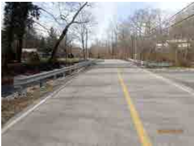
LOOKING SOUTH FROM ROAD
