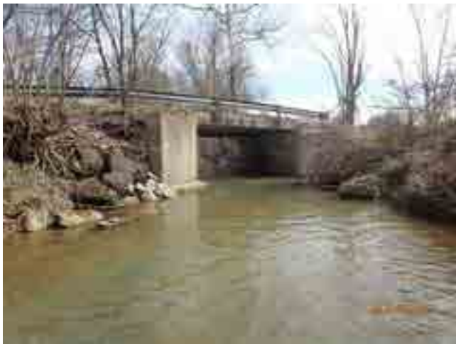
LOOKING EAST THROUGH CHANNEL
