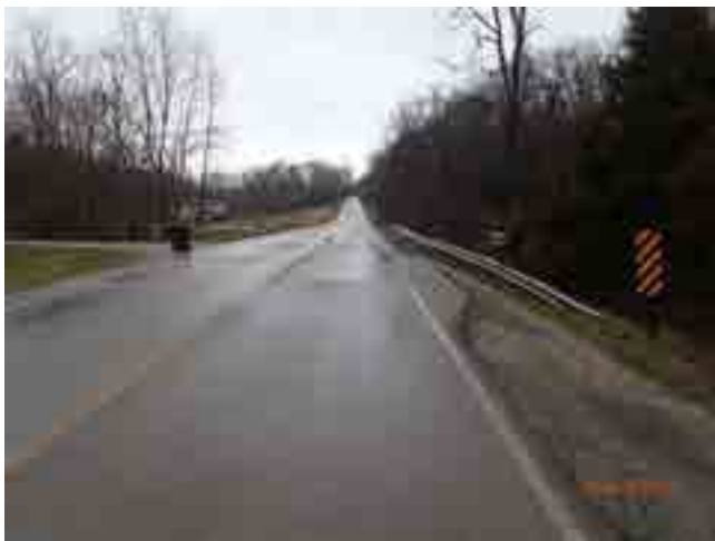
LOOKING NORTH FROM ROAD
