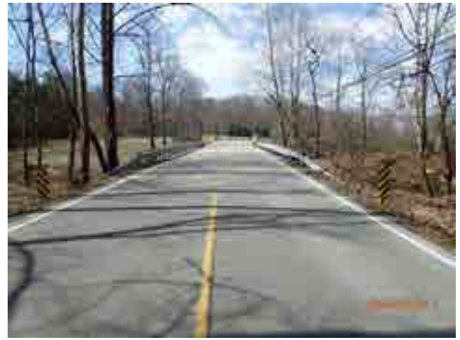
LOOKING WEST FROM ROAD
