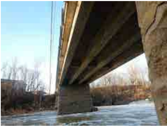
NORTH AT SOUTH SPAN SUPERSTR. AND DECK
