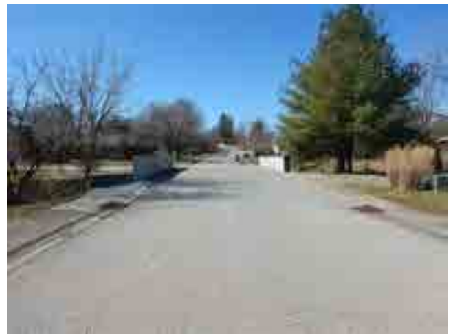
LOOKING SOUTH FROM ROAD
