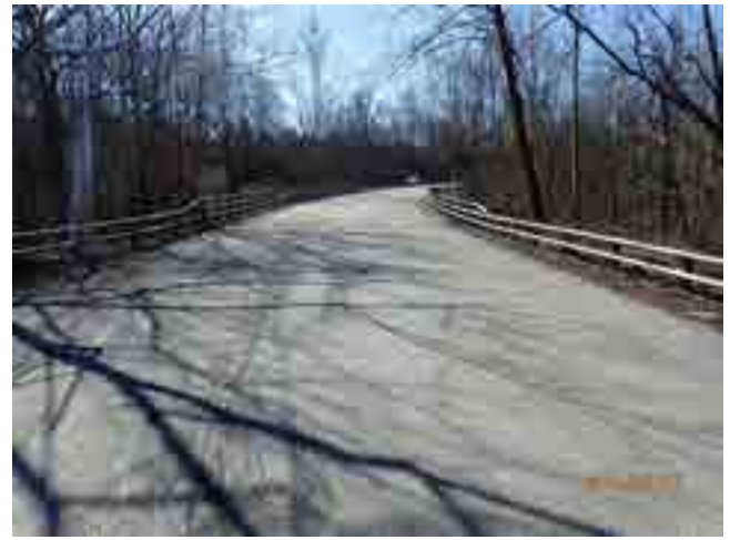
LOOKING SOUTH FROM ROAD
