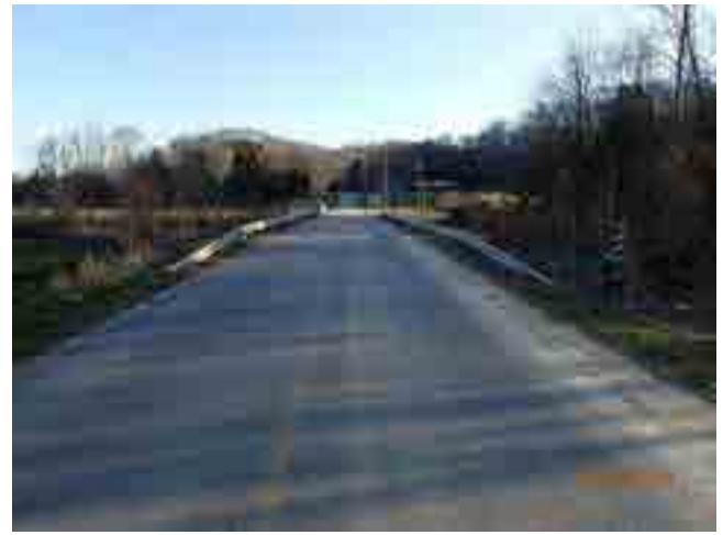
LOOKING SOUTH FROM ROAD
