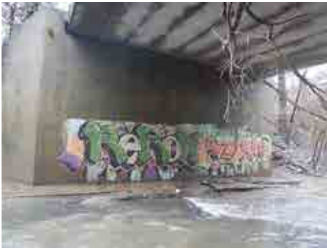
LOOKING SOUTH AT SOUTH BENT FOOTING
