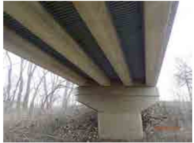
LOOKING EAST AT EAST PIER
