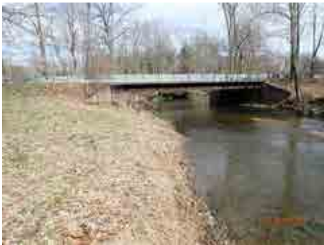
LOOKING NORTH THROUGH CHANNEL
