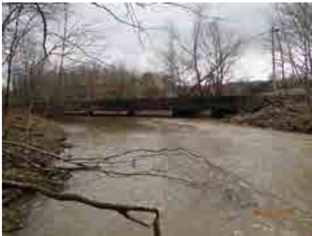
LOOKING WEST THROUGH CHANNEL
