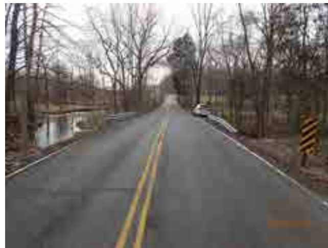
LOOKING WEST FROM ROAD
