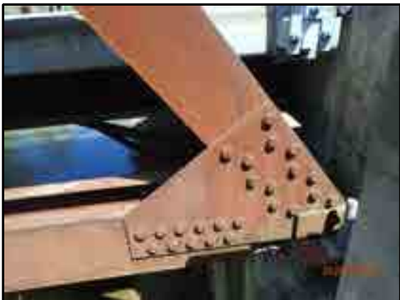
LOOKING AT SOUTH TRUSS L12
