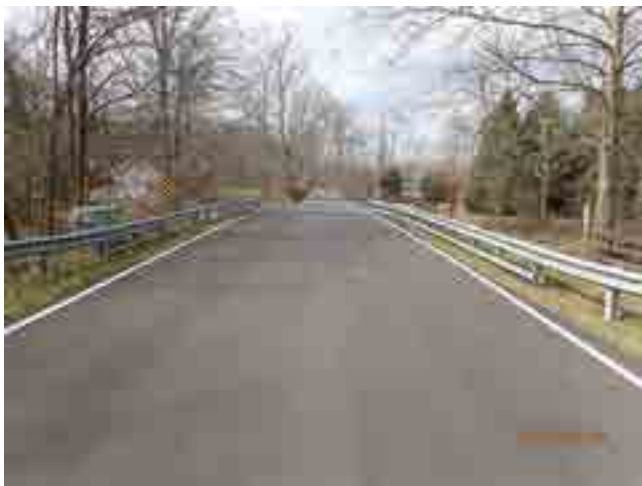
LOOKING WEST FROM ROAD
