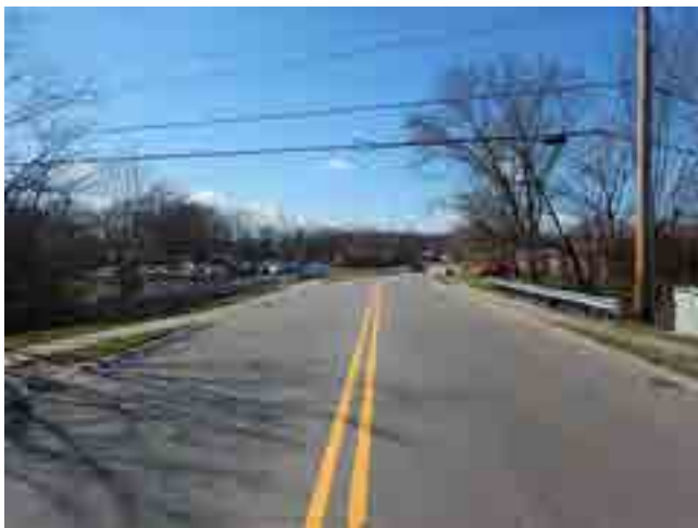
LOOKING WEST FROM ROAD
