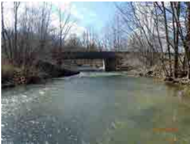
LOOKING WEST THROUGH CHANNEL
