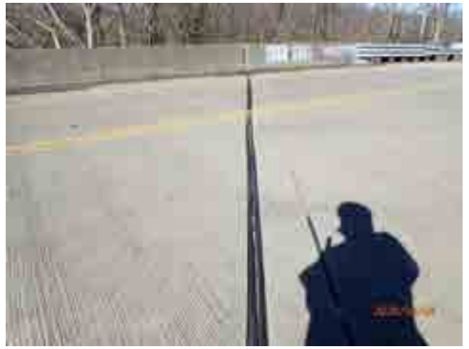
NORTH EXPANSION JOINT
