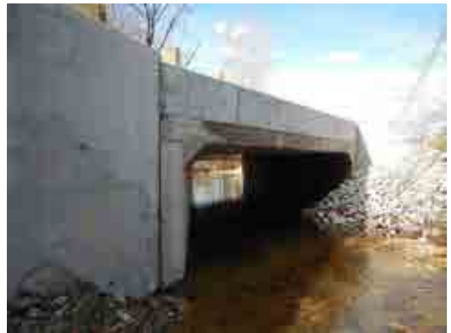
LOOKING WEST DOWNSTREAM
