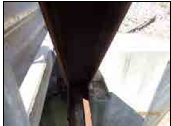
LOOKING AT NORTH TRUSS L0
