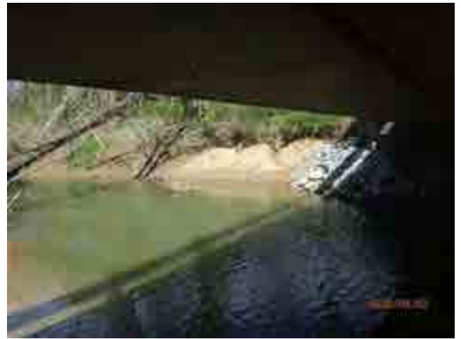
LOOKING AT NE CORNERS
