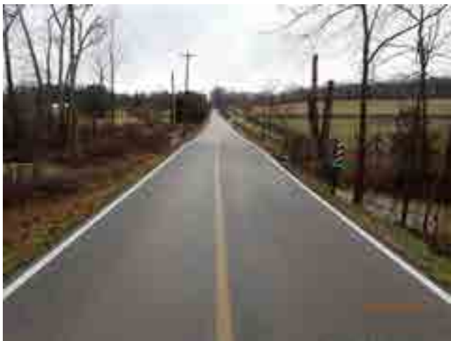
LOOKING WEST FROM ROAD
