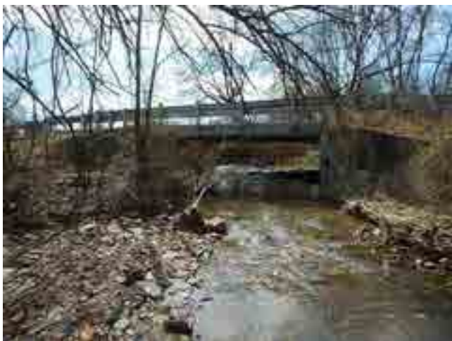
LOOKING WEST DOWNSTREAM
