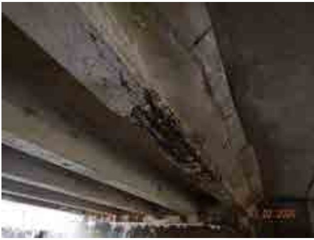
LOOKING SOUTH AT NORTH SPAN WEST COPING T-BEAM
