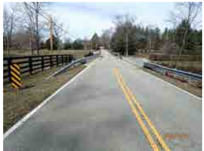
LOOKING NORTH FROM ROAD
