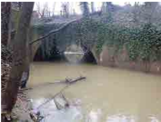
LOOKING WEST FROM CHANNEL
