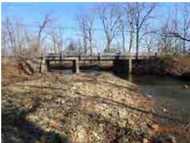
LOOKING NORTH THROUGH CHANNEL
