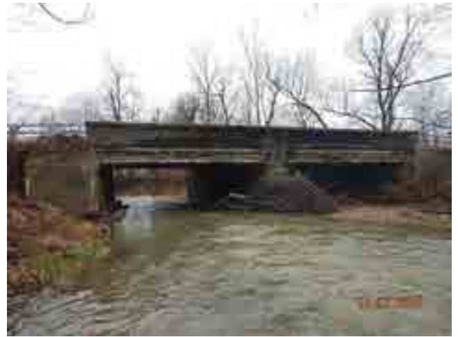
LOOKING WEST DOWNSTREAM
