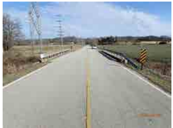
LOOKING NORTH FROM ROAD
