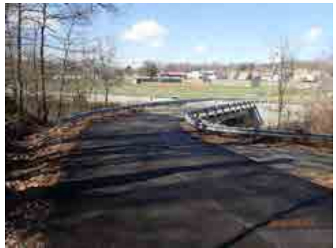
LOOKING NORTH FROM ROAD
