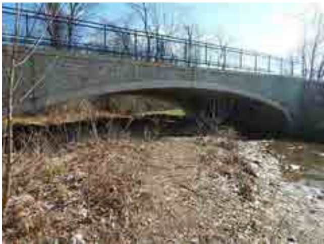
LOOKING EAST DOWNSTREAM
