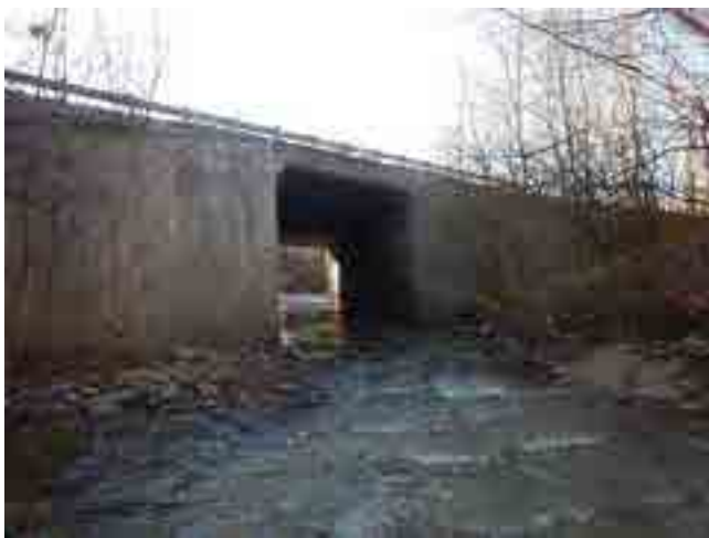
LOOKING EAST DOWNSTREAM
