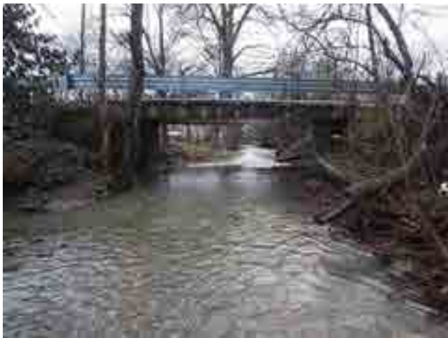
LOOKING EAST DOWNSTREAM
