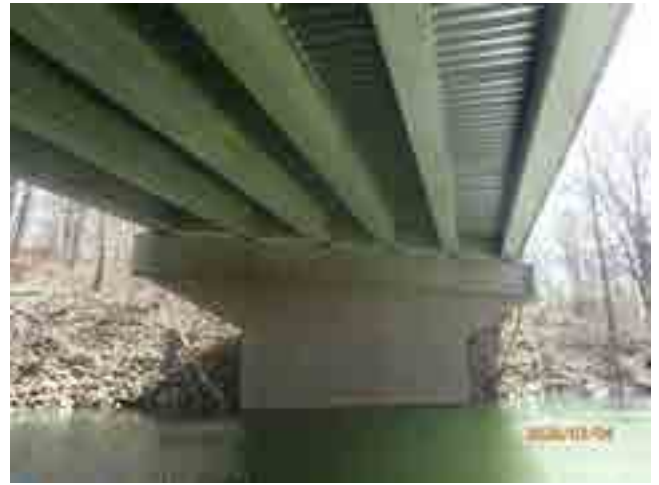
LOOKING SOUTH AT SOUTH PIER
