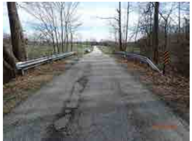
LOOKING SE FROM ROAD
