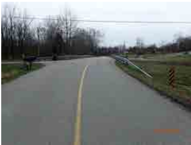
LOOKING WEST FROM ROAD
