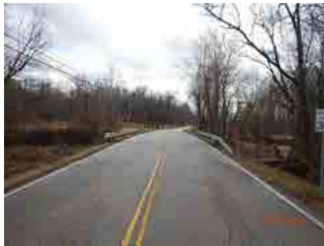
LOOKING SOUTH FROM ROAD
