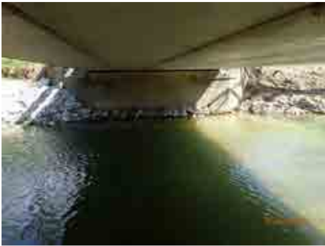
LOOKING AT EAST ABUTMENT
