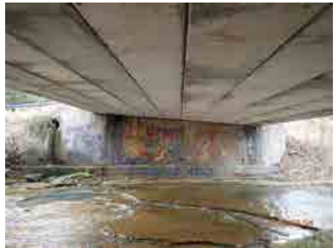
LOOKING NORTH AT ABUTMENT
