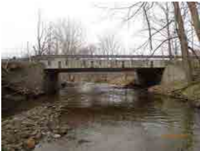
LOOKING WEST THROUGH CHANNEL
