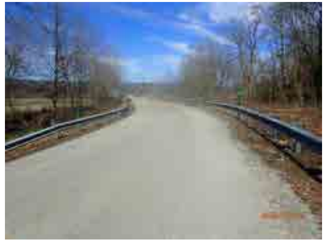
LOOKING NORTH FROM ROAD
