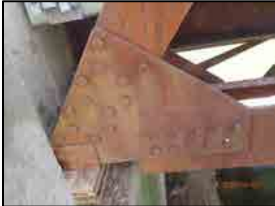
LOOKING AT NORTH TRUSS L12
