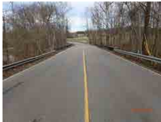
LOOKING NORTH FROM ROAD
