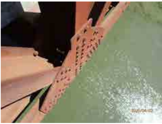
LOOKING AT SOUTH TRUSS L6 OUTSIDE GUSSET PLATE
