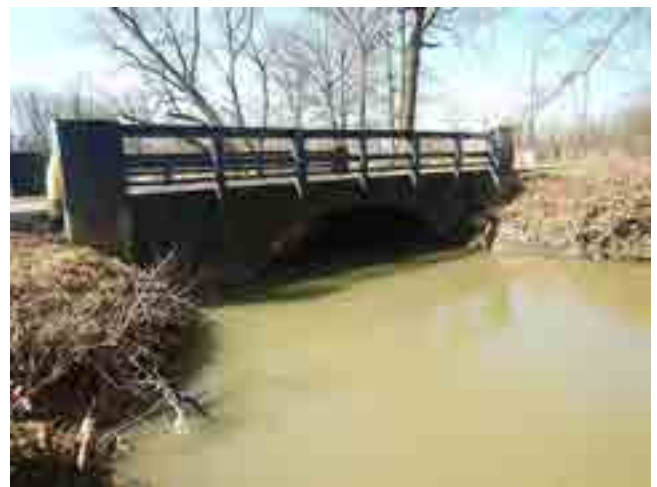
LOOKING SOUTH UPSTREAM
