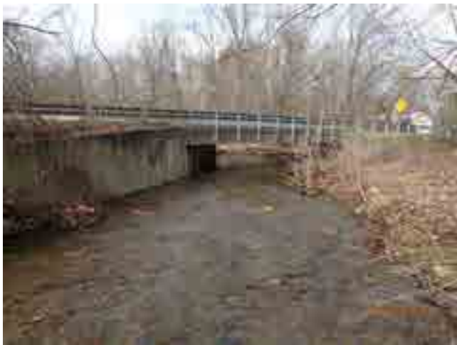
LOOKING WEST THROUGH CHANNEL
