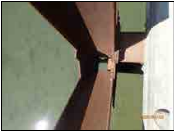
LOOKING AT SOUTH TRUSS L6
