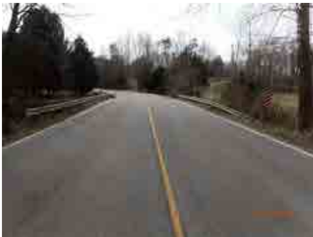
LOOKING SOUTH FROM ROAD
