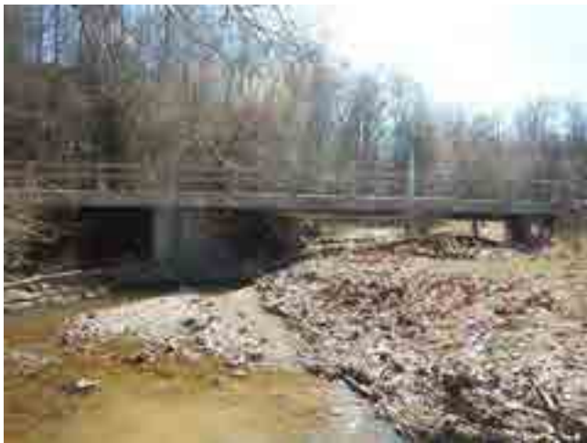
LOOKING SOUTH THROUGH CHANNEL
