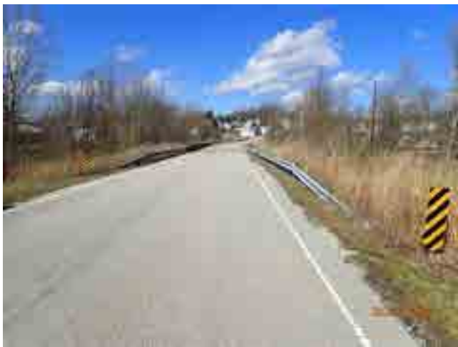
LOOKING NORTH FROM ROAD
