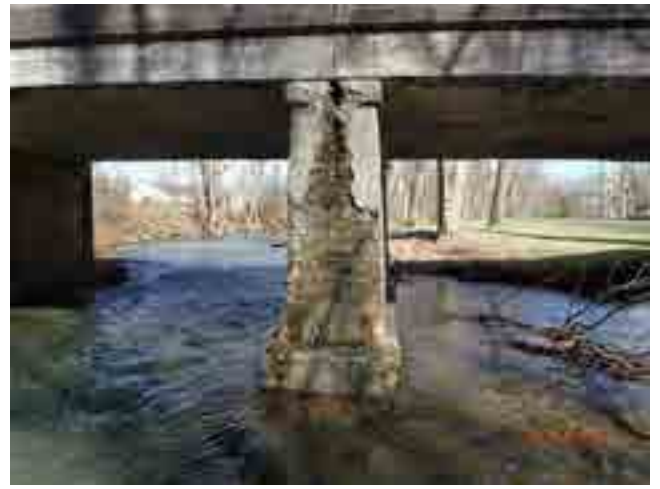
DOWNSTREAM PIER NOSE
