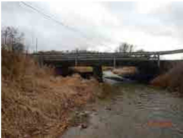
LOOKING WEST FROM CHANNEL
