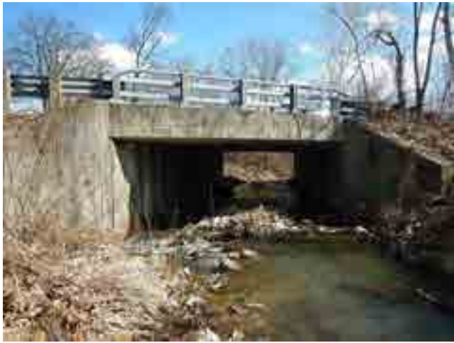
LOOKING EAST DOWNSTREAM
