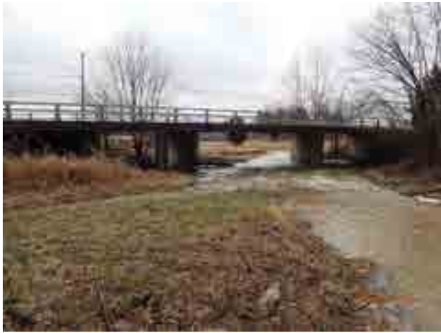
LOOKING EAST THROUGH CHANNEL
