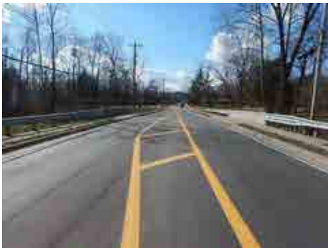
LOOKING WEST FROM ROAD
