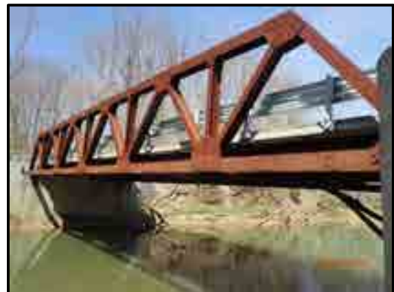
LOOKING NORTH FROM CHANNEL
