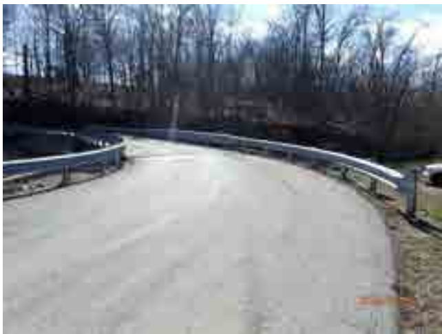
LOOKING SOUTH FROM ROAD
