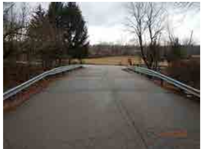
LOOKING WEST FROM ROAD
