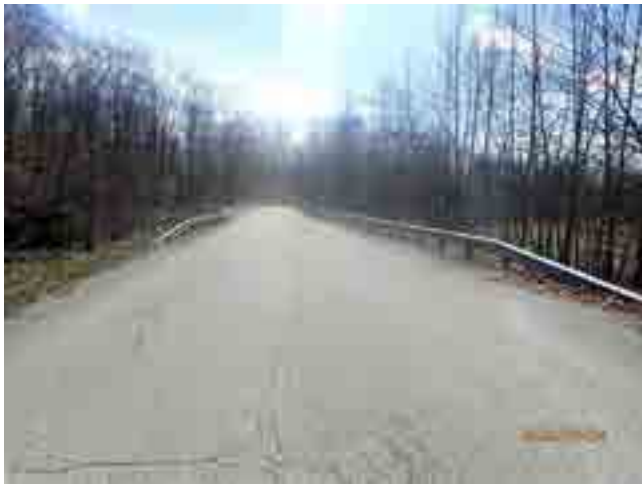
LOOKING SOUTH FROM ROAD
