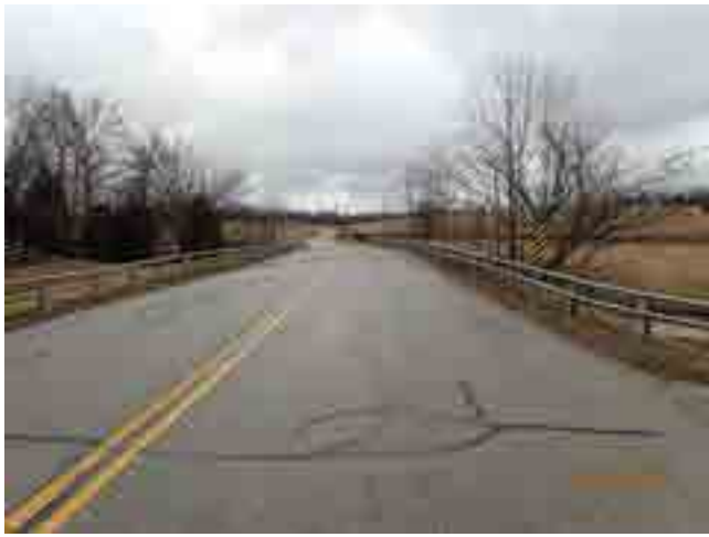
LOOKING NORTH FROM ROAD
