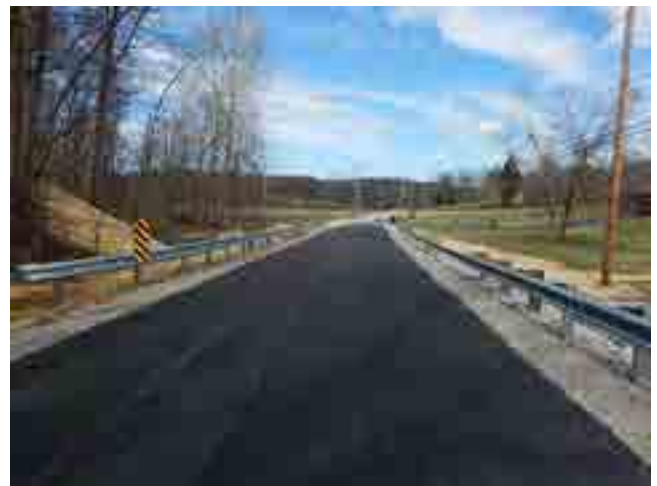
LOOKING NORTH FROM ROAD
