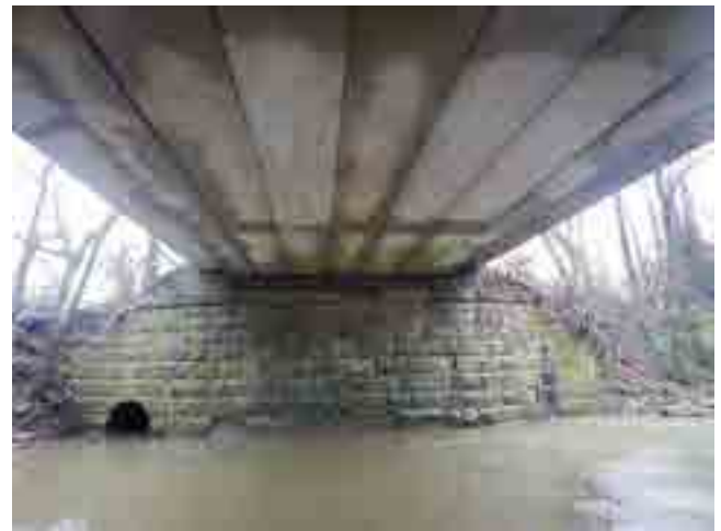
LOOKING SOUTH AT SOUTH ABUTMENT
