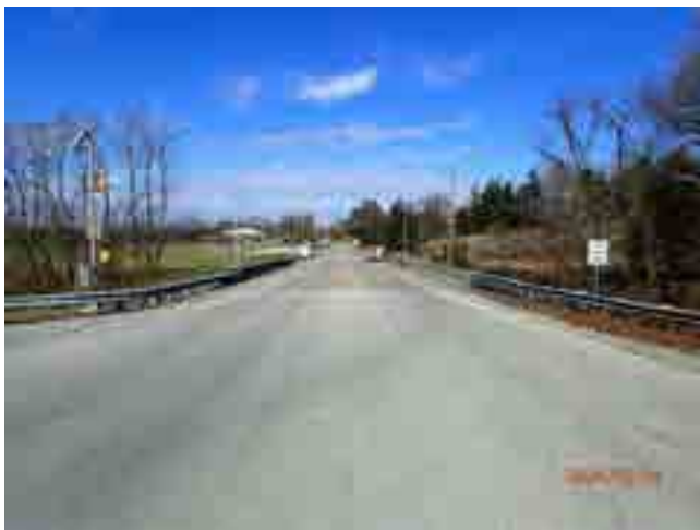
LOOKING WEST FROM ROAD
