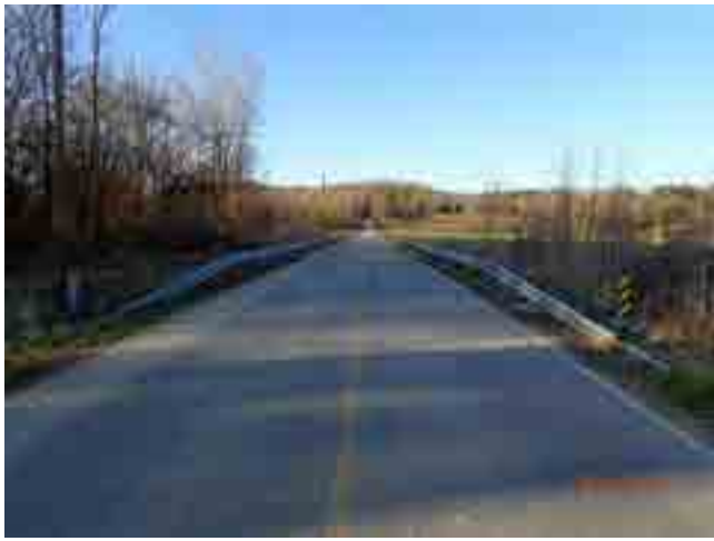
LOOKING NORTH FROM ROAD
