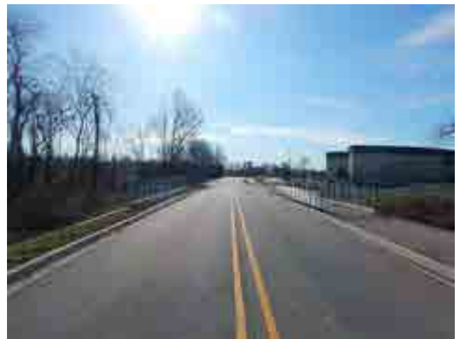
LOOKING SOUTH AT ROAD
