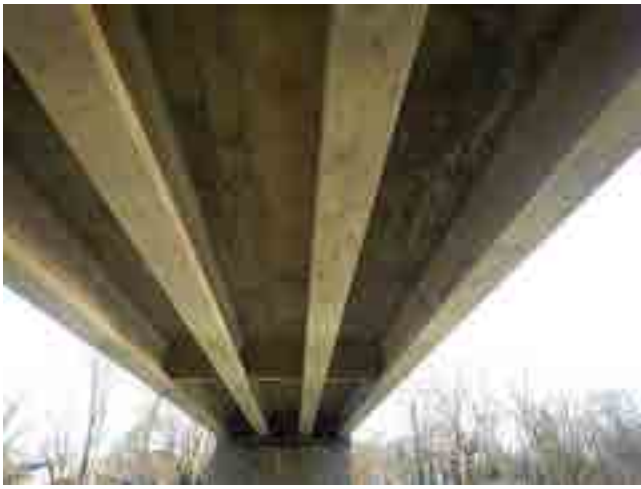
S AT NORTH SPAN SUPERSTRUCTURE AND DECK
