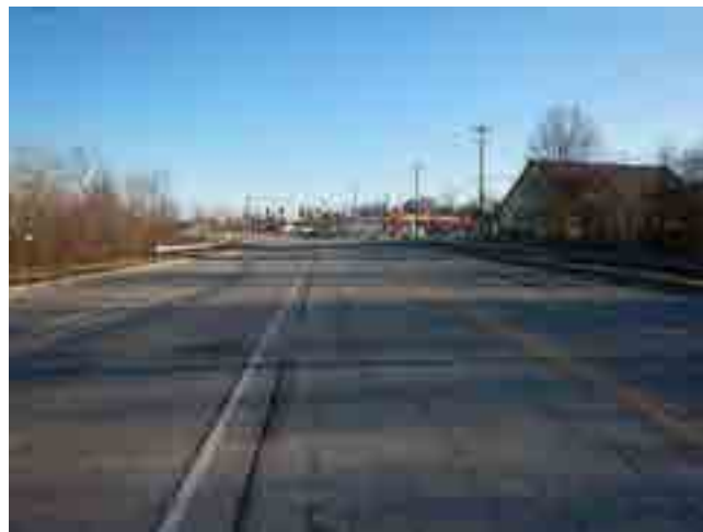
LOOKING NORTH FROM ROAD
