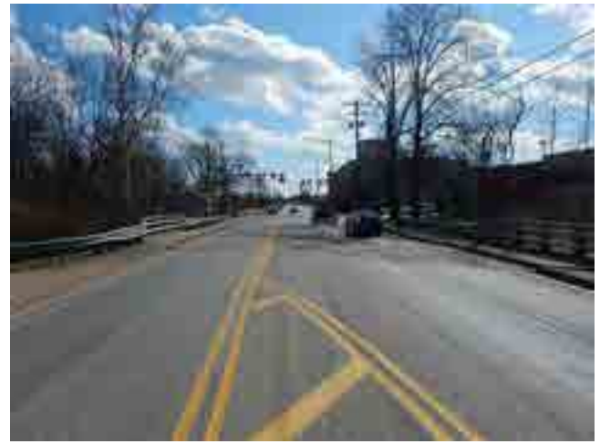
LOOKING SOUTH FROM ROAD
