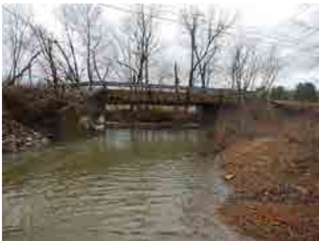
LOOKING WEST THROUGH CHANNEL
