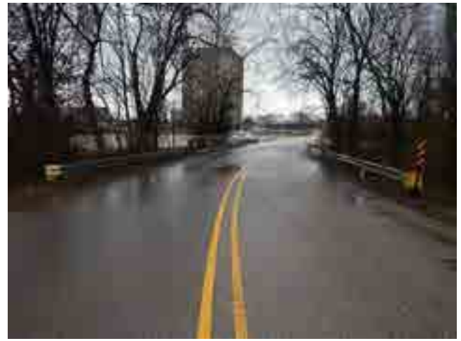
LOOKING SOUTH FROM ROAD
