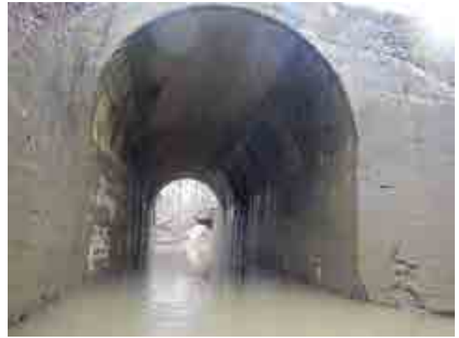
LOOKING SOUTH AT CULVERT INTERIOR
