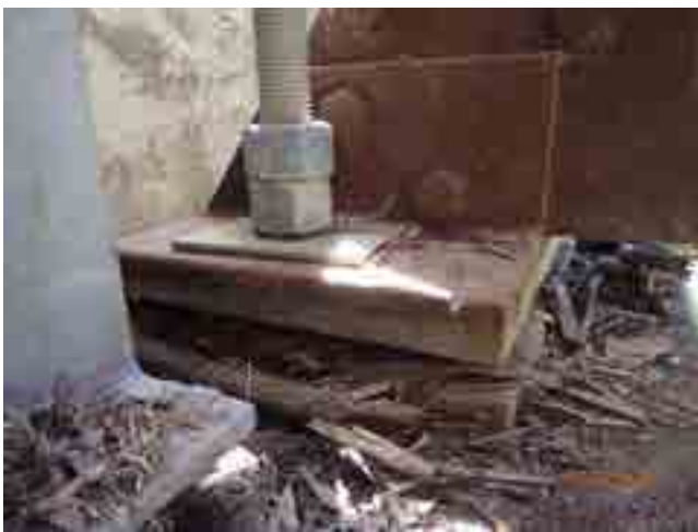
LOOKING AT SOUTH TRUSS L12
