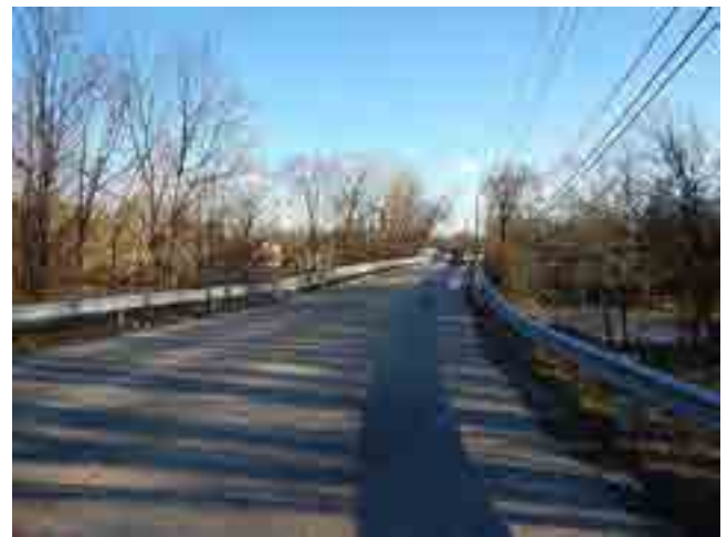
LOOKING SOUTH FROM ROAD
