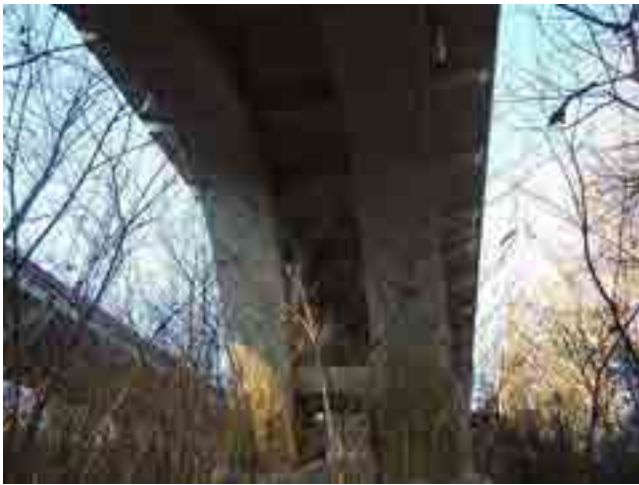
LOOKING WEST AT APPROACH SPANS
