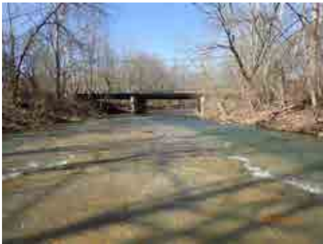
LOOKING WEST THROUGH CHANNEL
