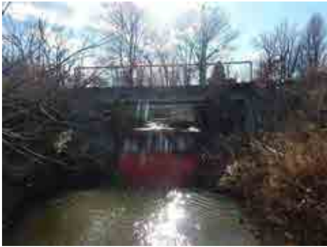
LOOKING WEST DOWNSTREAM
