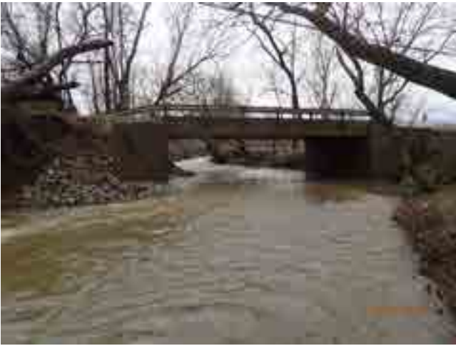
LOOKING SOUTH FROM CHANNEL
