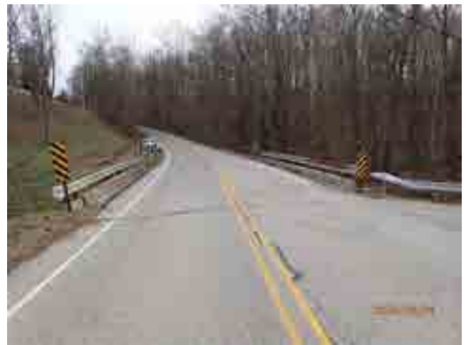
LOOKING SOUTH FROM ROAD
