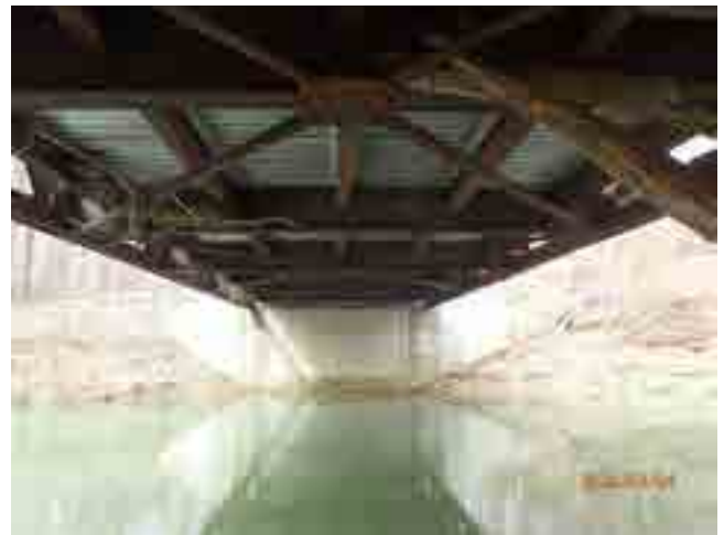
LOOKING WEST AT ABUTMENT
