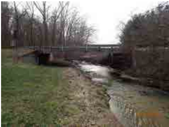
LOOKING WEST THROUGH CHANNEL
