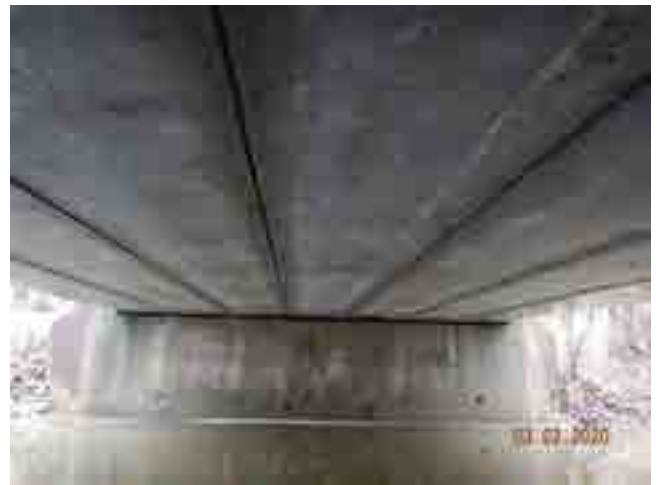
LOOKING EAST AT SUPERSTRUCTURE AND EAST
