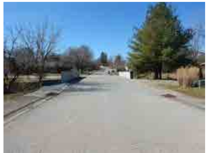
LOOKING SOUTH FROM ROAD
