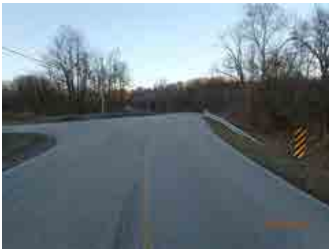
LOOKING NORTH FROM ROAD
