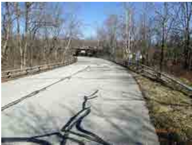
LOOKING NORTH FROM ROAD
