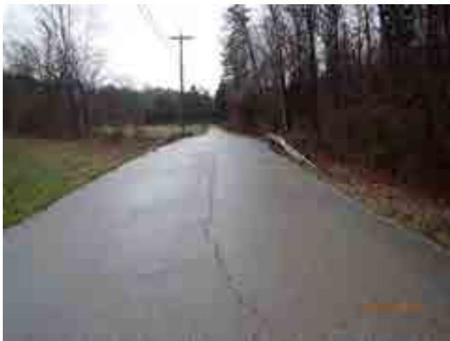
LOOKING NORTH FROM ROAD
