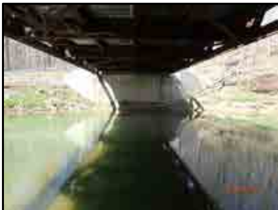
LOOKING AT WEST ABUTMENT
