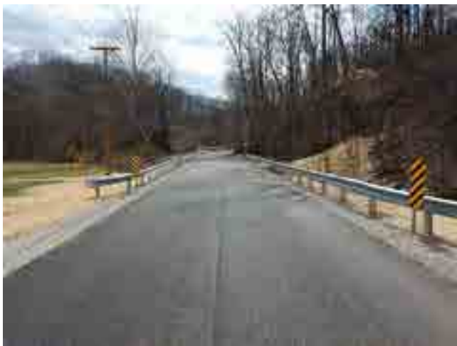
LOOKING SOUTH FROM ROAD
