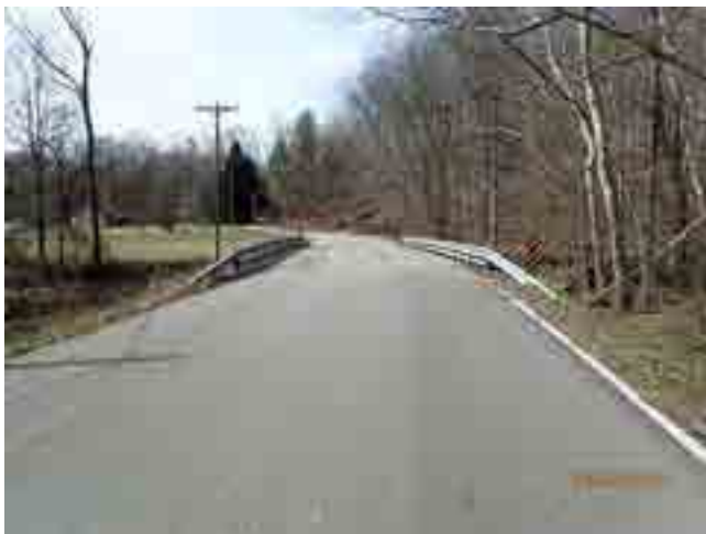
LOOKING WEST FROM ROAD
