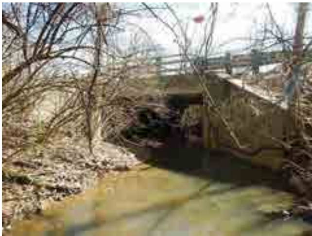
LOOKING SOUTH DOWNSTREAM
