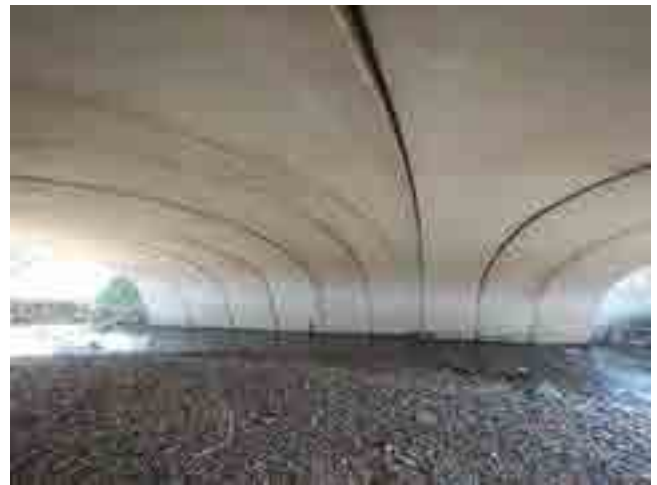
LOOKING SOUTH AT PRECAST UNITS
