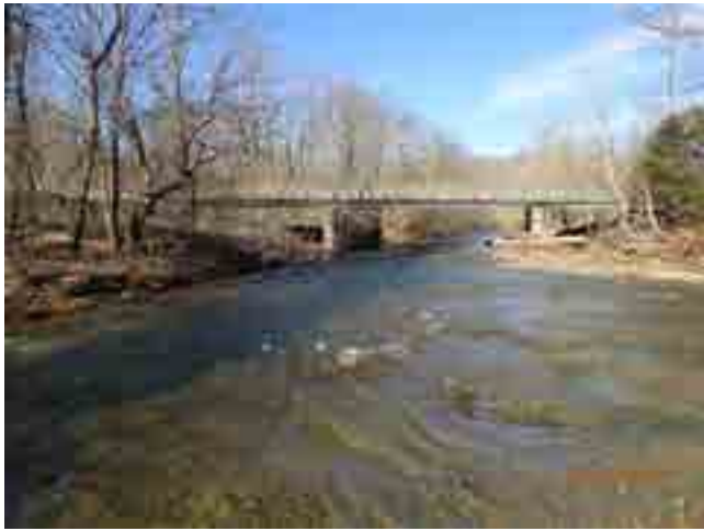
LOOKING WEST THROUGH CHANNEL
