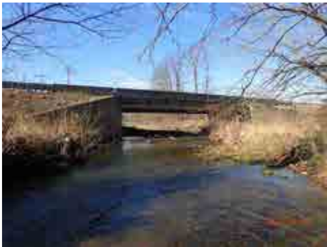
LOOKING SOUTH THROUGH CHANNEL
