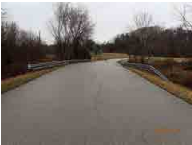
LOOKING WEST FROM ROAD
