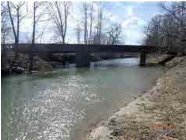
LOOKING SOUTH THROUGH CHANNEL
