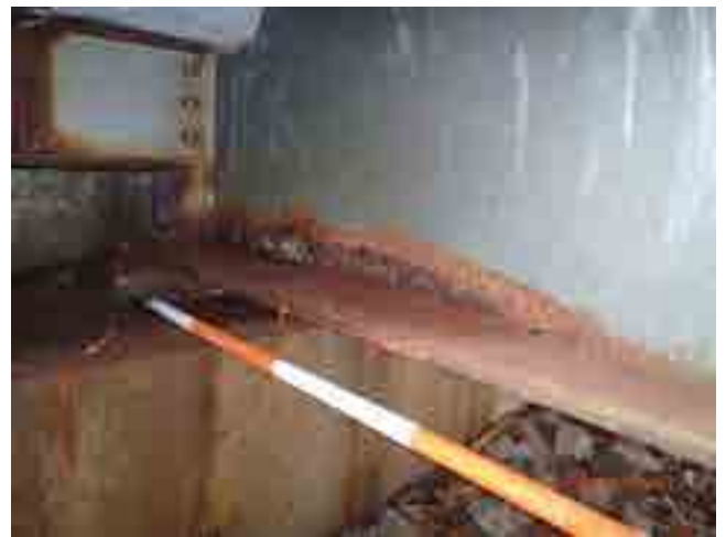
NORTH ABUTMENT BEARING
