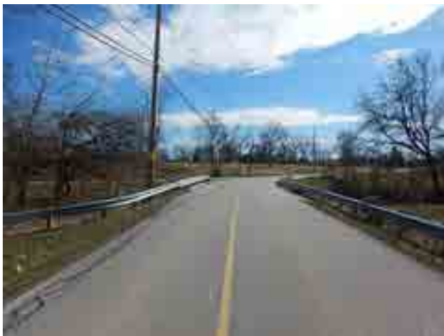
LOOKING SOUTH FROM ROAD
