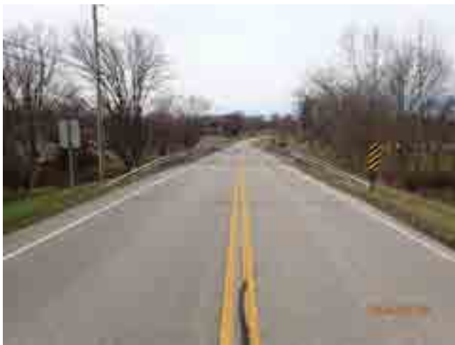
LOOKING NORTH FROM ROAD
