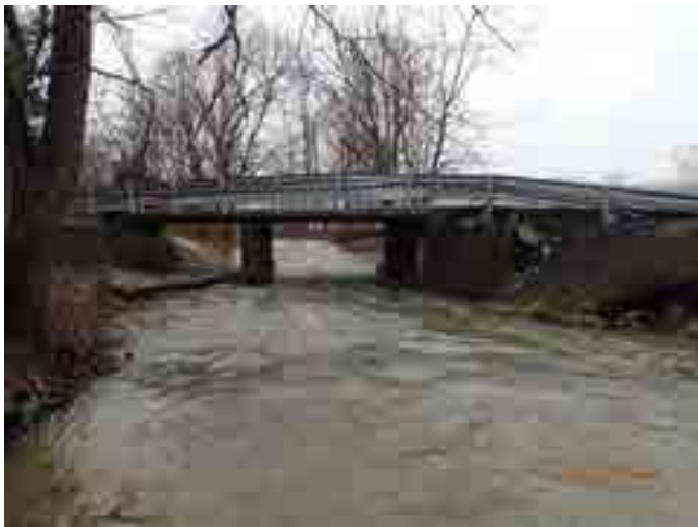
LOOKING NORTH FROM CHANNEL
