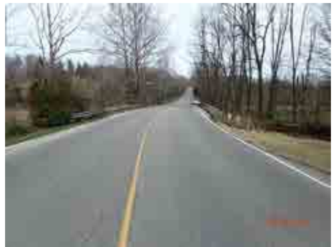
LOOKING NORTH FROM ROAD
