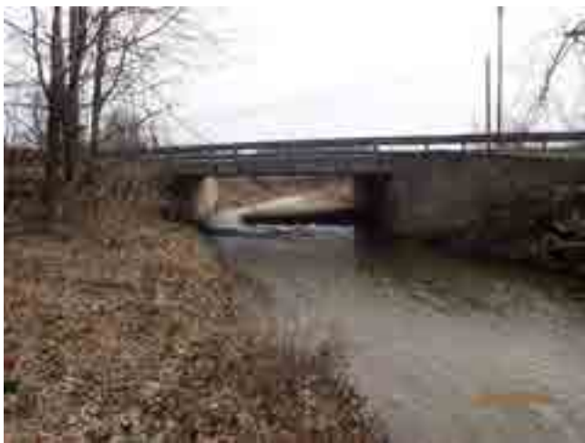
LOOKING SOUTH THROUGH CHANNEL
