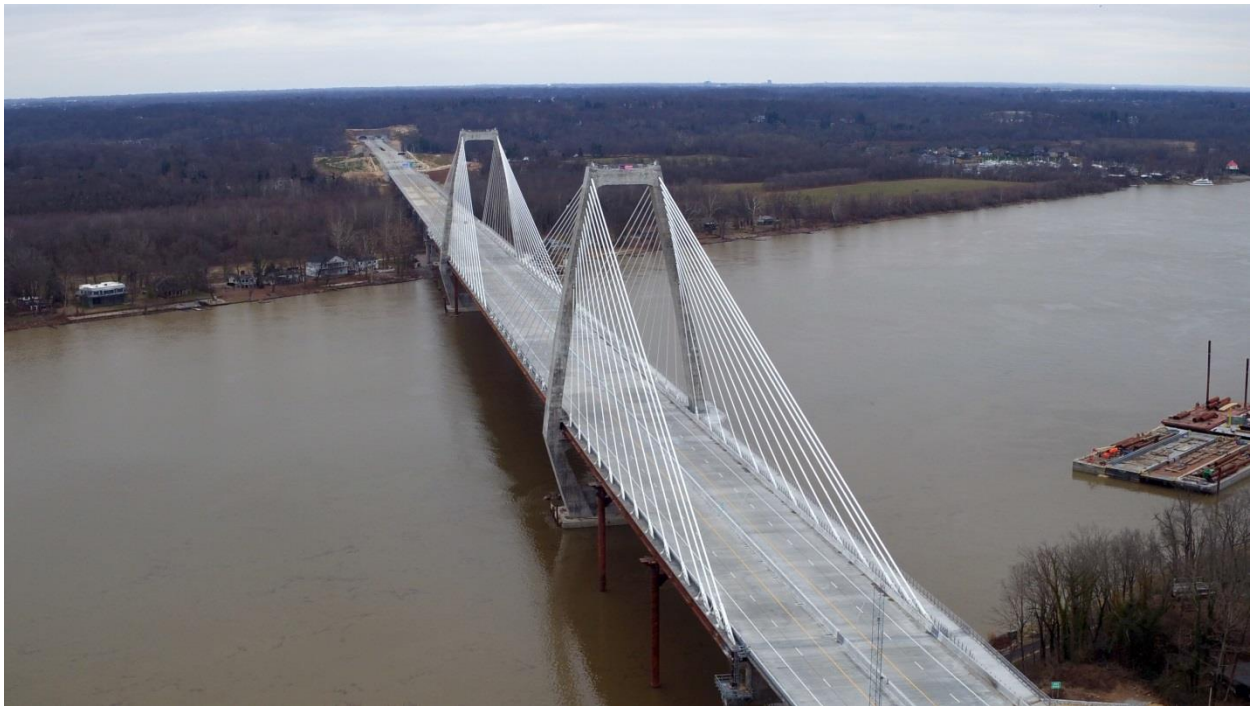
The Lewis and Clark Bridge spans the Ohio River and connects Indiana State Road 265 with Kentucky State Highway 841. (Photo courtesy of INDOT)
