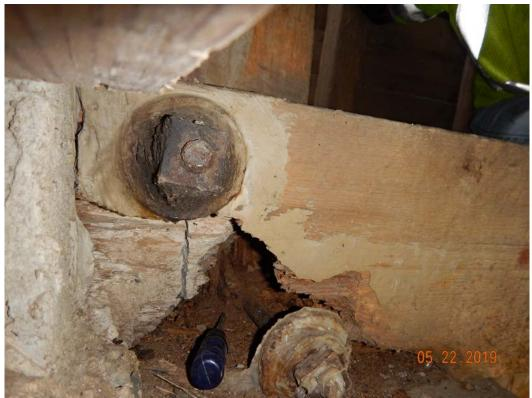
Photograph #14: Looking at severe rot on the lower chord.
