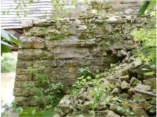
Photograph #18: Looking at deterorated stones in the northwest wingwall.
