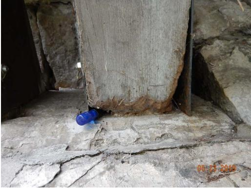
Photograph #15: Looking at severe rot to the lower chord at the bearing.
