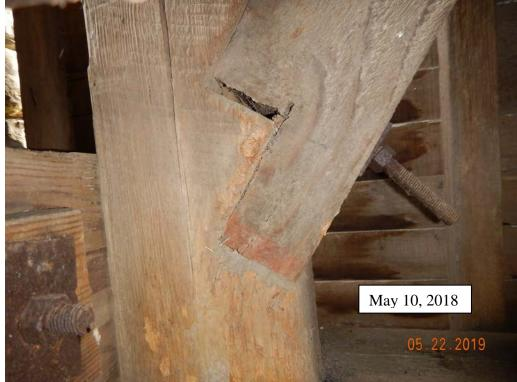
Photograph #11: Looking at the gap between the vertical and diagonal.
