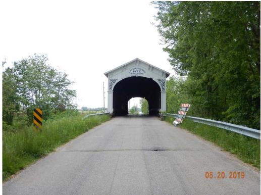
Photograph #19: Looking at approach guardrail to be replaced.
