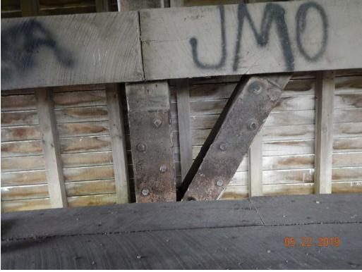
Photograph #9: Looking at existing plate repairs to the vertical and diagonal.
