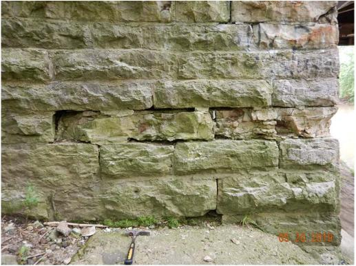
Photograph #16: Looking at stone deterioration at NE wingwall
