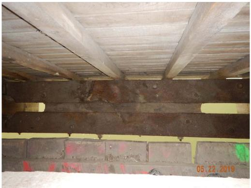
Photograph #10: Looking at existing steel plate repairs to the lower chord.
