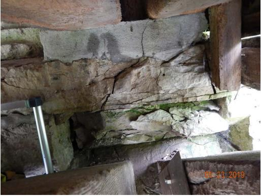
Photograph #17: Looking at cracked stone under northwest truss bearing.
