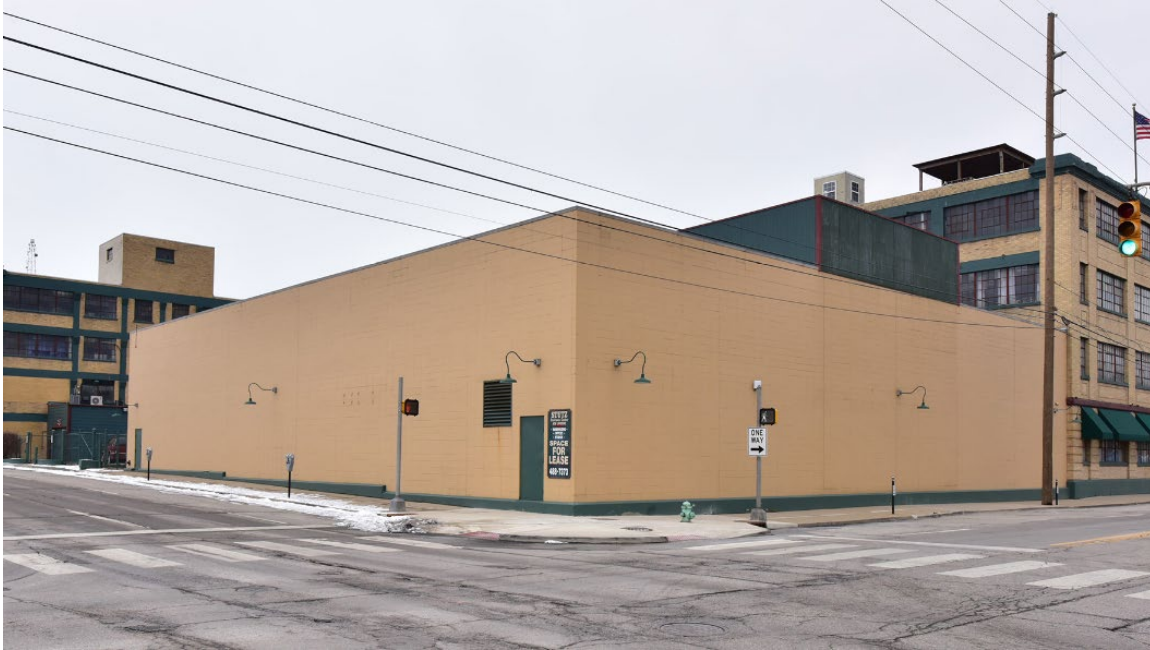
Figure 23. Building G. Top: North and west elevations, looking SE; bottom: interior, looking northwest from southeast corner. Source: Brad Finch, February 2021.
