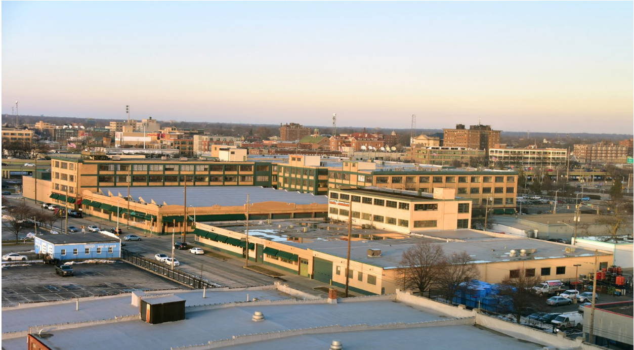
Figure 3: View looking northeast at the Stutz Factory. Source: Brad Finch, February 2021.
