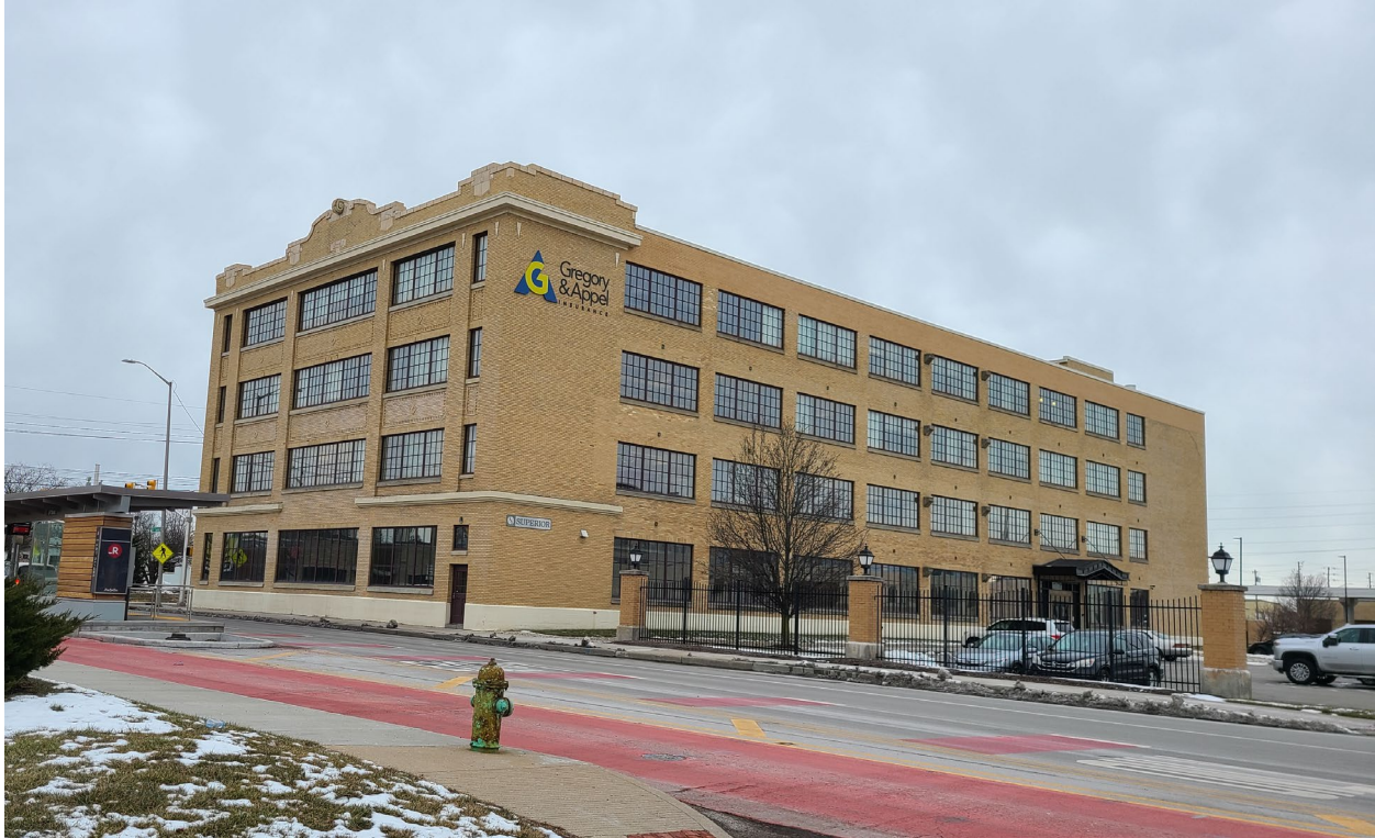
Figure 26. The H.C.S. Motor Car Company Building at 1402 North Capitol Avenue in February 2021, view looking southwest at east and north elevations. Source: Amanda Loughlin.
