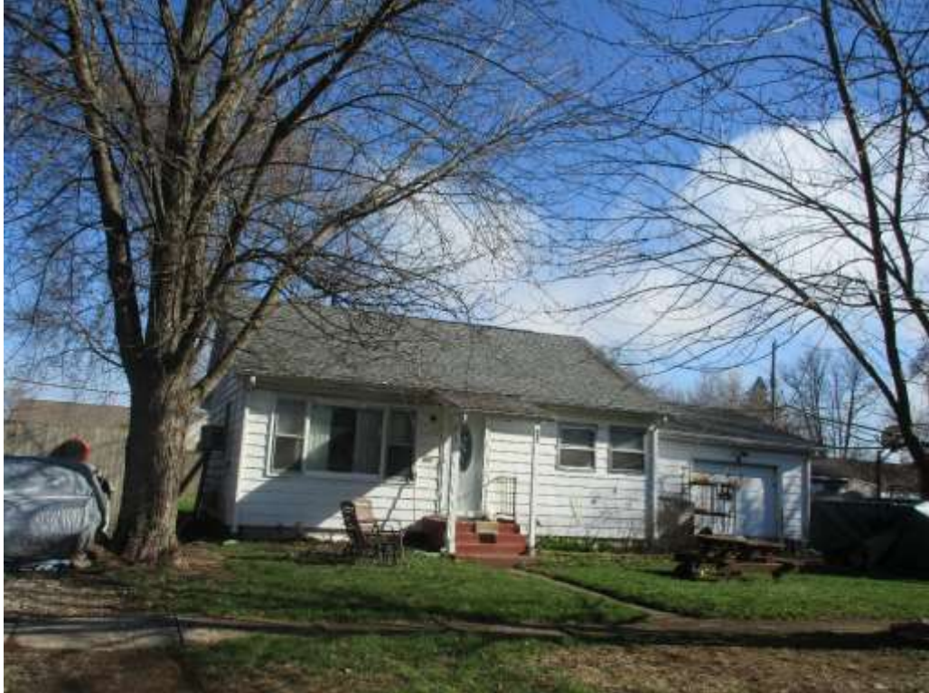
Photo 5: View of 452 Fairmount Road, facing north
