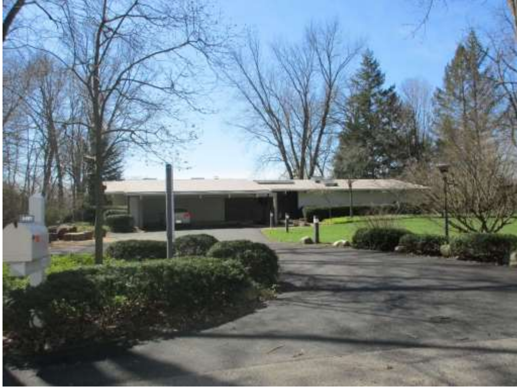
Photo 5: View of 311 Kenwood Place, facing south
