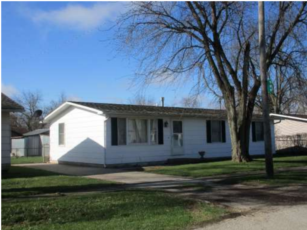
Photo 6: View of 509 Tudor Road, facing southwest
