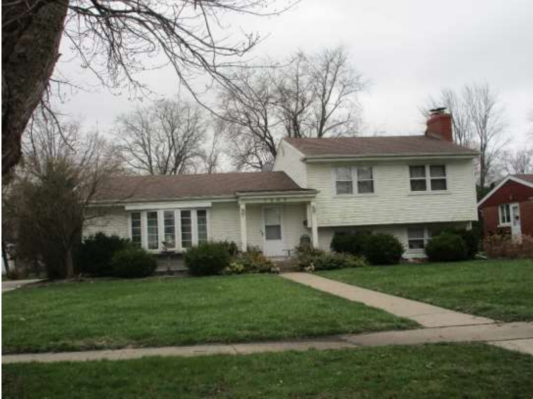
Photo 1: View of 1506 MacArthur Boulevard, facing south
