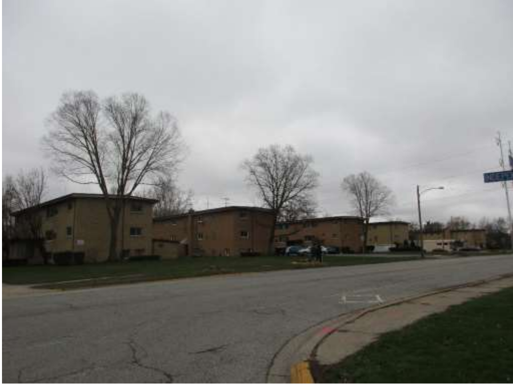
Photo 5: Streetscape view of White Oak Avenue, facing northwest
