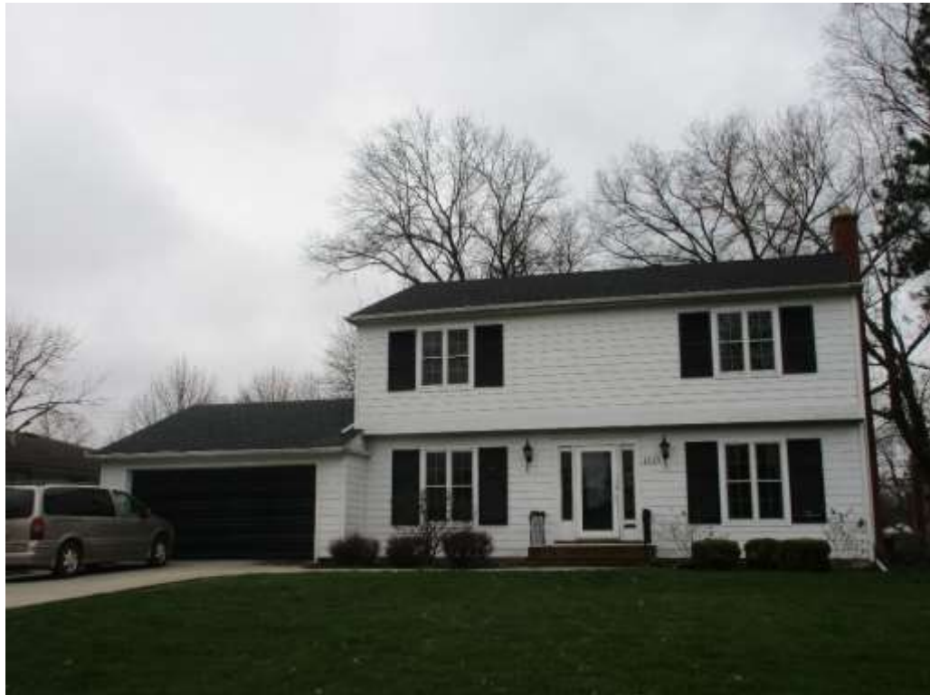
Photo 4: View of 1418 MacArthur Boulevard, facing south
