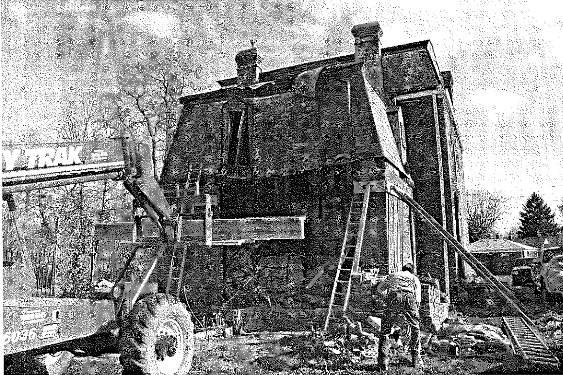
November 10, 2011 installation of support beam
