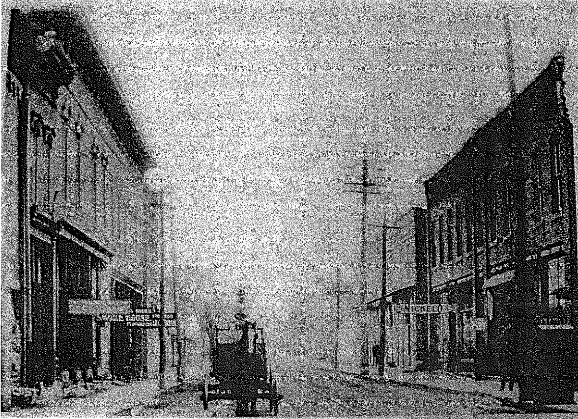
Photo D: 1. Locust Street west of Fifth Street. 2. Henry County, Indiana. 3. Unknown 4. c. 1905 5. Middletown Historical Society 6. North and south facades on Locust Street.
