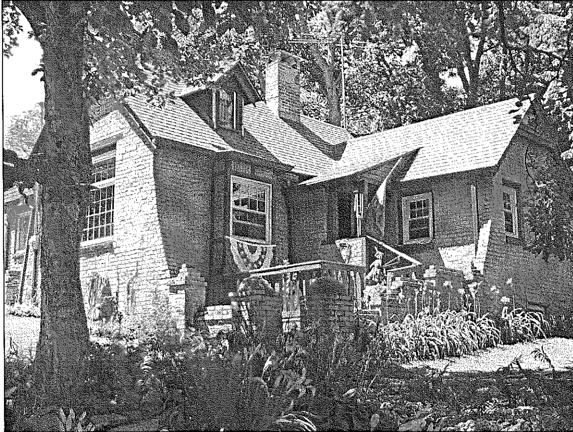
JC 9. 410 N. St. Clair St., c.1946. The house that Julian Cramer designed and built for himself features eccentric and whimsical elements, including brick courses "laid off the line," a door made from a cobbler's bench salvaged from the Old Hickory Furniture Co., a concrete relief image of his dog, Ruby, on the chimney face, hand-forged ironwork, and concretions used in the designed landscape. The house is an excellent example of folk art.
