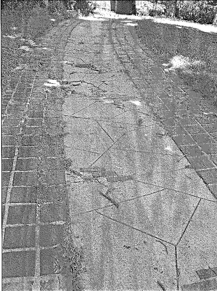
JC 5. 415 N. Jefferson St., 1928. This driveway features easily identifiable work by Julian Cramer and his brothers: incised concrete to resemble tiles and diamond brick insets framed by square brick pavers.
