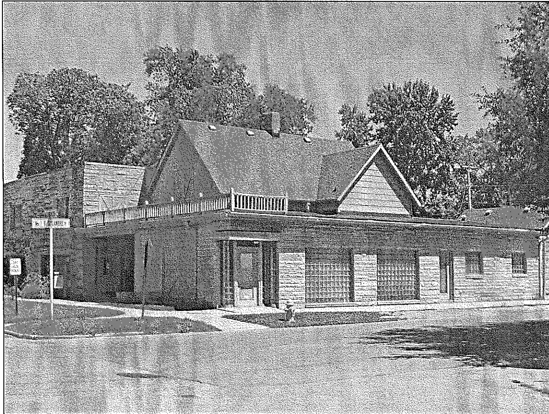
JC 10. 219 E. Washington St., c.1940. Julian combined several buildings for Dr. Wolf, an optometrist, by constructing a new commercial front made of limestone and glass block. The corner entrance features a floor of colored and incised concrete. The Washington Street entrance has a wall face of water struck Norman brick. Dr. Wolf was involved with the development of Lake Lemon in Monroe County. Julian built sea walls and buildings for him on the lake's north shore.
